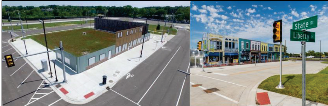
Figure 29. Mcity building facades provide an urban testing environment. The image on the left is a design rendering, and the physical implementation on site is shown on the right . (Image reproduced with permission from Mcity 2015.)
