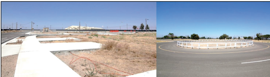
Figure 7. Castle features driveway infrastructure ( left ) and a roundabout feature ( right ) to further challenge vehicle competencies. (Images reproduced with permission from Madrigal 2017.)
