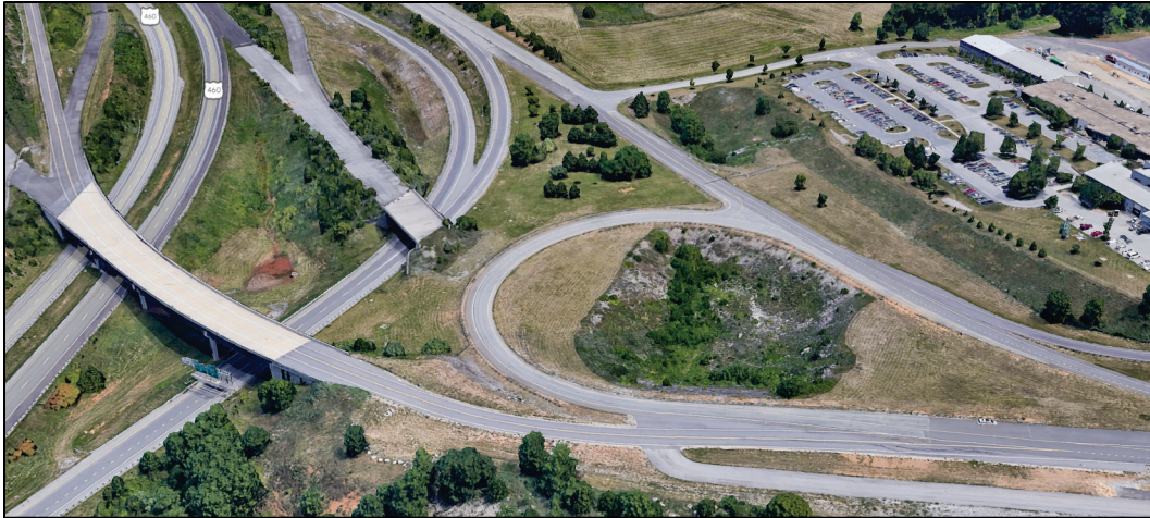
Figure 49. Satellite imagery of Virginia Tech Transportation Institute (VTI), where AVs can be properly challenged for real-world urban and suburban situations on the designated surface street. (Map data: Google Landsat / Copernicus 2019.)
