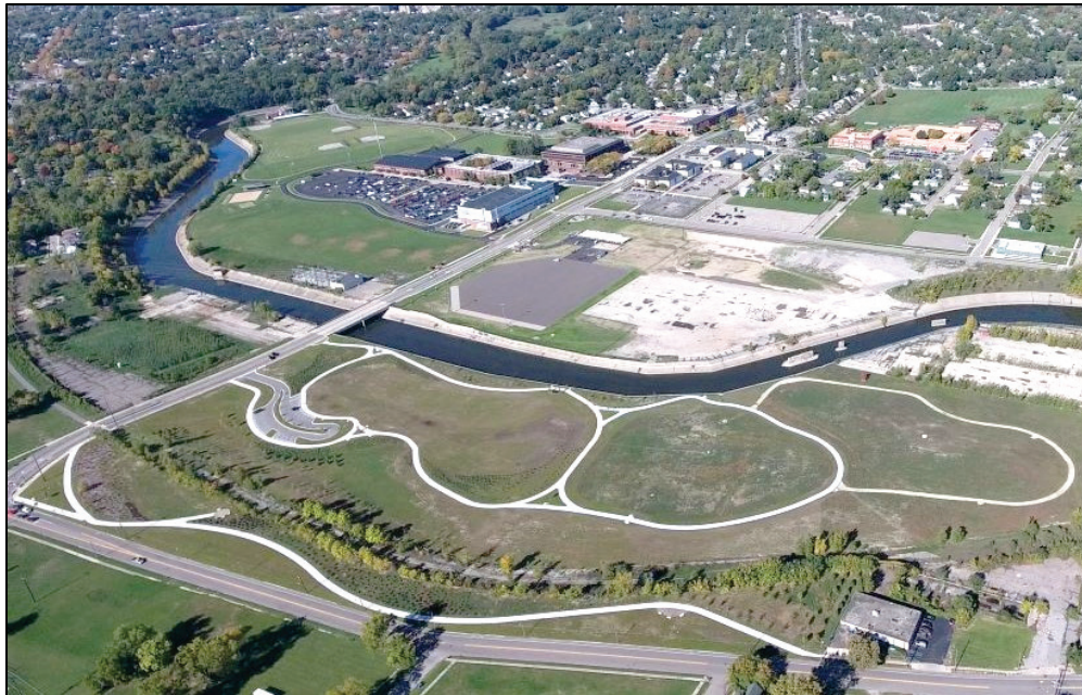
Figure 15. Satellite imagery of the General Motors (GM) Mobility Research Center, which features a unique road structure that allows for extensive testing capabilities. (Map data: Google Earth 2019.)
