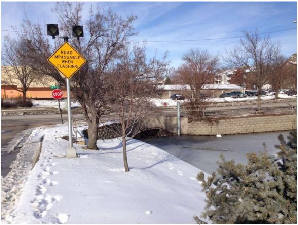
Figure 13. Stage Activated Traffic Flood Warning Device near 50th and R Streets, Lincoln, NE
