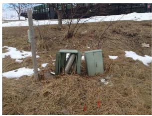
**Photo #7** Broken electrical/communications box near southeast corner of Home Depot.
