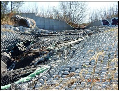
Figure 8. Eroded Tributary Outfall Between 38th St. and 48th St.
