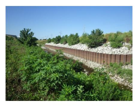
Figure 5. Bank stabilization (rock rip-rap) shown on the west bank. Standing on the east bank looking southwest.
