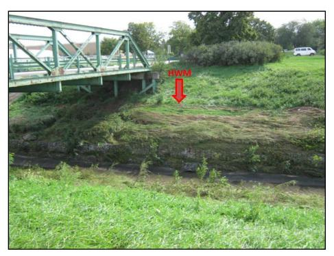
Figure 13. High water mark at 38th Street Bridge
