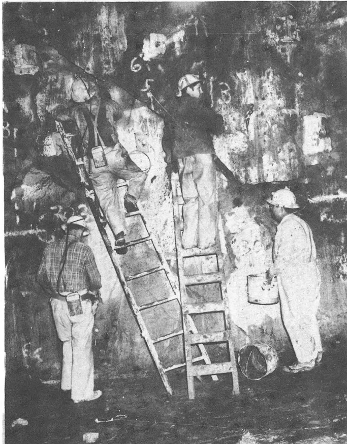
Calking Cracks
