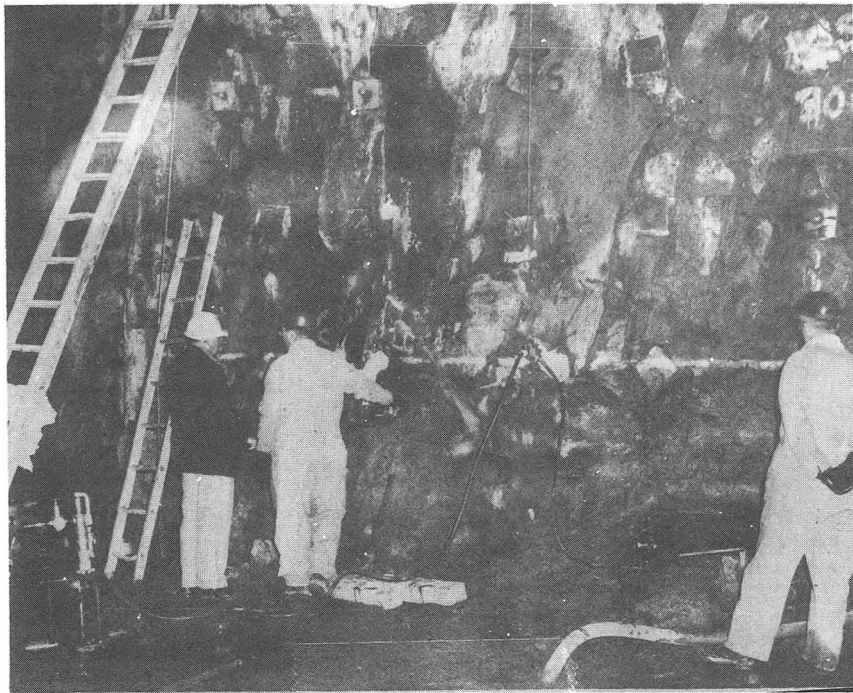
Epoxy Resin Injection Operations
