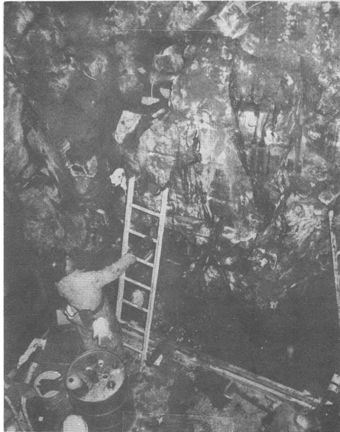
Polyester Resin Grout Returns During Injection of Hole T-8
