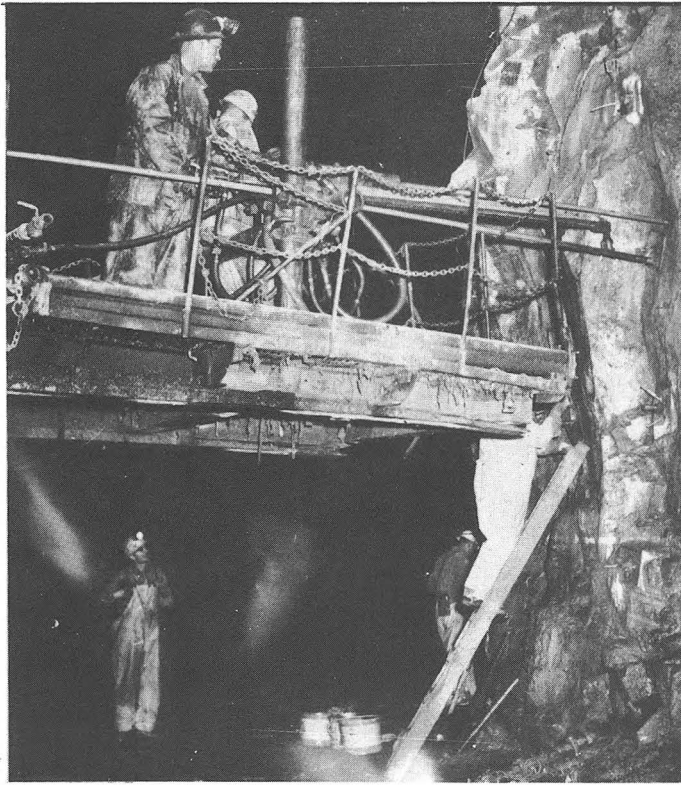
Drilling Injection Holes
