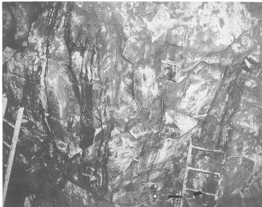
Polyester Resin Grout Returns During Injection of Hole T-8
