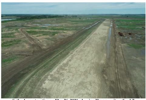
Setback construction on May 26, 2021, showing "borrow pit wetlands" on both sides of new levee alignment
