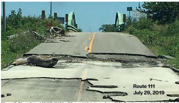
Figure 7. Photo from MDOT (2020) of Route 111 damage from 2019 flooding, east of the L-536 project area
