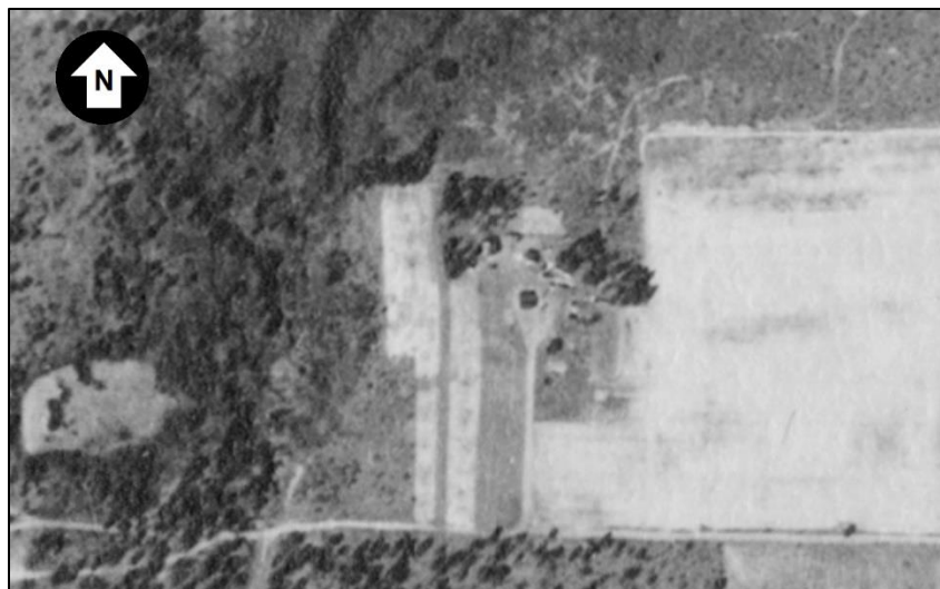
Figure 334. A 1939 aerial photograph of a farmstead associated with tract 328. (Image from Fort McCoy CRM. Public domain.)
