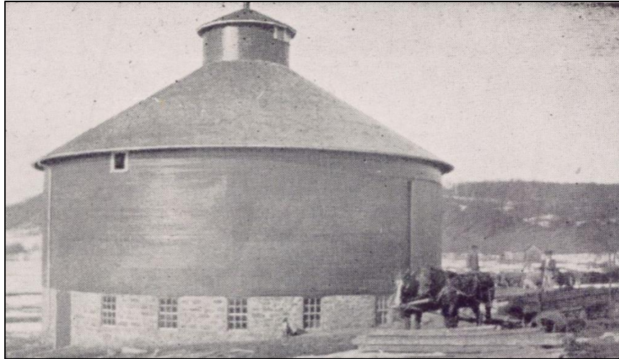
Figure 13. A 1915 image of a round barn with a central silo in Monroe County, on the Casper Heilmann farm. (Image from Wisconsin Historical Society. Public domain.) 74
