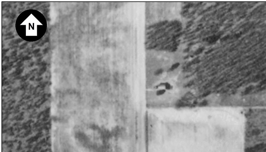
Figure 360. A 1939 aerial photograph of the schoolhouse on tract 353. (Image from Wisconsin Historic Aerial Imagery Finder. Public domain. Modified by ERDC-CERL, 2023.)
