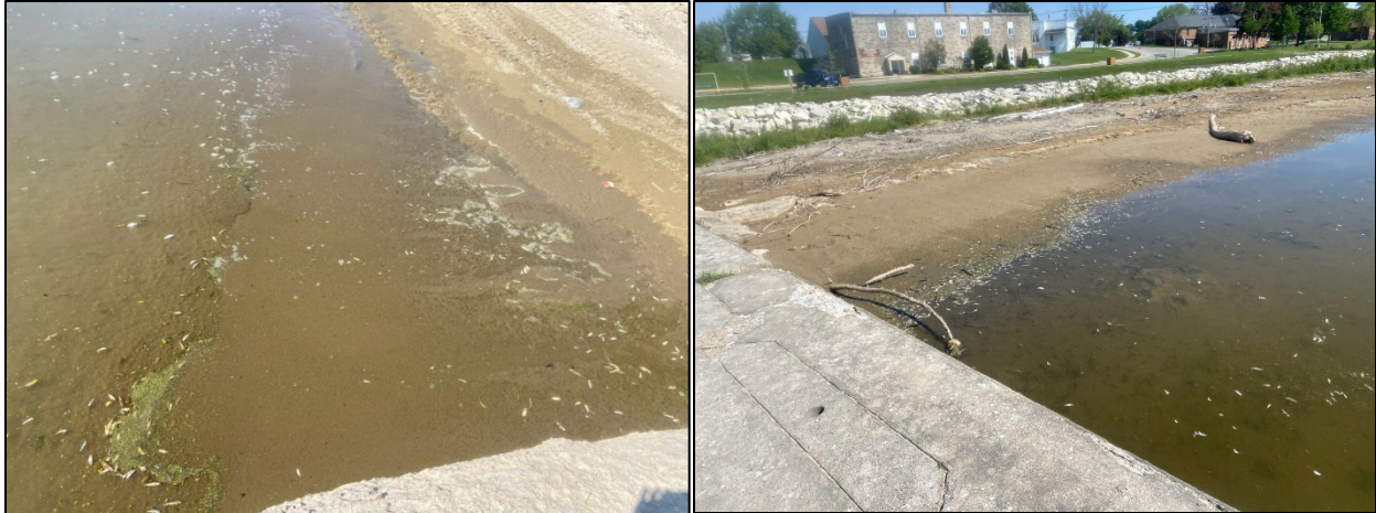
Photo 3: Evidence of collection of detritus as the point where the south breakwater meets the shore. Left - Lakeward side. Right - Harbor side. Photos taken July 2022.
