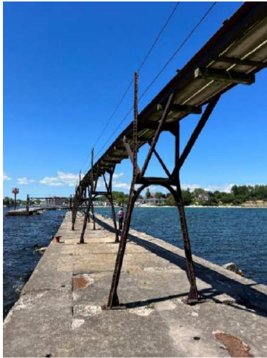
Photo 1 – Existing Catwalk Structure on the North Breakwater
