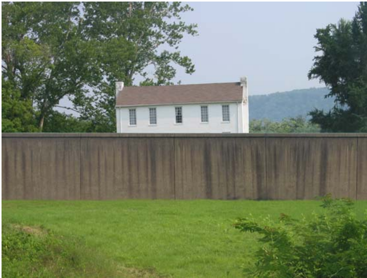
Figure B.1. Simulated floodwall surrounding the Jenkins House.
