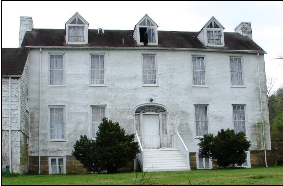
Figure 1. On the North elevation, the awkward placement of dormers disrupts the alignment of the Federal window program below (author).
