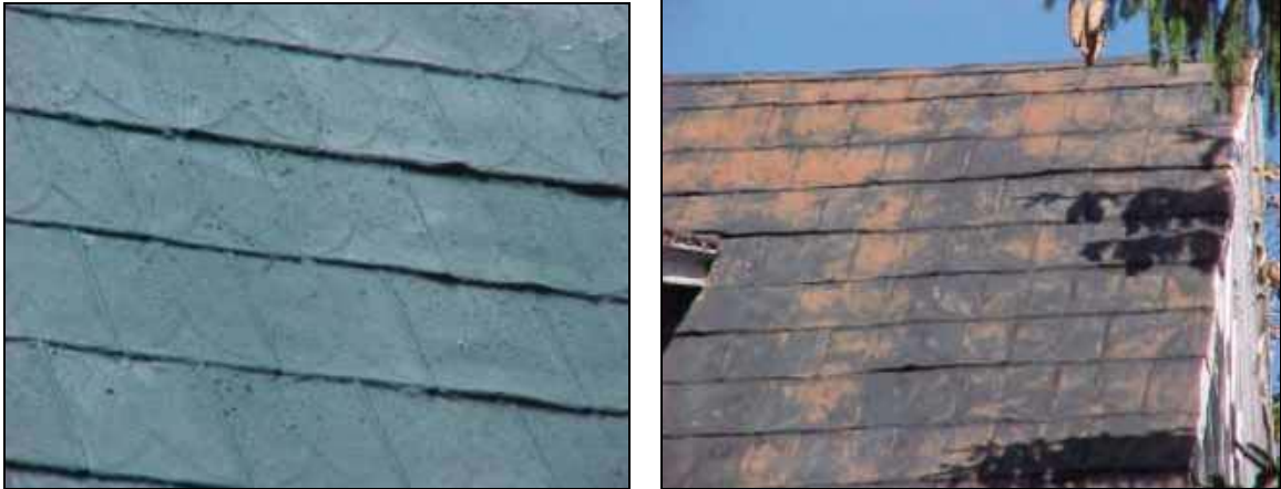
Figure 3. Two examples of late nineteenth century textured tin shingles found on Virginia houses. The circa 1906 photo of the Jenkins House (below) depicts a replacement roof with a similar use of metal shingles, applied as flat sheets stiffened at ridges with a protective material.
