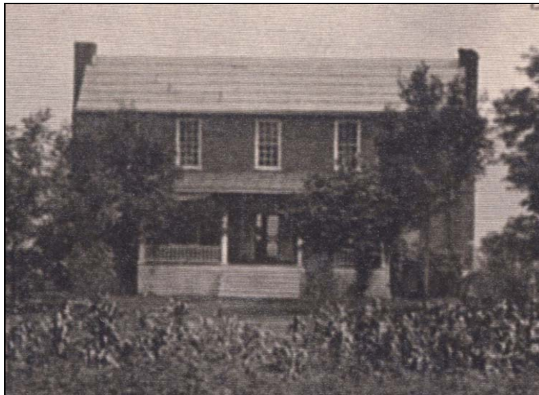
Figure 4. The only photograph currently available that reveals the status of the roof during the home's brief occupation by the F. A. McDonald family between 1905 and 1906. The dormers had not yet been installed. Although the image depicts six rows of roofing material with some texture, it is not clear whether this cladding was wood shingle, wood board, or metal, however the evenness of the horizontal lines and the wide vertical size of the rows suggest metal.
