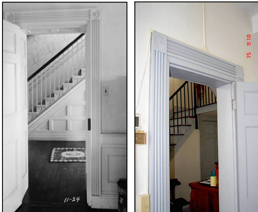
Figure 12. At left, a well preserved interior door frame from Dan's Hill, Virginia, reveals that the west room entry details at the Jenkins House are faithful to the Federal design period, and can serve as an original template for the restoration of interior finish details, when needed. (author)
