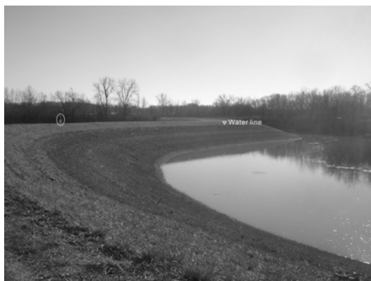
Figure 5. The Valley Park levee looking south, only 1 hour after the flood gates were reopened on January 2, 2016. The floodwater level (dark) almost breached the levee and exceeded the estimated level for a “100-year flood” (FEMA, 1995) by nearly 2 m, forcing evacuation of the protected area to the left. Bicyclist (circled) on levee top shows scale. Photo by Robert E. Criss.
