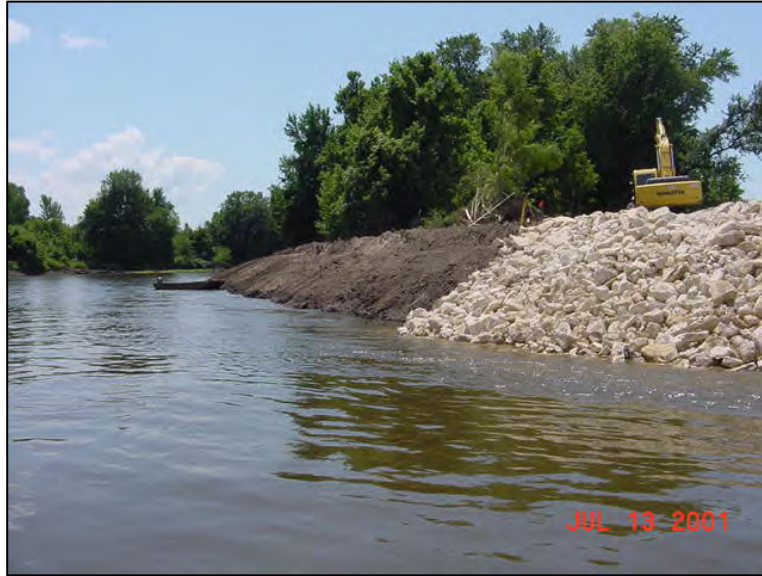
Photograph M-10: Rock Placement Following Shaping (Gardner Division HREP)
