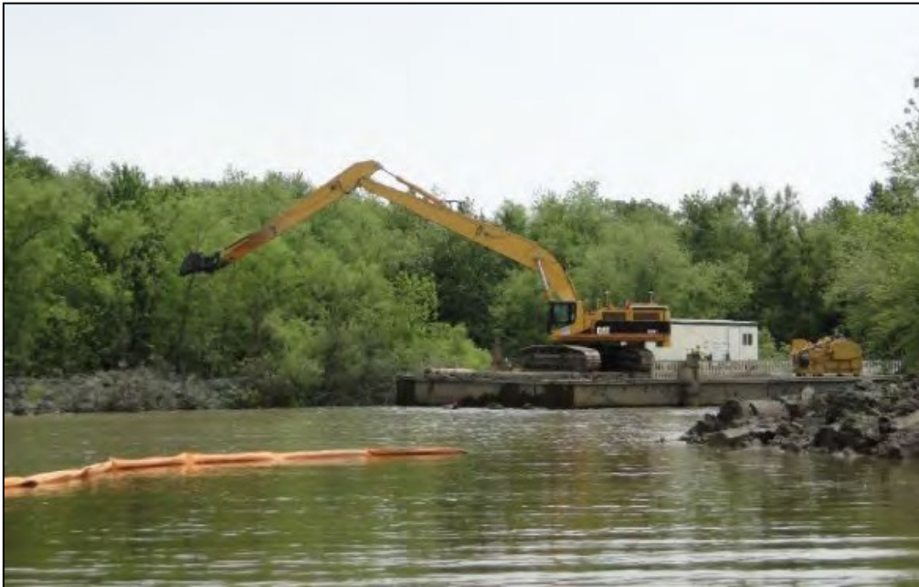
Photograph M-2: Barge-mounted Excavator (Lake Odessa HREP)
