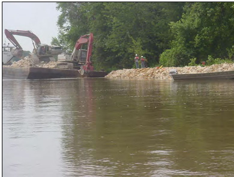
Photograph M-11: Transporting Rock from Barge to Bankline (Gardner Division HREP)
