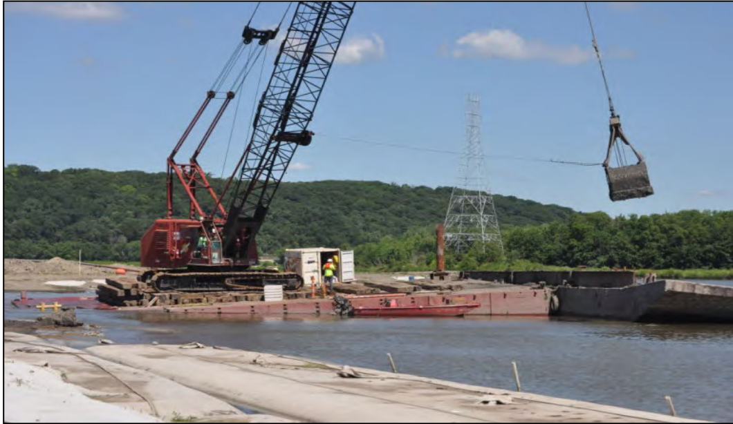
Photograph M-3: Barge-mounted Crane with Clamshell Bucket (Peoria Islands)
