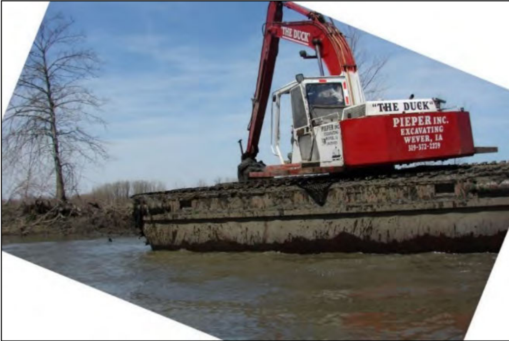
Photograph M-1: High Buoyancy Excavator (Lake Odessa HREP)
