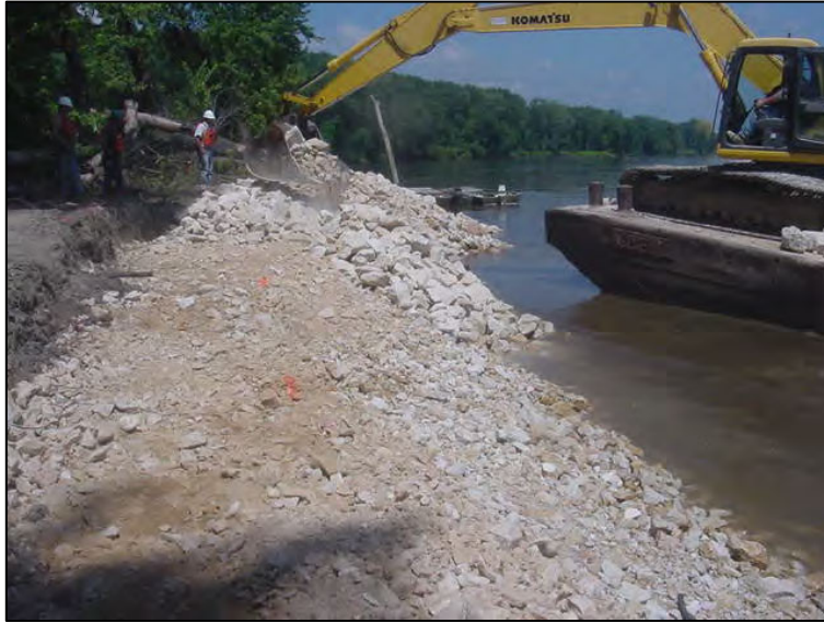
Photograph M-12: Riprap on Bedding Stone (Gardner Division HREP)
