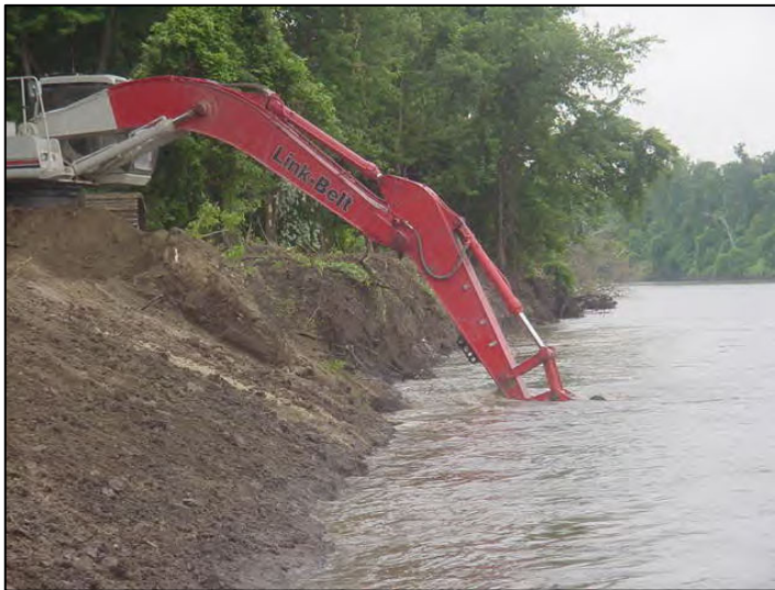
Photograph M-8: Bankline Shaping Prior to Receiving Rock Protection (Gardner Division HREP)
