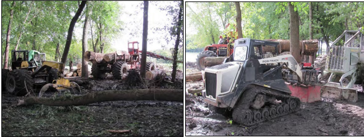
Photograph M-5: Tree Clearing Equipment (Huron Island HREP)
