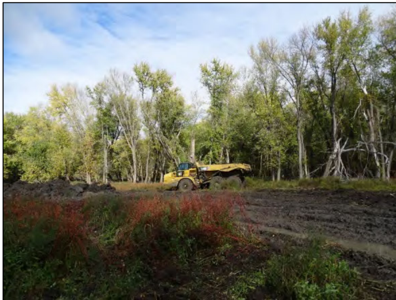
Photograph M-6: Transporting Excavated Material from Adjacent Placement Site to Forest Enhancement Site (Huron Island HREP)
