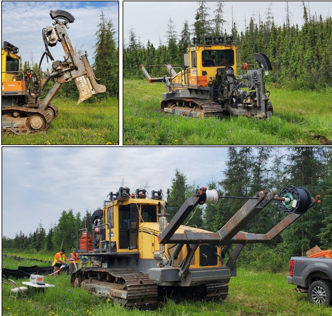
Figure 10. Fiber optic installation with a cable plow.
