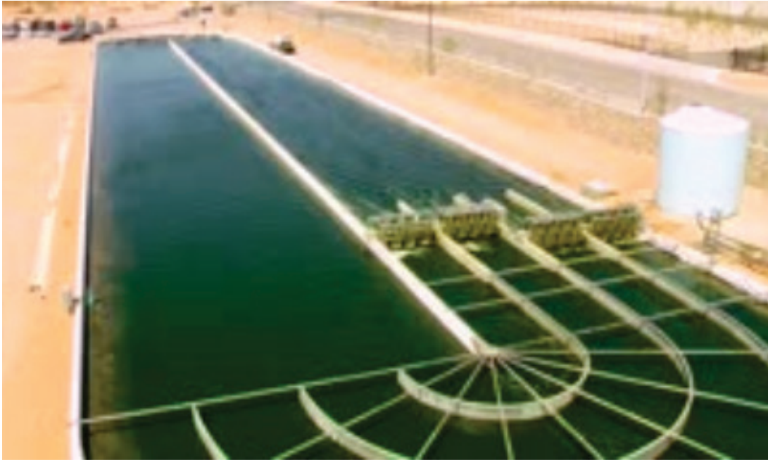
Figure 2. Sapphire Energy raceway pond.
