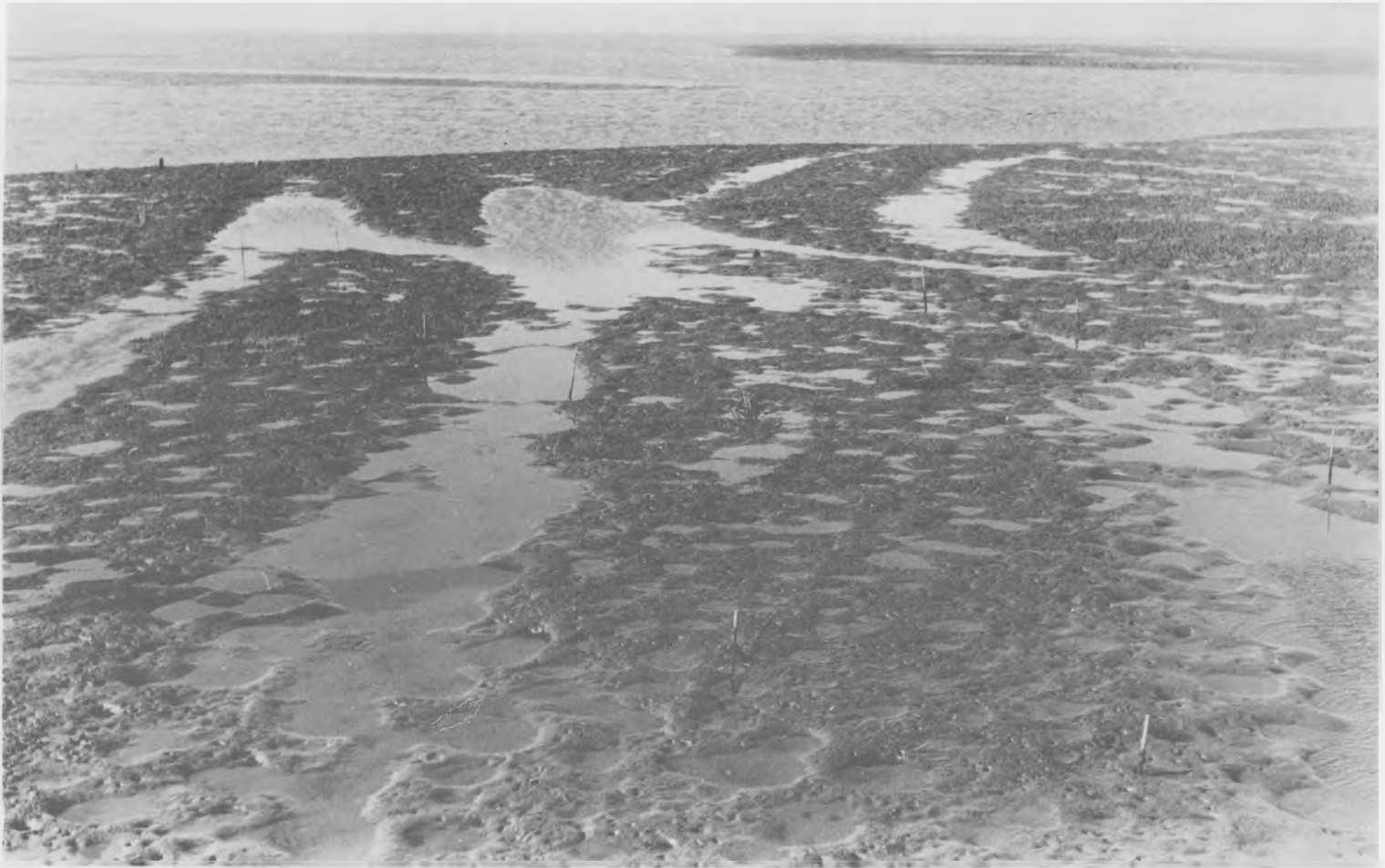
Figure 11. Bulldozer tracks made during construction of the marsh area in 1975 still evident at low elevation in October 1977
