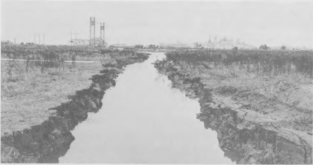
a. Interior trench constructed in an approximately 10-in. surface crust
