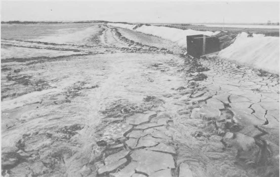
Figure 16. Collector sump walled in front of outflow weir by pivoting the RUC in place several times
