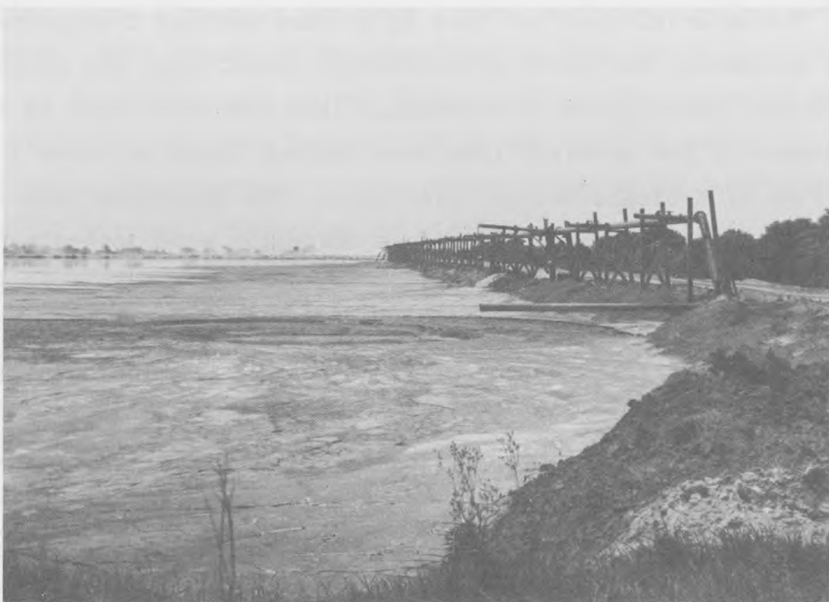
b. Deposition of coarse-grained material adjacent to perimeter dike to facilitate future dike raising
