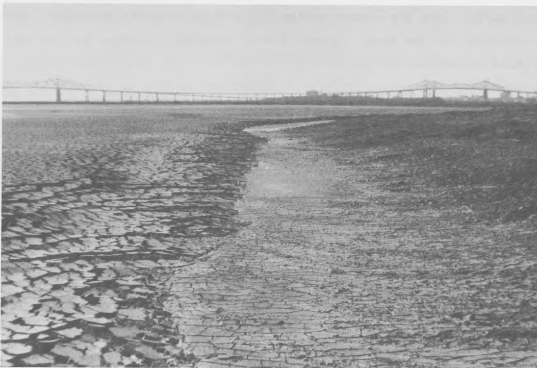
Figure 5. Shallow initial perimeter trench constructed by dragline operating from perimeter dike
