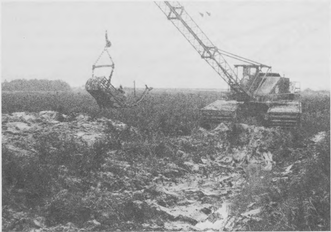
Figure 33. Amphibious dragline constructing initial drainage trenches in 6-in. surface desiccation crust
