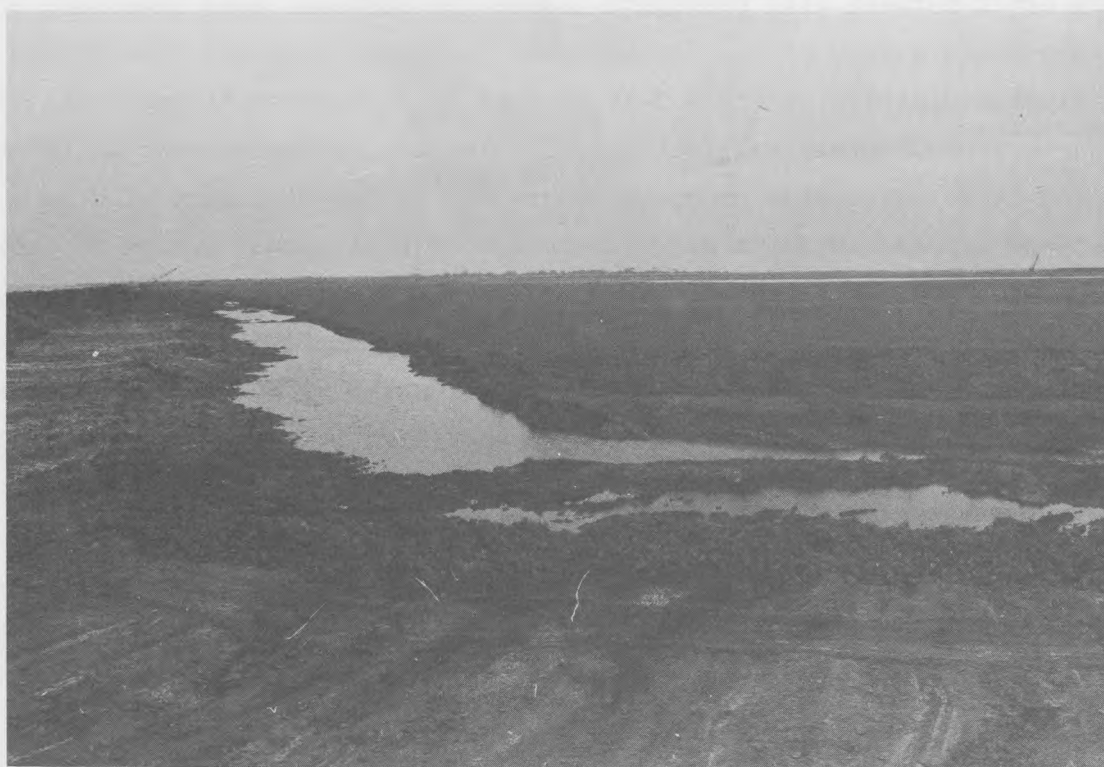
Figure 10. A well-developed perimeter trenching system
