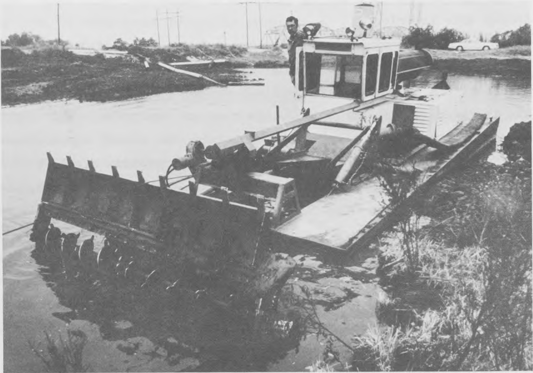
Figure 28. Mudcat dredge used in disposal site interior trenching operations
