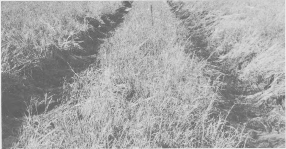
a. Incomplete RUC trench produced on initial trenching pass
