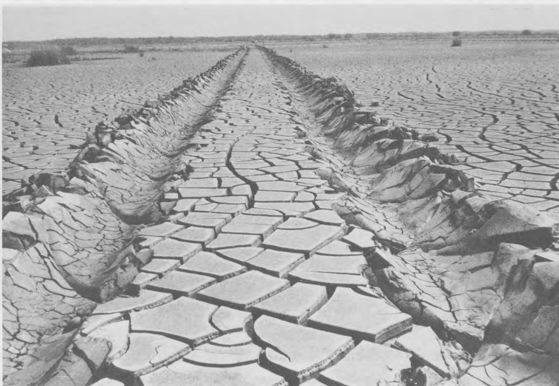
Figure 19. Dredged material surface drying and crust formation produces a crack network draining directly into the RUC drainage trenches
