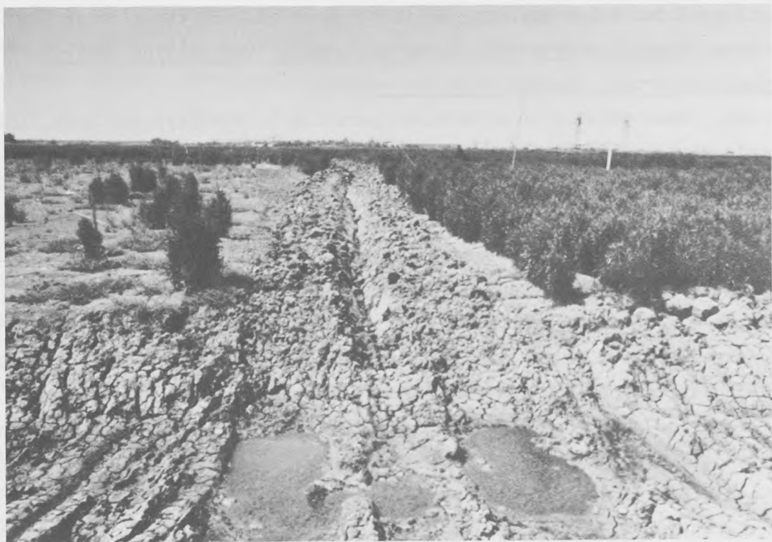
Figure 27. Thiokol drag plow produced trenches extending from the dragline perimeter trench into the disposal site
