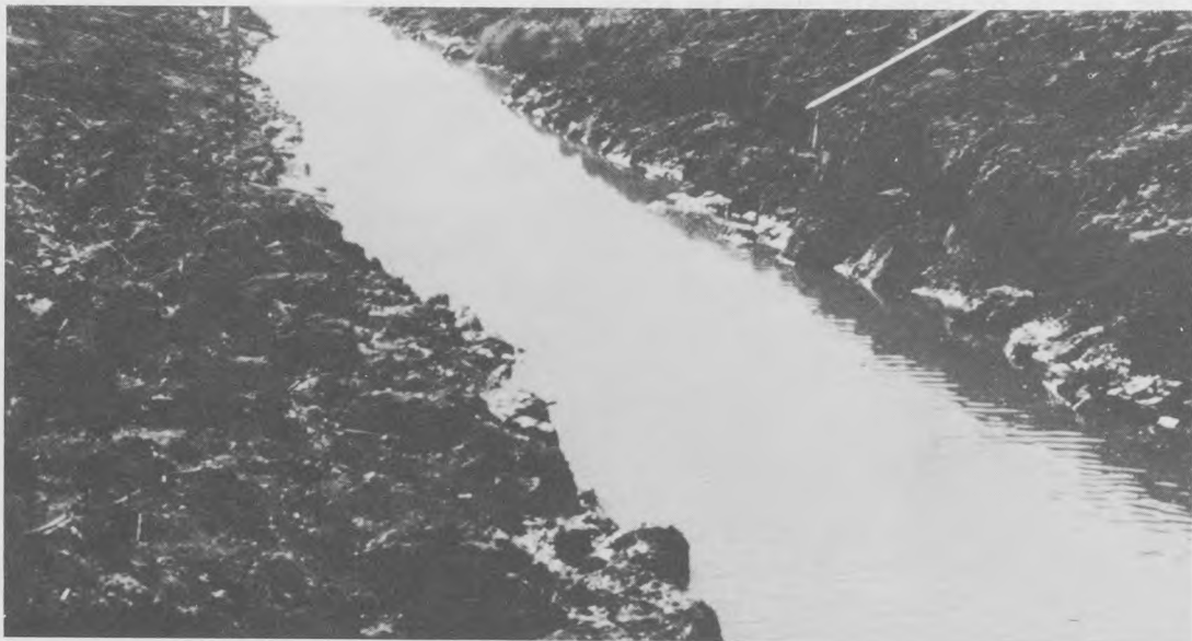
b. Deepened perimeter trench between outlet weirs, originally made by dragline
