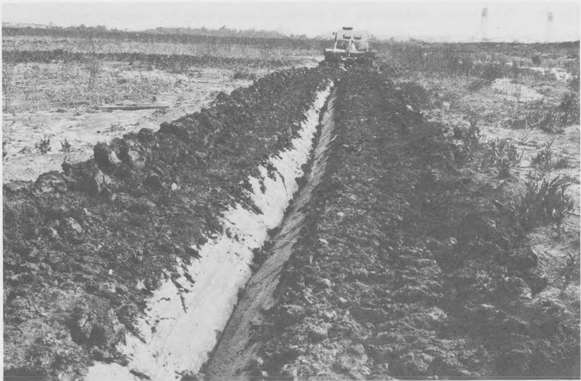
Figure 26. Trackmaster and drag plow trenching operation in progress
