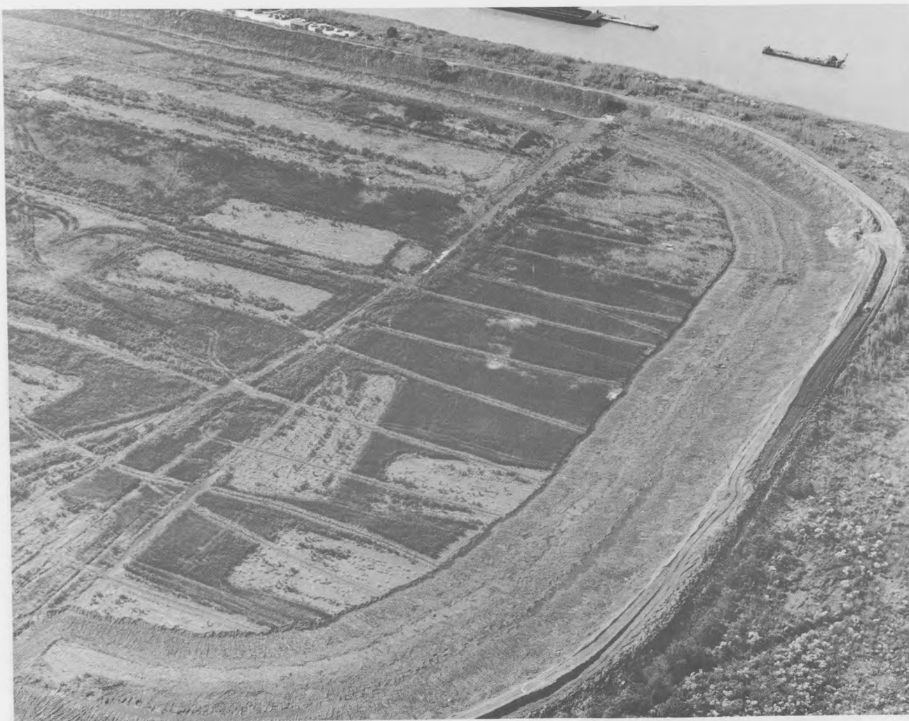
Figure 7. Aerial view of north end of Upper Polecat Bay Disposal Area, looking west southwest from northeast corner. Note strip of dewatered fine-grained dredged material removed around disposal site perimeter
