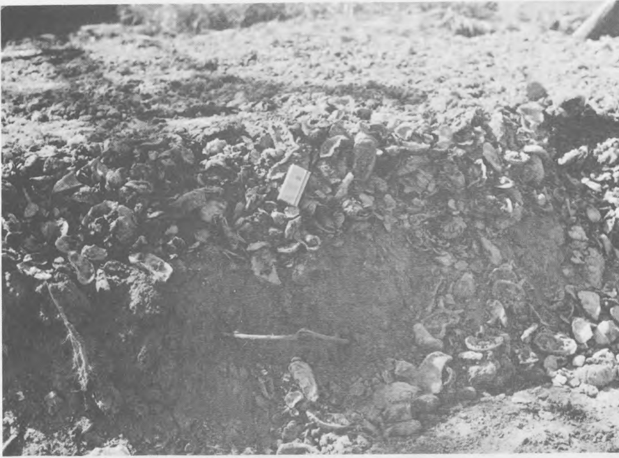
Figure 9. Photograph of completed haul road section showing dredged material surface, semicompacted subgrade mound, and shell surfacing. The fabric was placed at the interface between surfacing and subgrade
