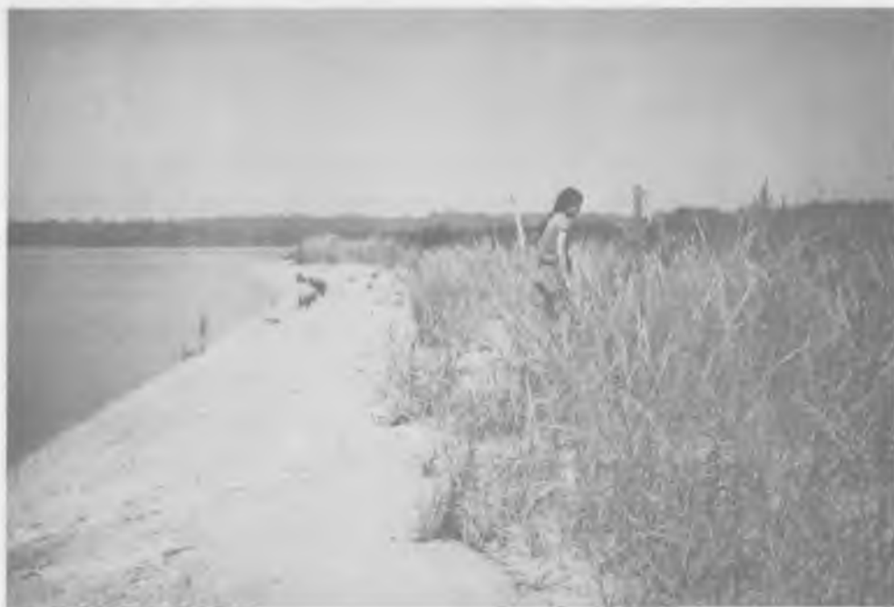
b. EXTERIOR SLOPES, SEP 1976
