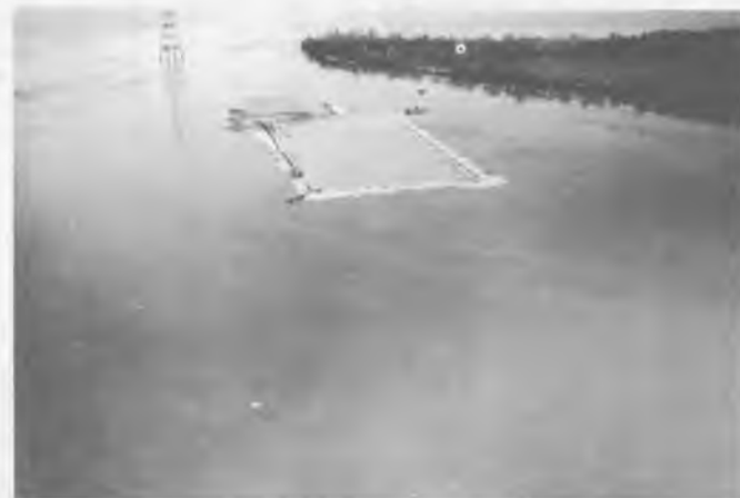
d. COMPLETED HYDRAULIC FILL, 17 JAN 1975
