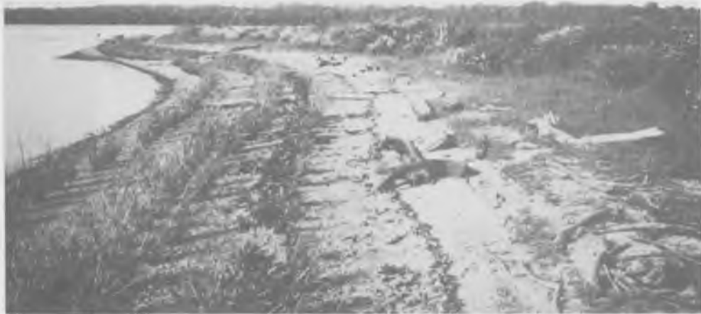
a. EXTERIOR SLOPE, OCT 1975
