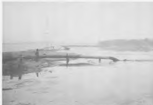
b. DREDGED MATERIAL DISCHARGE
