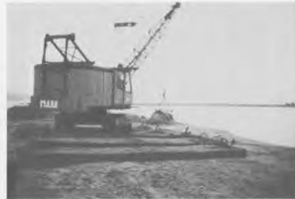
b. DRAGLINE FILL CONSTRUCTION
