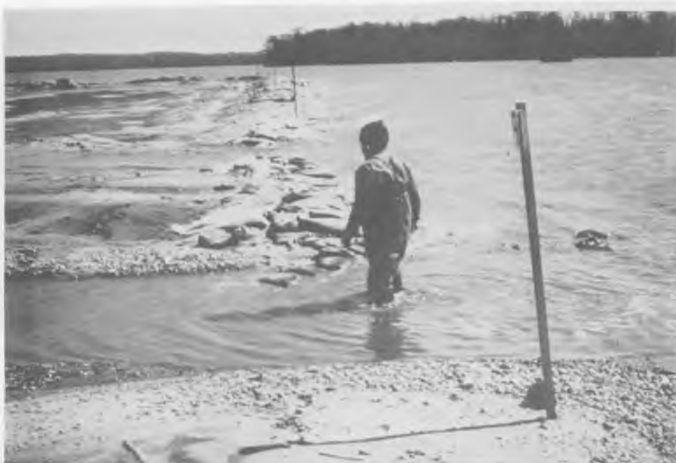
Figure 13. Breached section along south dike, 25 Mar 1975
