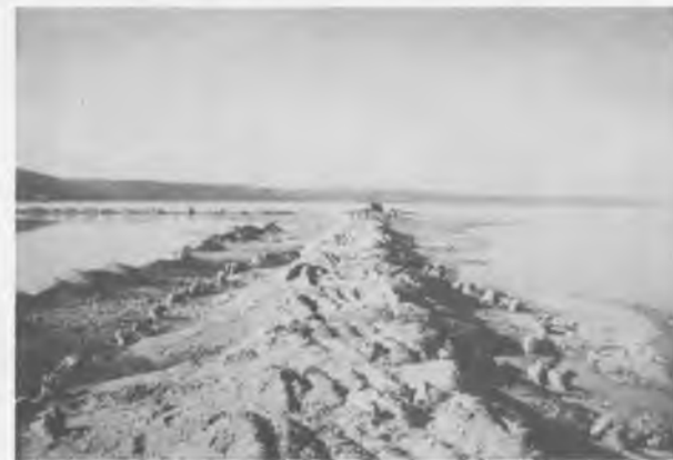
c. COMPLETED DRAGLINE FILL ALONG NORTH DIKE ALIGNMENT
