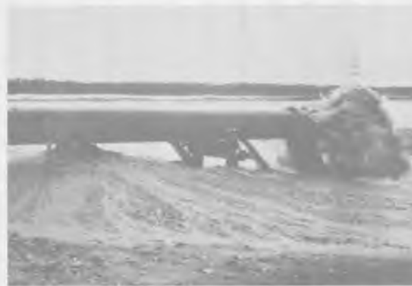
d. REPAIR OF BREACH ON SOUTH DIKE ALIGNMENT, 26 JAN 1975
