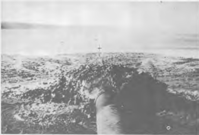
b. HYDRAULIC FILL CONSTRUCTION, 15 DEC 1974
