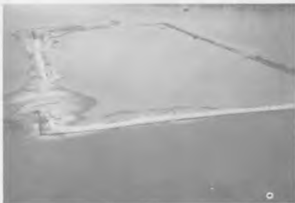
b. REPAIRED BREACH ON NORTH DIKE ALIGNMENT, 24 JAN 1975
