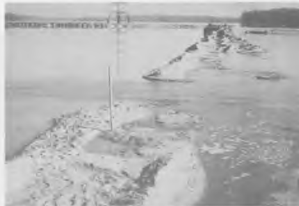
c. BREACH ON SOUTH DIKE ALIGNMENT, 24 JAN 1975
