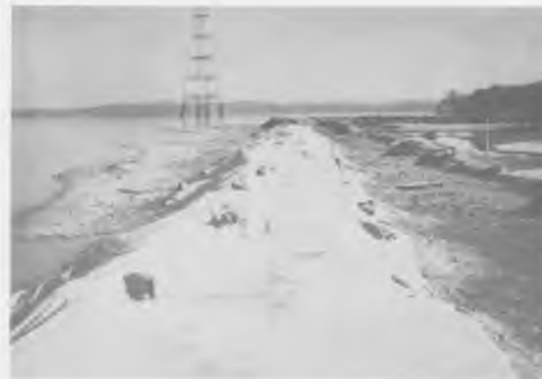
b. POLYETHYLENE SHEETING - NORTH DIKE ALIGNMENT, 23 JAN 1975
