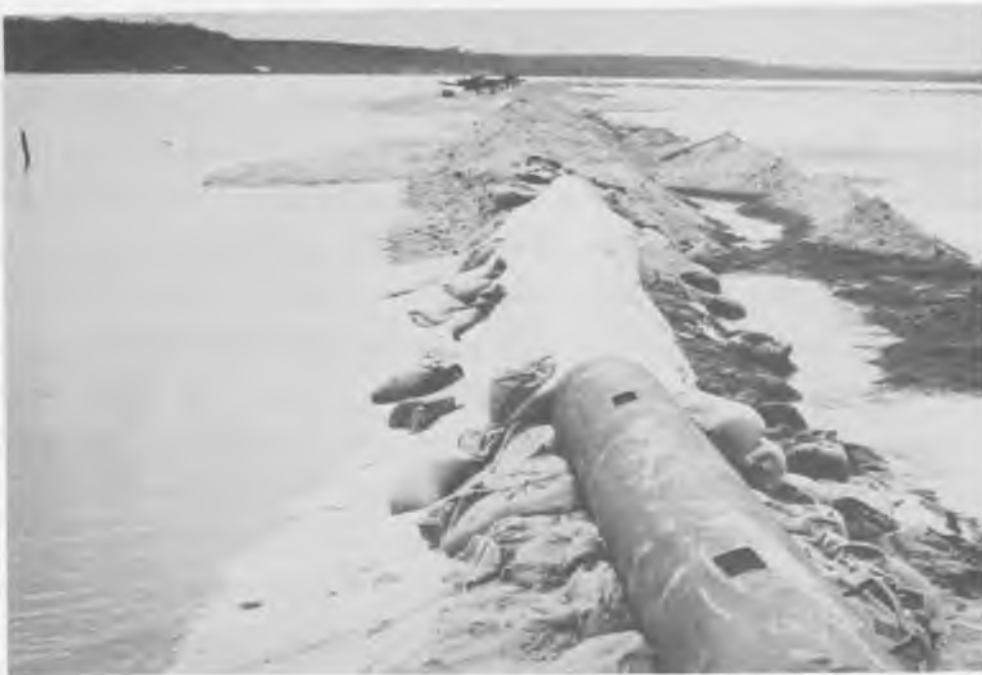
b. REPAIRED BREACH, 29 JAN 1975
