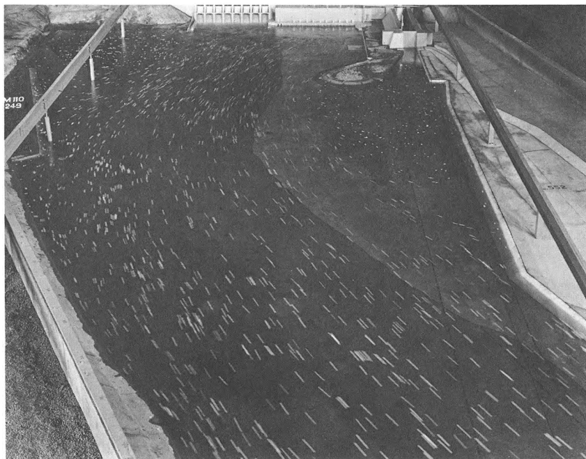
Powerhouse units 1 to 6 in operation
