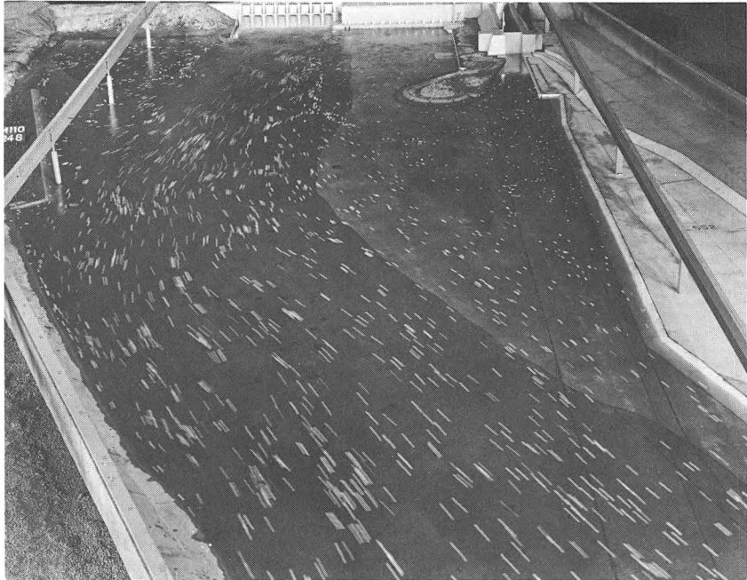
Powerhouse units 1 to 3 in operation
