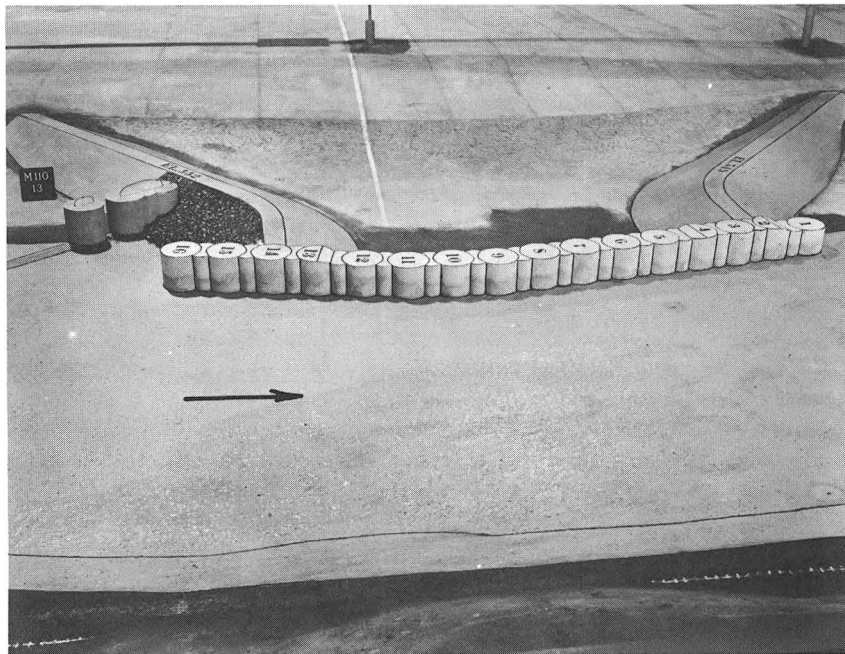
Fig. 3. Plan A (original design) first-step cofferdam and diversion channel. The cells upstream from cell 16 were not part of this plan.
