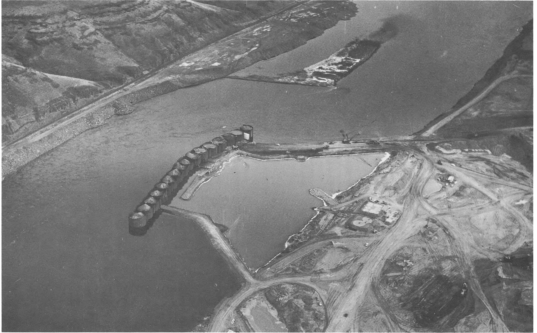
Fig. 4. Aerial view, looking upstream, of prototype first-step cofferdam.
