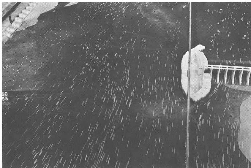
Stage I A: Cofferdam cells 1 to 3 removed with first-step embankments
