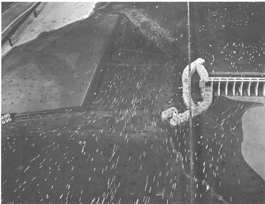
Stage III: Junior cofferdam along left bank
