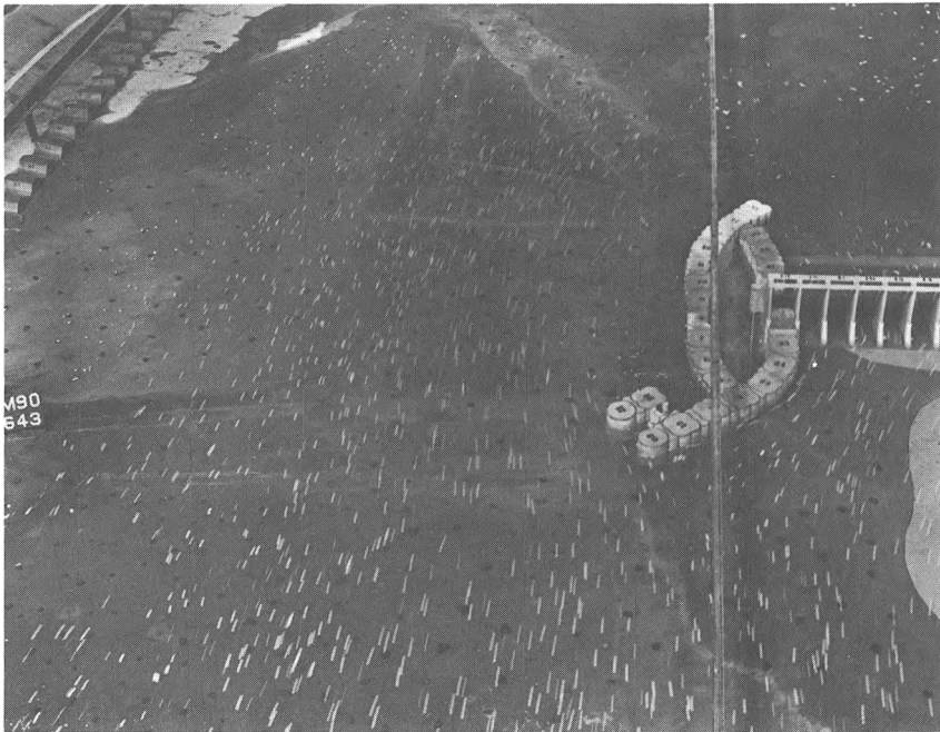
Stage II: Second-step cells 17 to 22 completed
