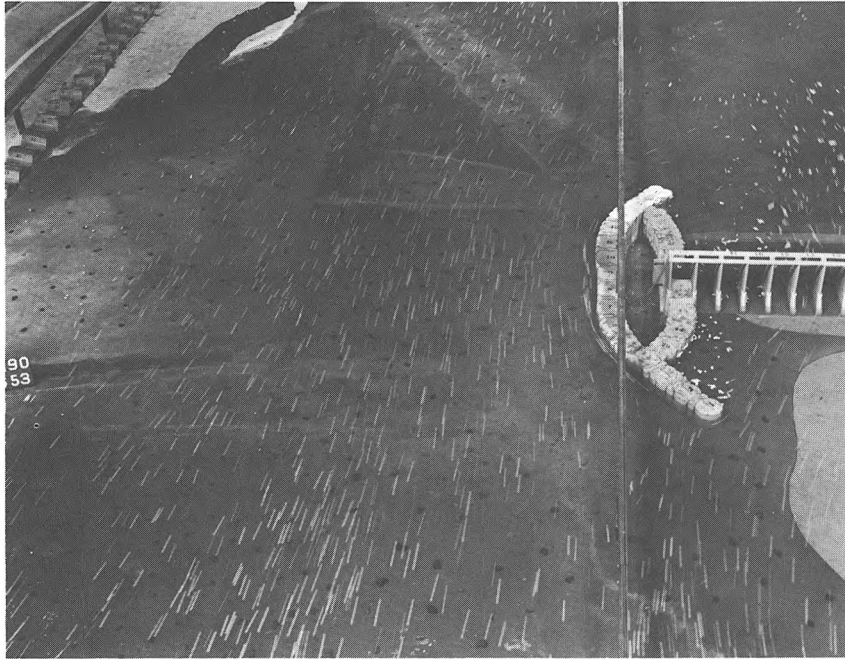
Stage I: Cofferdam cells 1 to 3 left after removal of first-step embankments
