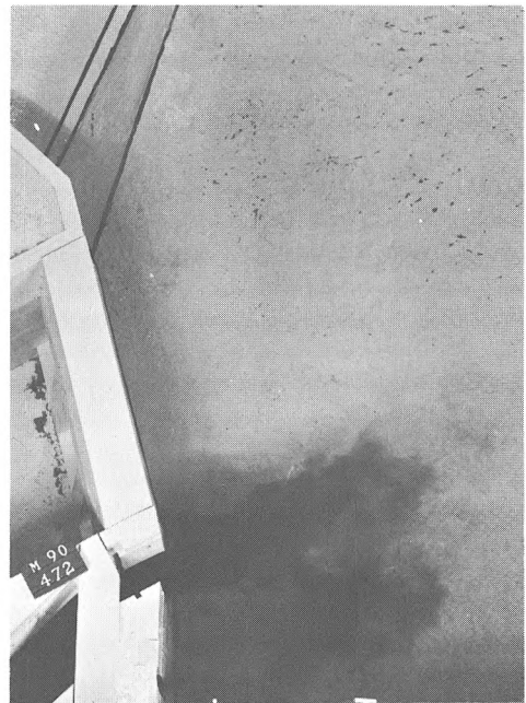
Powerhouse units 3 to 10 operated
