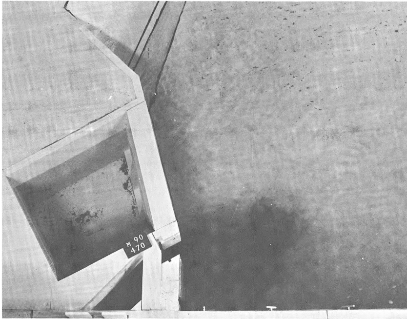
Powerhouse units 1 to 8 operated
