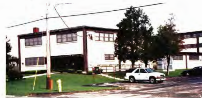
Building 2382 - south elevation with new glass entry
