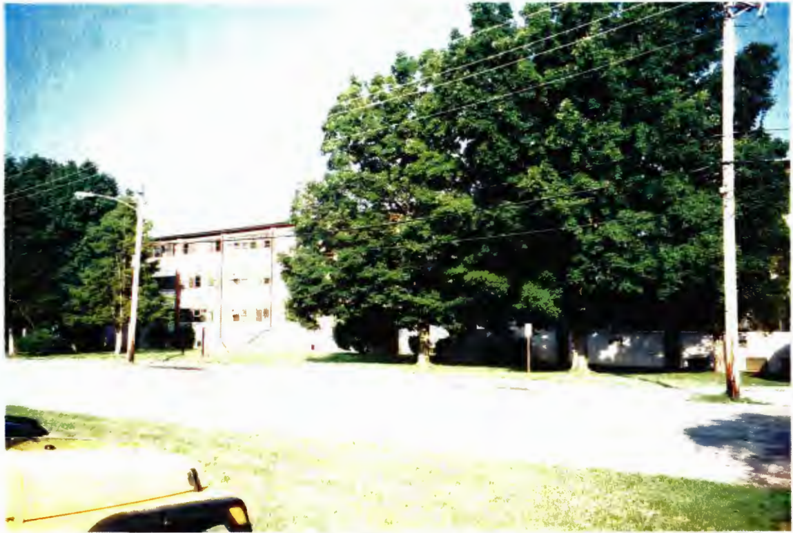
Building 297 – southeast elevation of the handle
