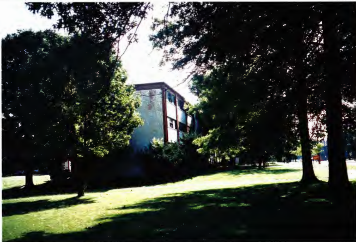
Building 1480 – west elevation of the handle
