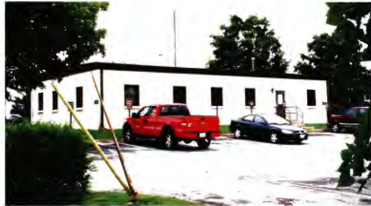
Building 6538 - oblique view of the north and east elevations
