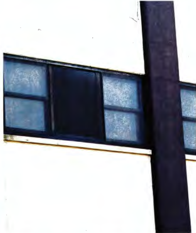
Current painted concrete and concrete block with anodized aluminum replacement windows
