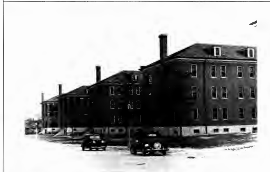
Figure 20: Permanent brick barracks constructed in 1934 to house four companies (Images of America: The United States Army at Fort Knox).
