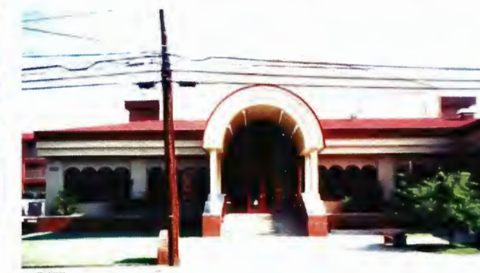
Building 1485 - new arched entrance, arched windows, and gable parapet wall located on the south elevation
