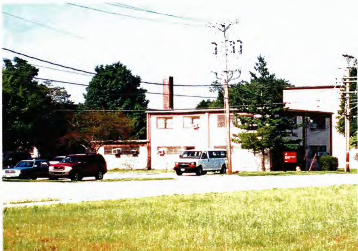
Building 1477 – north elevation
