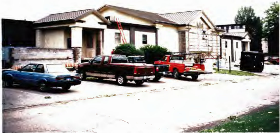
Building 6542 on the far right with an addition connecting to Building 6543 on the far left
