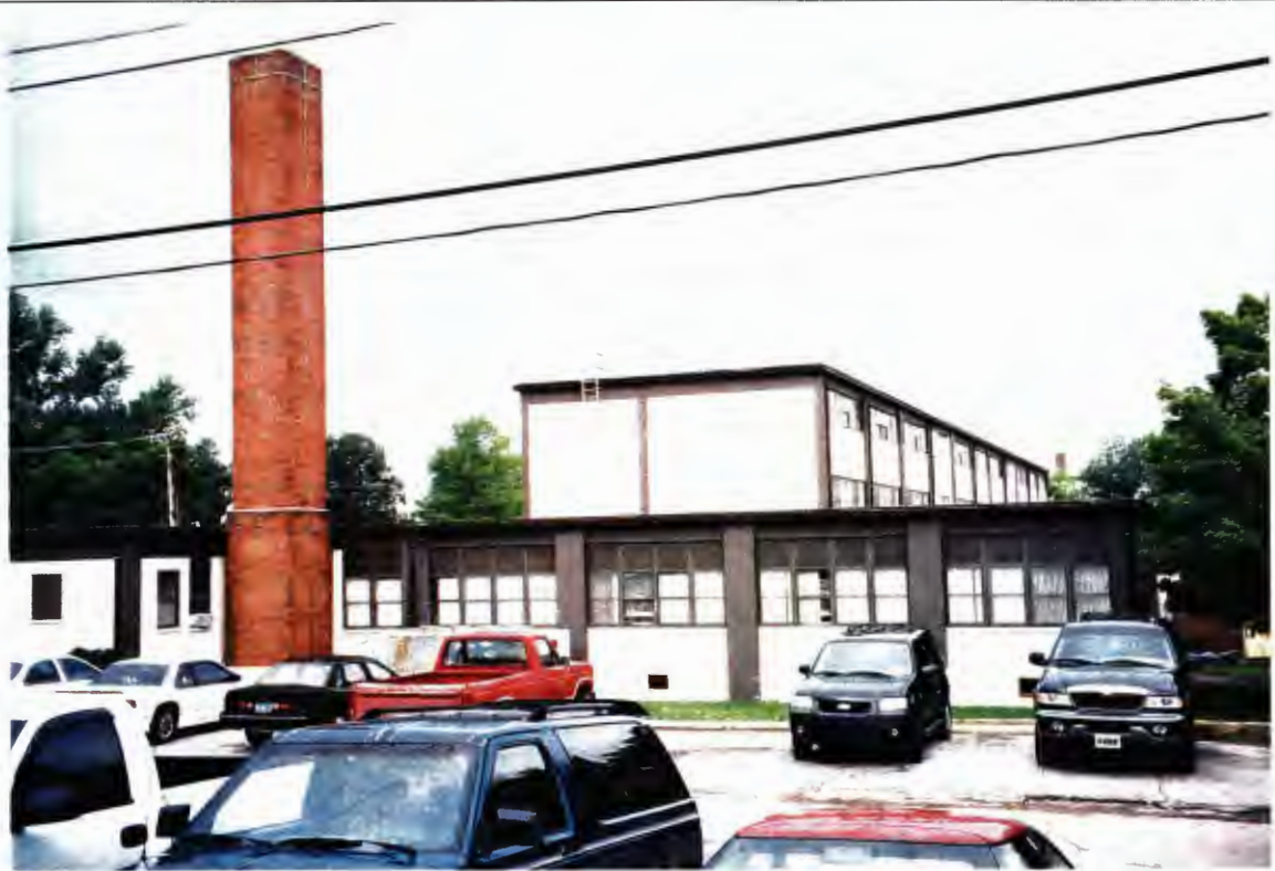
Building 6548- east elevation with large brick chimney
