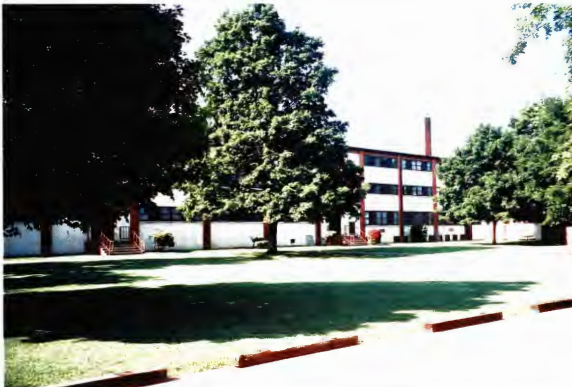
Building 1475 – north elevation of the handle portion where the barracks are located
