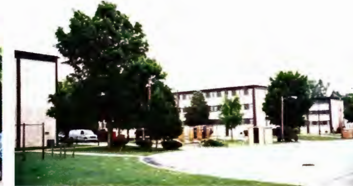
Oblique views of east and south elevations of Buildings 6546-left, 6547-middle, and 6548-right
