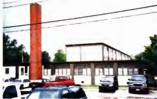
Building 6548 - east elevation with large exterior brick chimney
