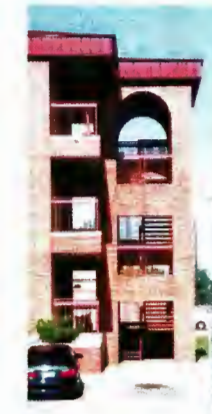
Building 1485 - close up of brick circulation addition on the north elevation
