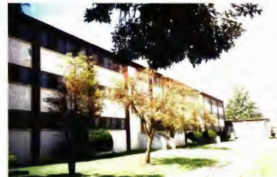
Building 2378 - north elevation of handle portion containing the barracks
