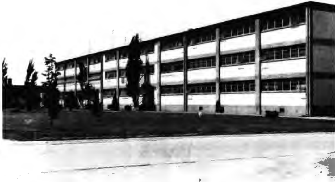
View of original ribbon awning windows (no date, Patton Museum Vol. 2)
