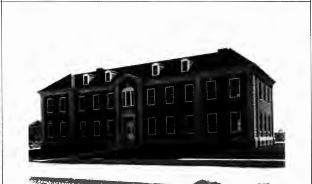
Figure 22: Administration building, more commonly known as the headquarters, was completed in 1934 (Images of America: The United States Army at Fort Knox).
