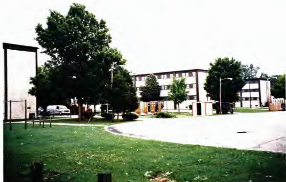
East elevations of Buildings 6546, 6547, and 6548 (right to left)
