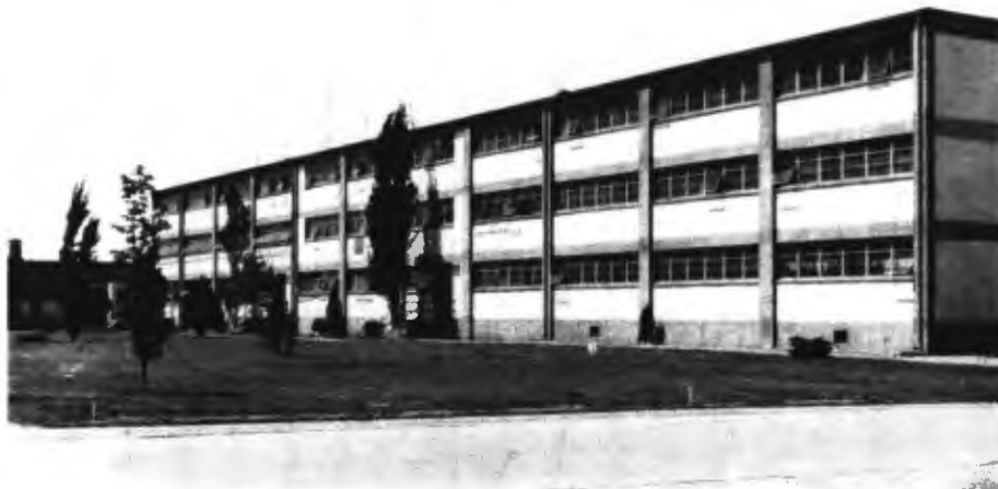
Figure 28: Typical 225-man hammerhead barracks constructed at Fort Knox in the regimental areas, no date for the photo (Patton Museum; Vol. 4).
