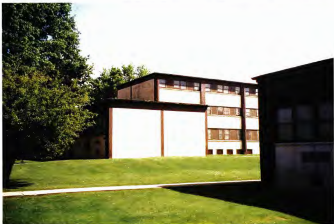
Building 2379 – oblique view of the south and west elevation of the tail portion
