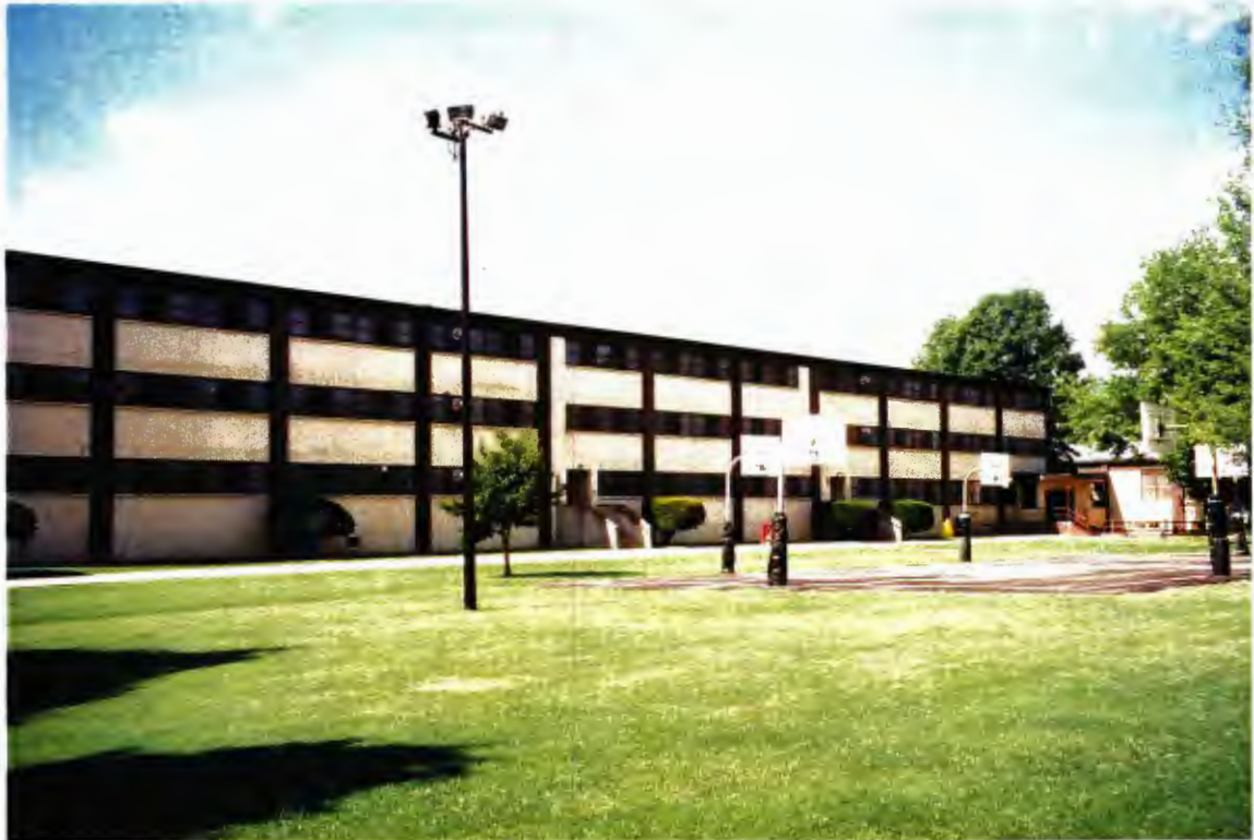
Building 2379 – north elevation of the handle portion where the barracks are located
