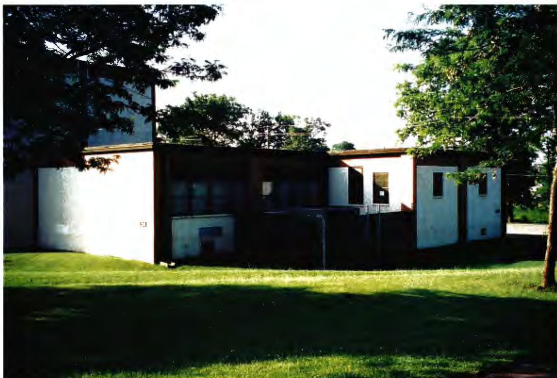
Building 296 - northwest elevation of the tail
