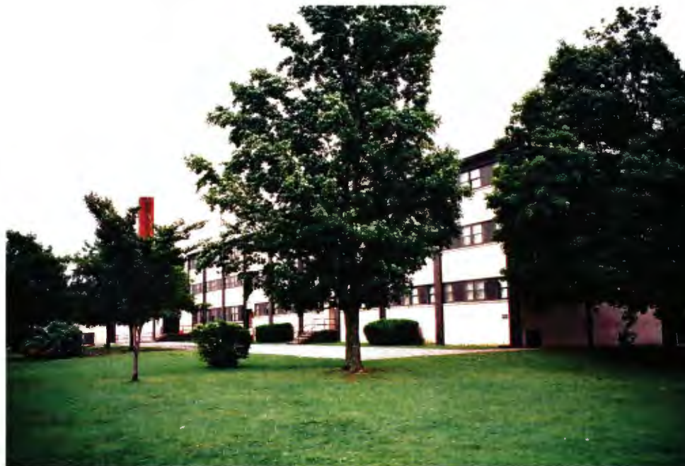
Building 6544 - north elevation of the handle portion where the barracks are located
