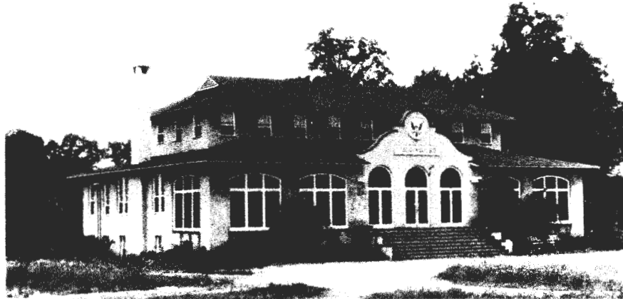
Figure 15: The Hostess House, originally constructed in 1919, was used in the early 1930s to house the influx of enlisted men and their families as they were assigned to the new mechanized cavalry at Fort Knox (Images of America; The United States Army at Fort Knox).
