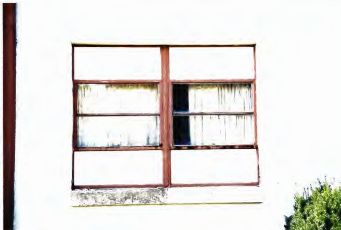
Building 2370 – original steel awning window
