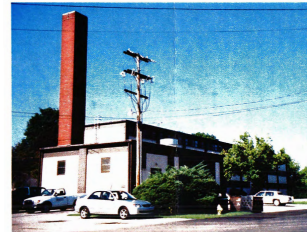
Building 6553 - oblique view of the north and east elevations and the large exterior brick chimney
