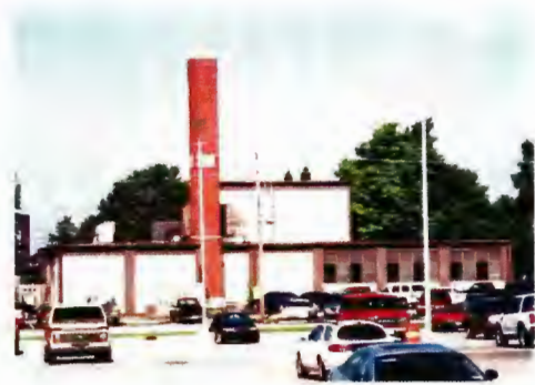
Building 2373 - east elevation of head and tail portions with brick chimney
