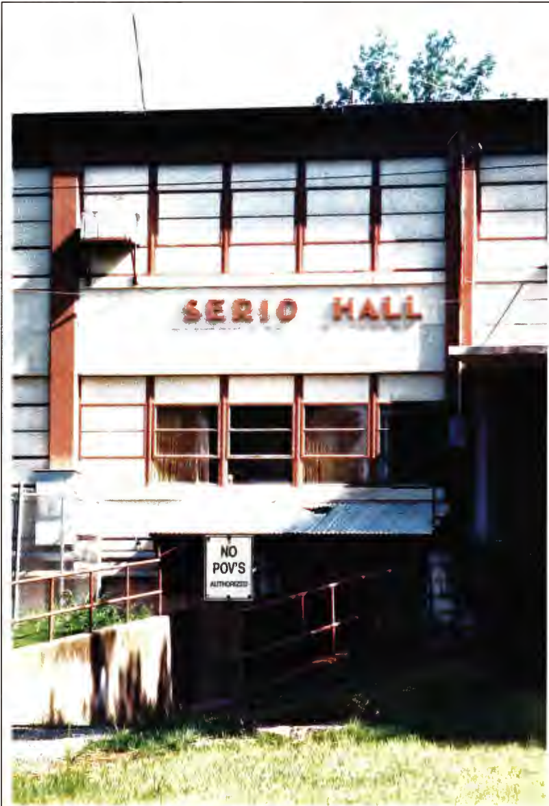
Building 2370 – a close up of the service bay
