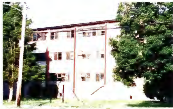
Building 297 - southeast elevation of the handle portion containing the barracks
