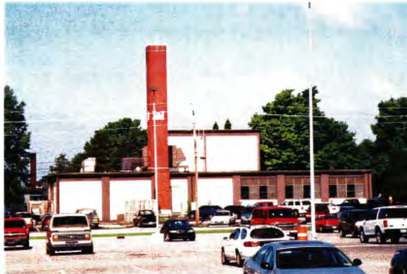
Building 2373 – east elevation with large exterior brick chimnenny
