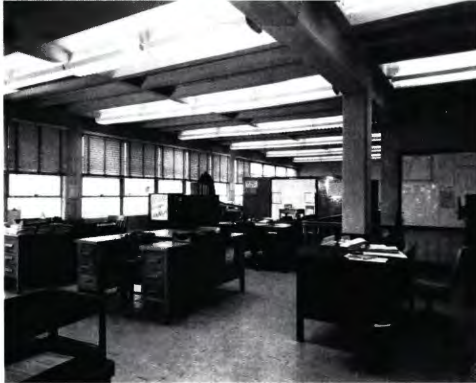
Interior view of Building 2370 depicting the concrete frame supports; similar to Building 6559 12 February 1957 (National Archives College Park)
