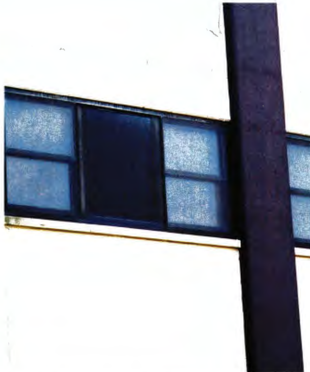
Current painted concrete and concrete block with anodized aluminum replacement windows
