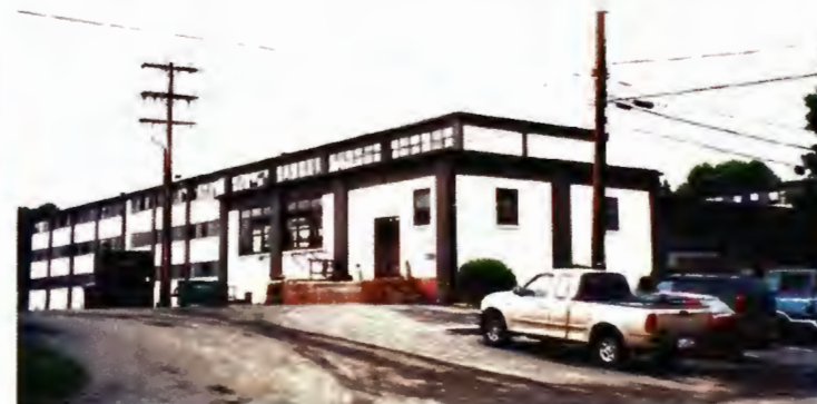
Building 6551 - oblique view of the north and west elevations
