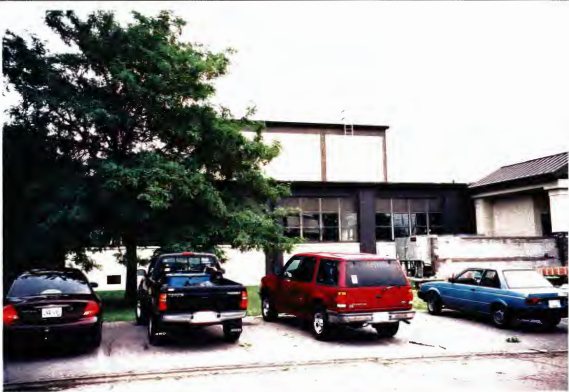
Building 6543 – west elevation with new addition on far right side
