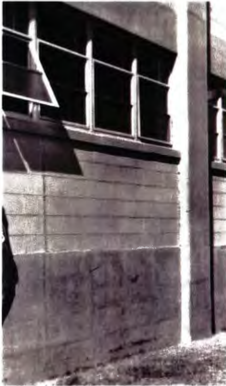
Original unpainted exposed concrete and concrete block with original steel awning windows
