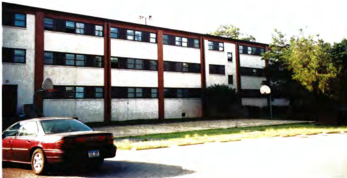
Building 297 – north elevation of the handle where the barracks are located
