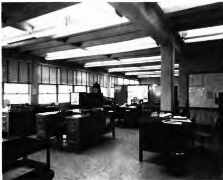
Building 2370 – interior view depicting the concrete supports 12 February 1957 (National Archives College Park)
