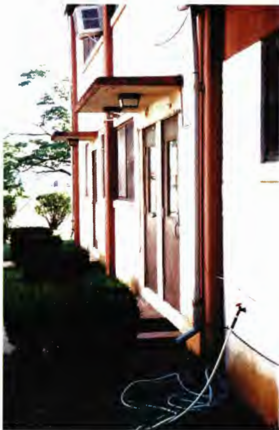
Building 1477 - close up of metal canopies on the west elevations
