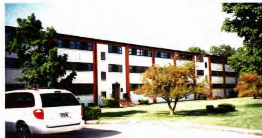
Building 1479 - south elevation of handle portion containing the barracks
