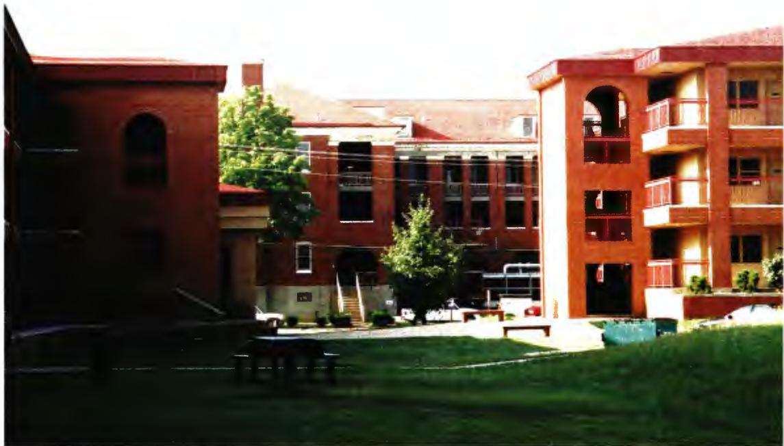
Building 1482 is located on the right side and Building 1485 located on the left side; showing arch comparisons on new additions with the original design of the 1930s brick barracks in the middle
