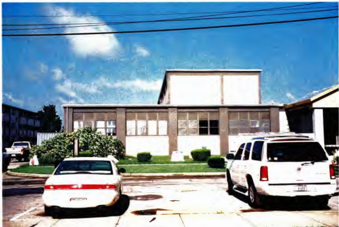
Building 6556 – east elevation with addition on the far right side
