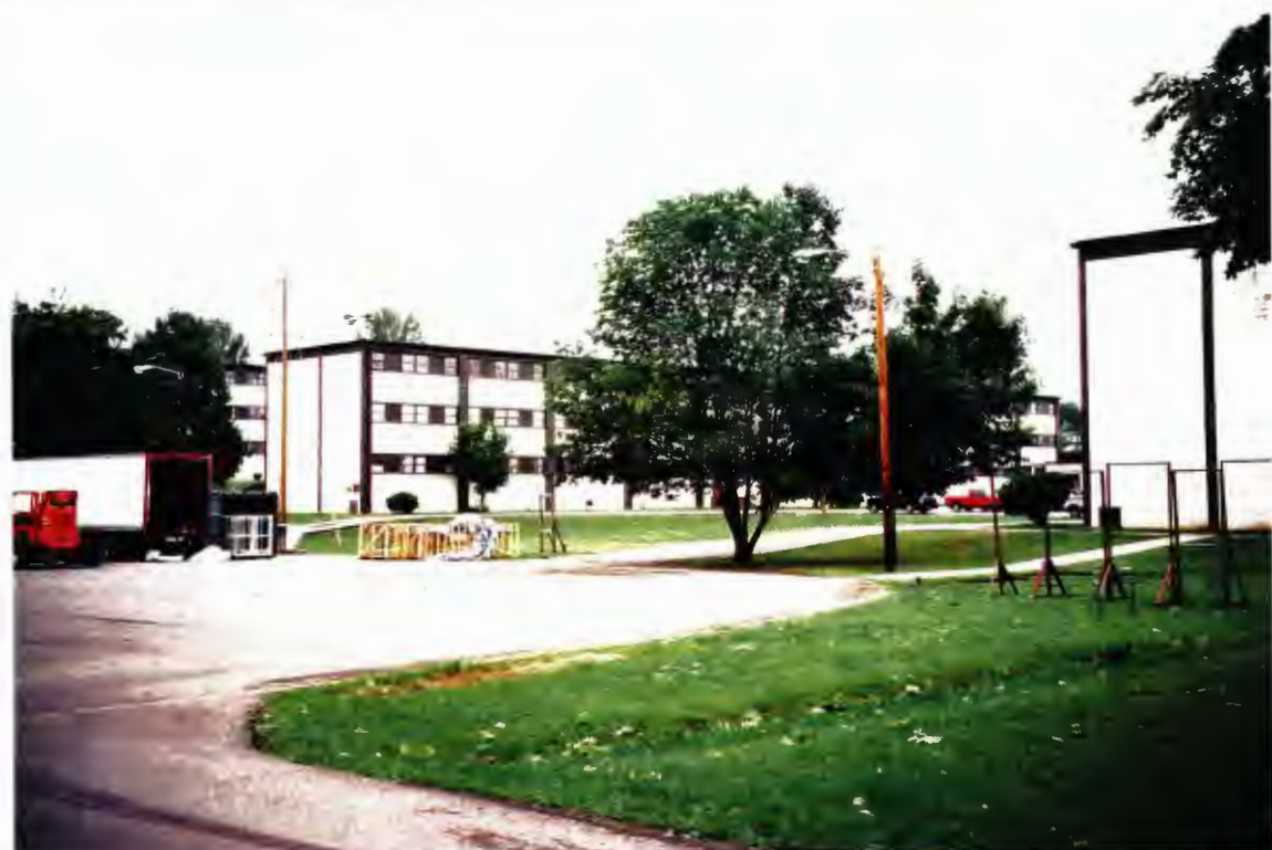
East elevations of Buildings 6541, 6542, and 6543 (left to right)
