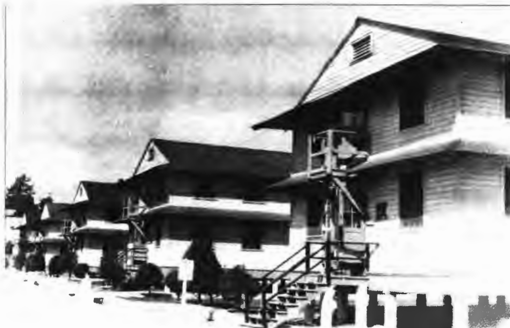
Figure 26: Two-story wooden barracks of the 700 and 800 series were constructed at Fort Knox (Images of America: The United States Army at Fort Knox).
