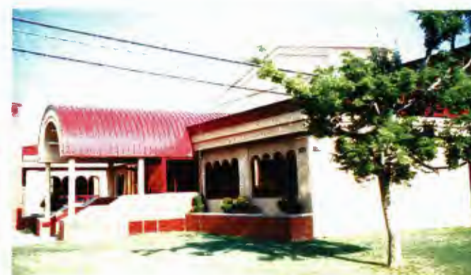
Building 1486 - new entrance located on the tail portion of the south elevation containing the mess hall
