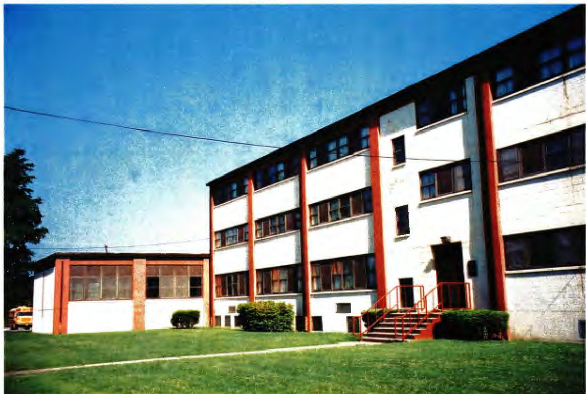
Building 1474 – south view of the handle and tail
