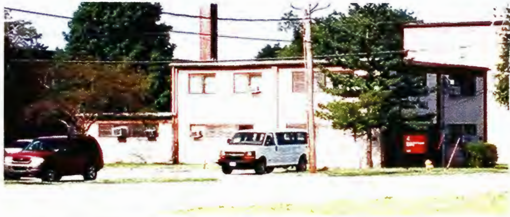
Building 1477 - oblique view of the north and east elevations
