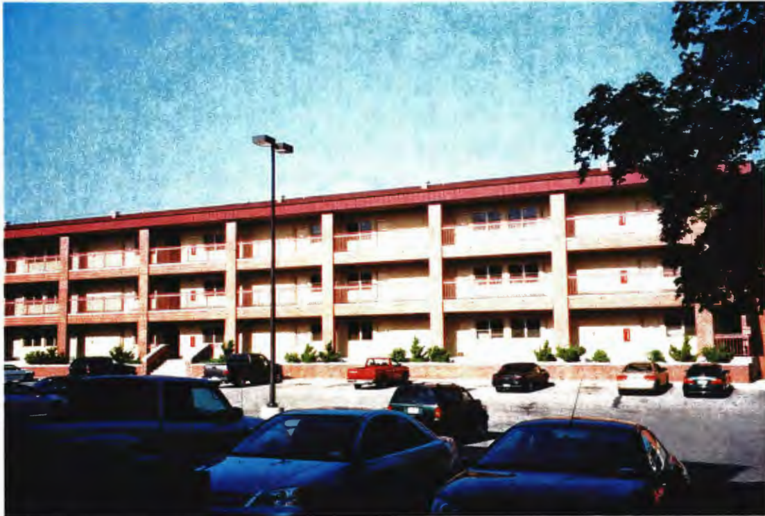
Figure 38: Under the One-Plus-One program in the 1990s, some hammerhead barracks were modified extensively to include exterior balconies, apartment-like rooms, brick veneer exterior walls, and exterior circulation towers (ERDC-CERL).
