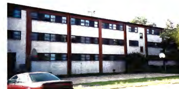
Building 297 - northeast elevation of the handle portion containing the barracks
