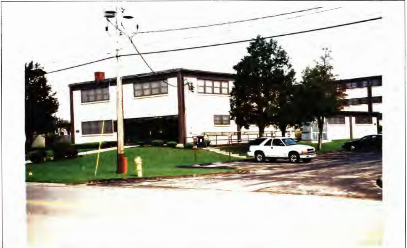
Building 2382 – south elevation with front entrance enclosed with glass
