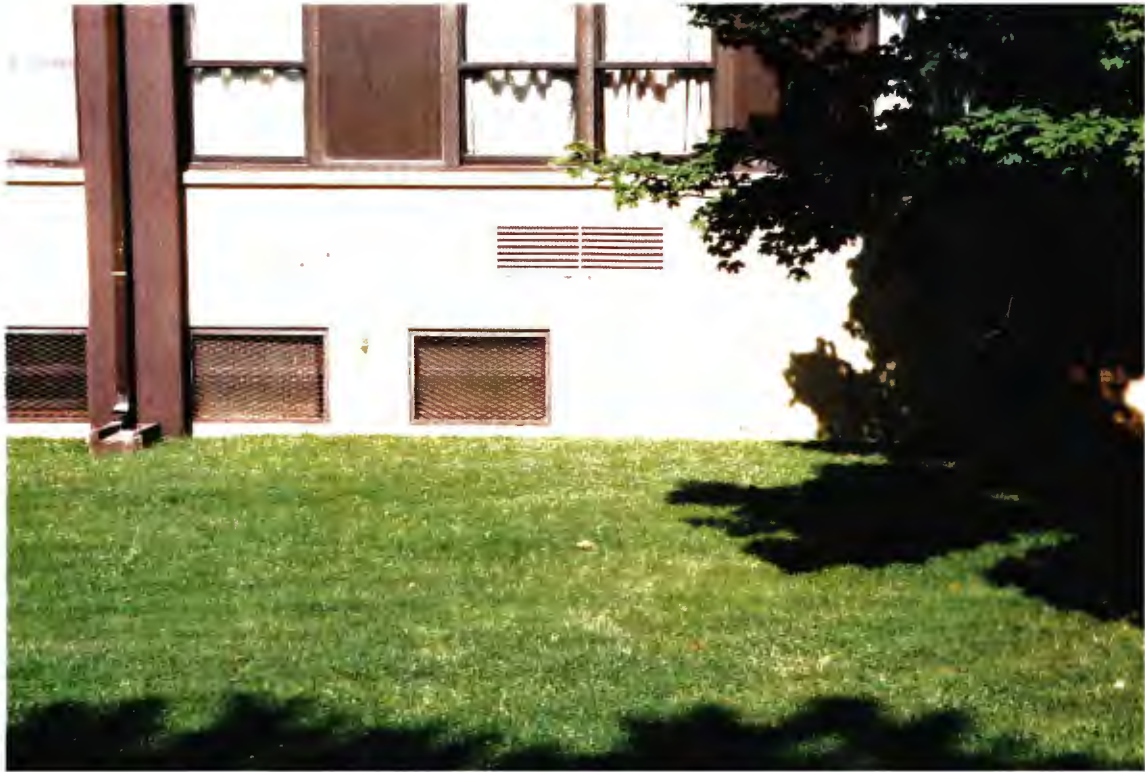
Building 2376 – basement window filled in with brick on the east elevation
