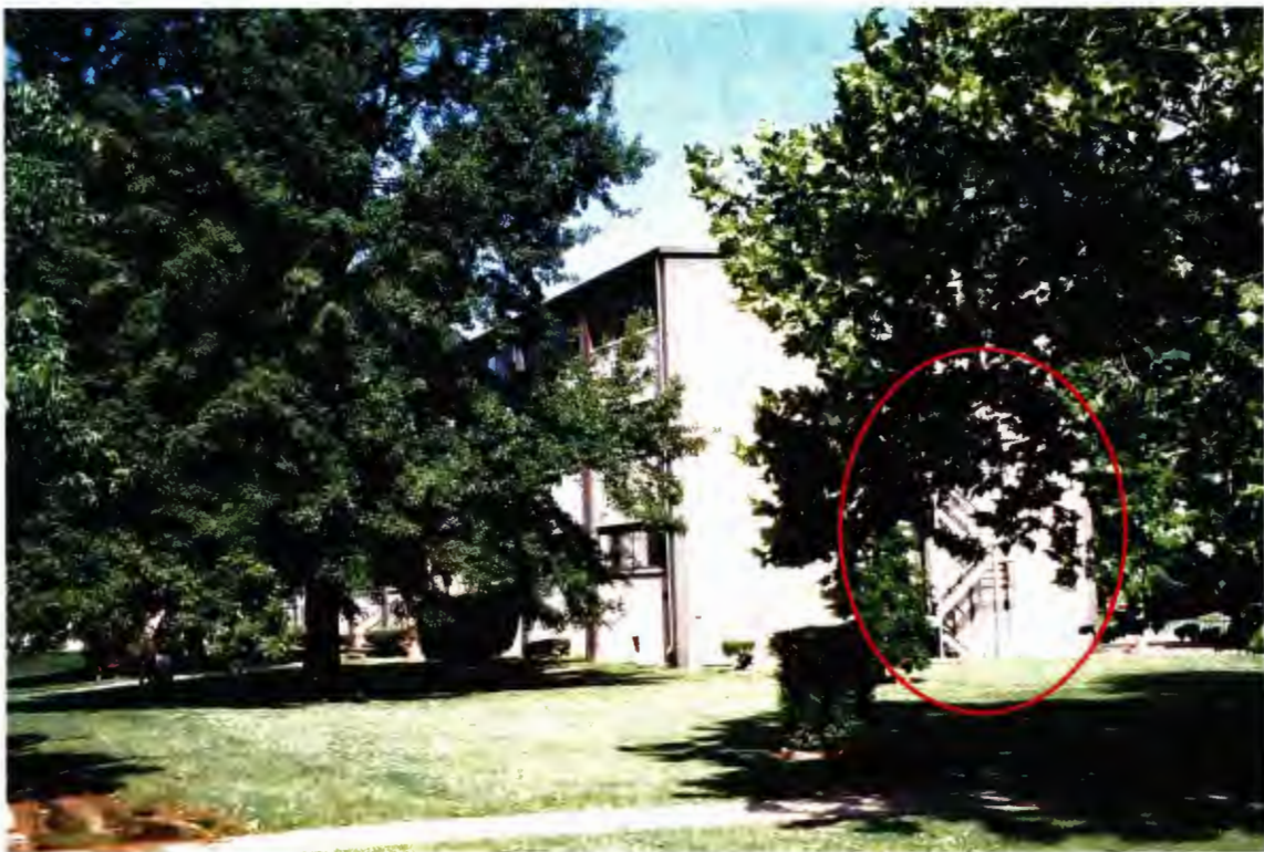
Building 6554 – east elevation with exterior staircase addition
