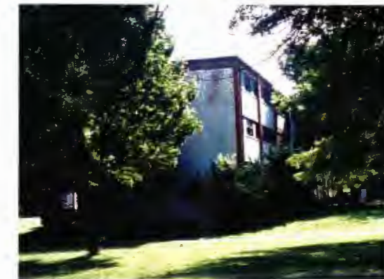
Building 1480 - west elevation of handle portion containing the barracks
