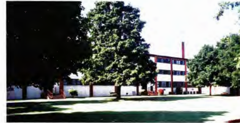
Building 1475 - north elevation of handle portion containing the barracks with exterior brick chimney protruding from the head portion which is the kitchen area
