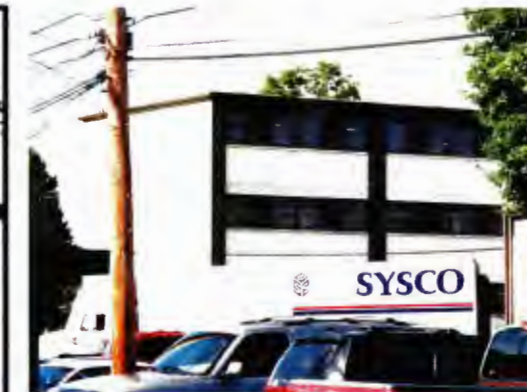
Building 6558 - oblique view of the north and east elevations
