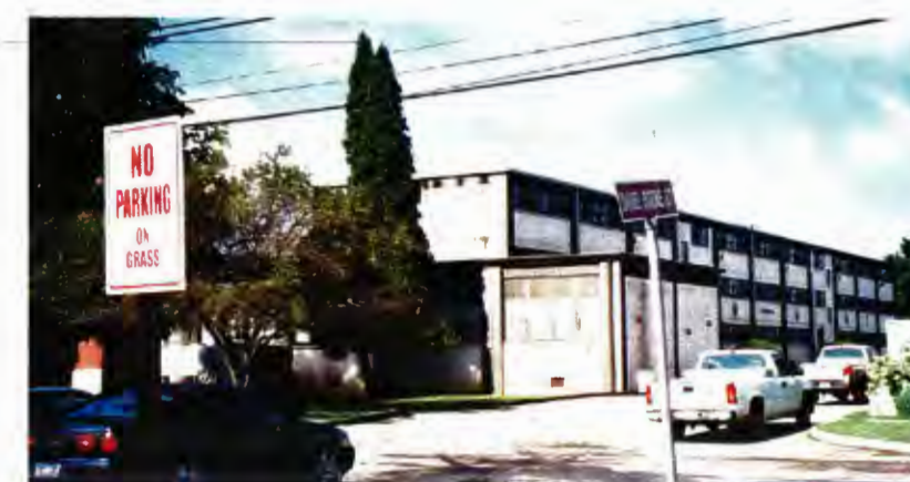
Building 6557 - oblique of the north and east elevations
