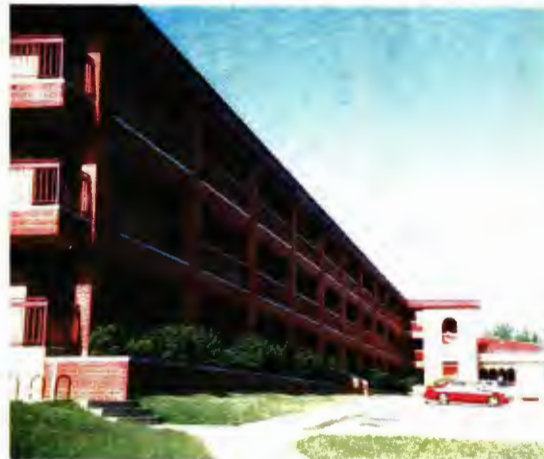
Building 1483 - north elevation of handle portion containing the barracks with addition of exterior brick balconies and circulation tower
