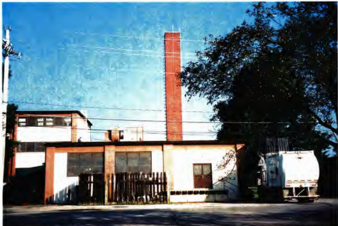
Building 297 – southeast elevation of the head where the kitchen is located
