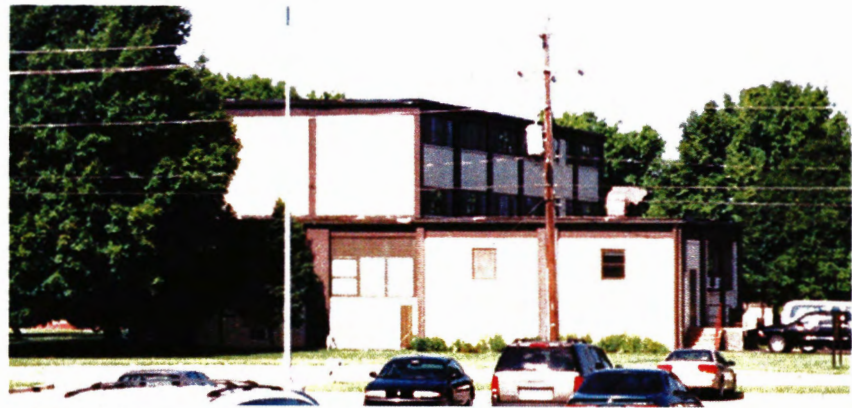
Building 2371 - east elevation of the head portion containing the kitchen
