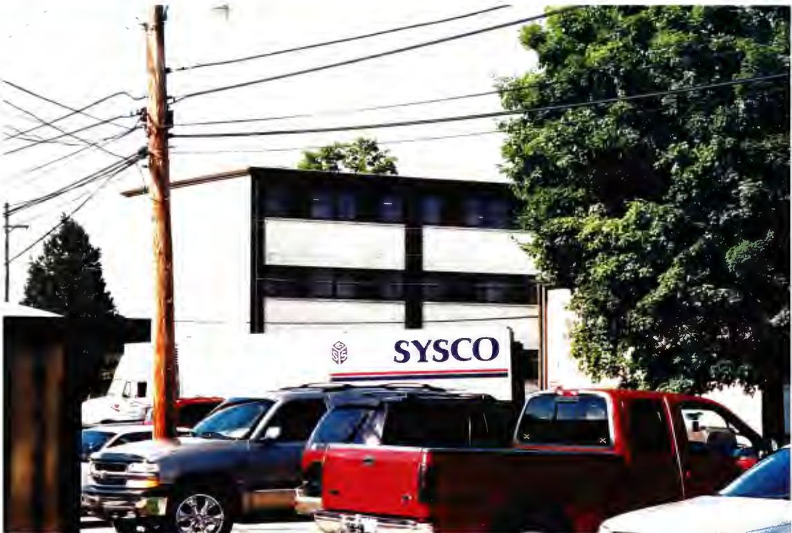
Building 6558 – oblique view of the north and east elevation of the handle portion
