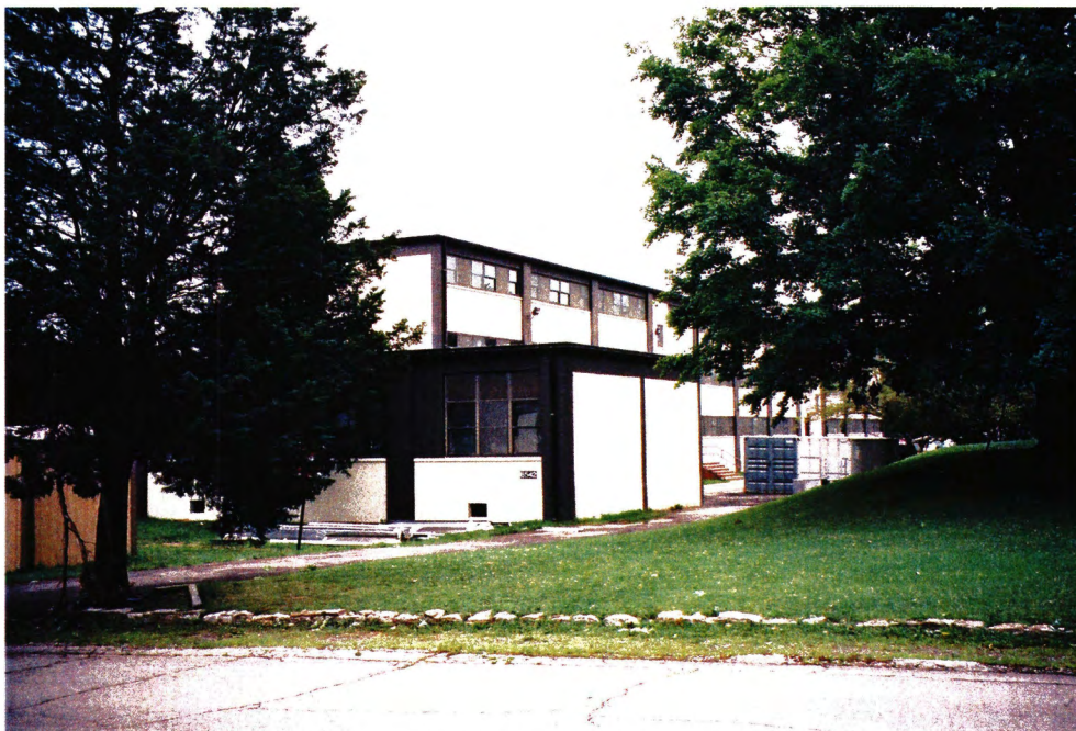
Building 6552 – west elevation of the tail portion where the mess hall is located
