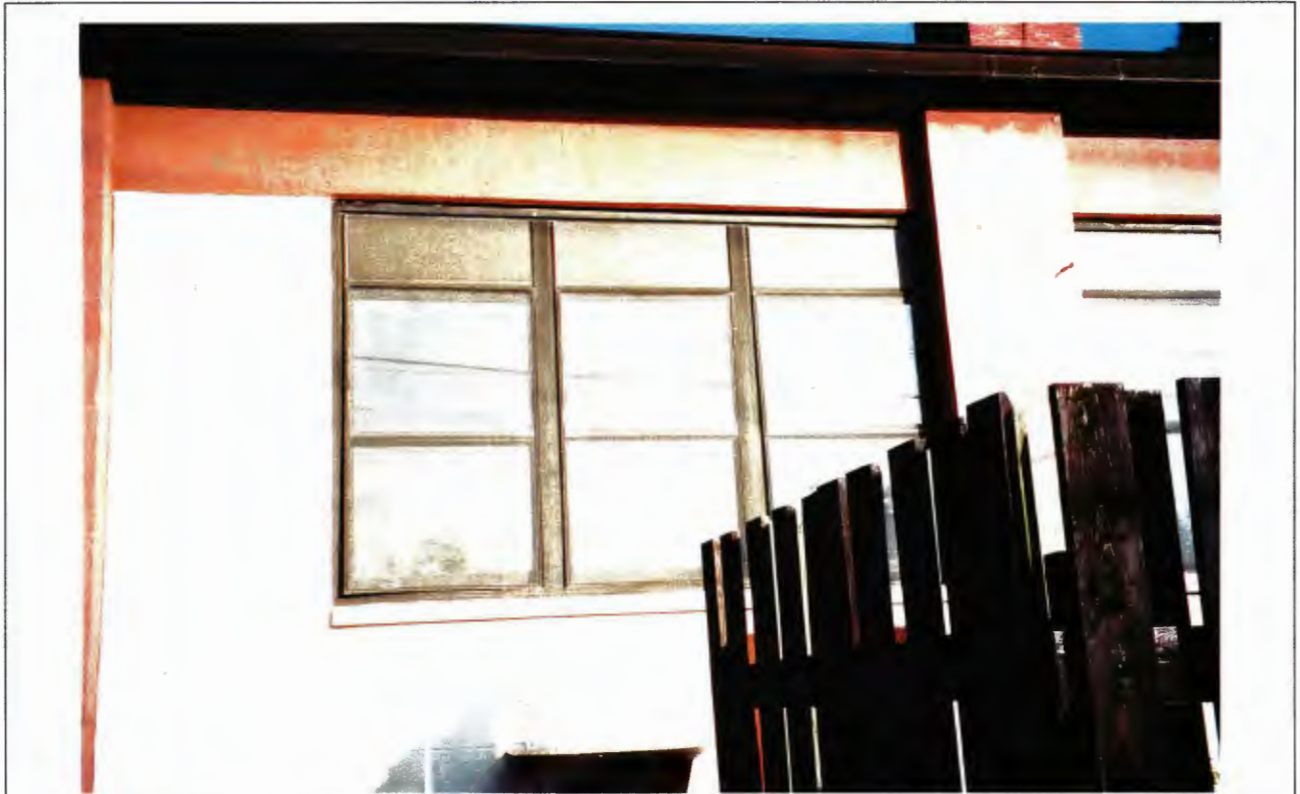
Building 297 – replacement anodized bronze aluminum window located on the head portion
