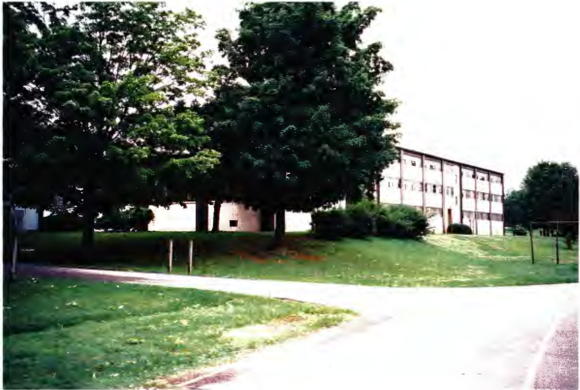
Building 6545 – north elevation of the handle portion where the barracks are located
