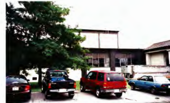
Building 6543 - west elevation of the head and tail portions
