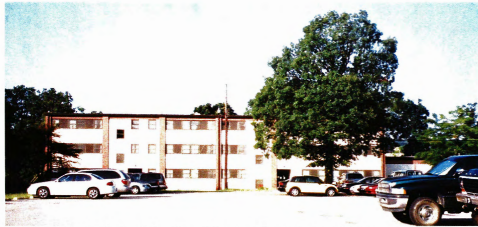
Building 296 - northeast elevation of the handle portion containing the barracks
