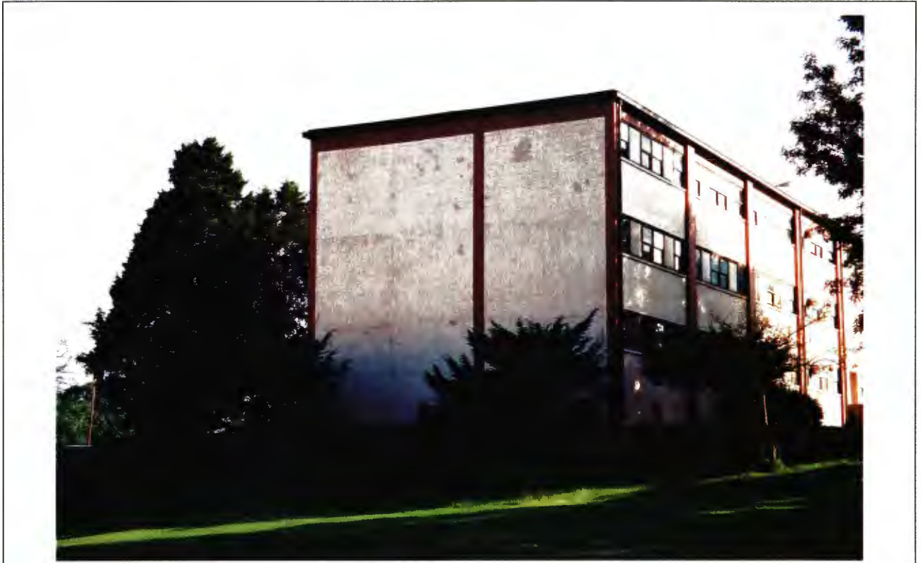
Building 297 – south elevation of the handle
