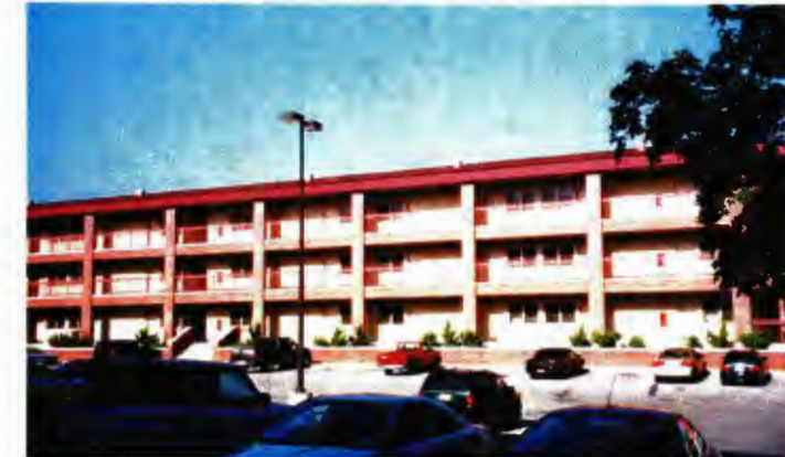
Building 1485 - east elevation of handle portion containing the barracks
