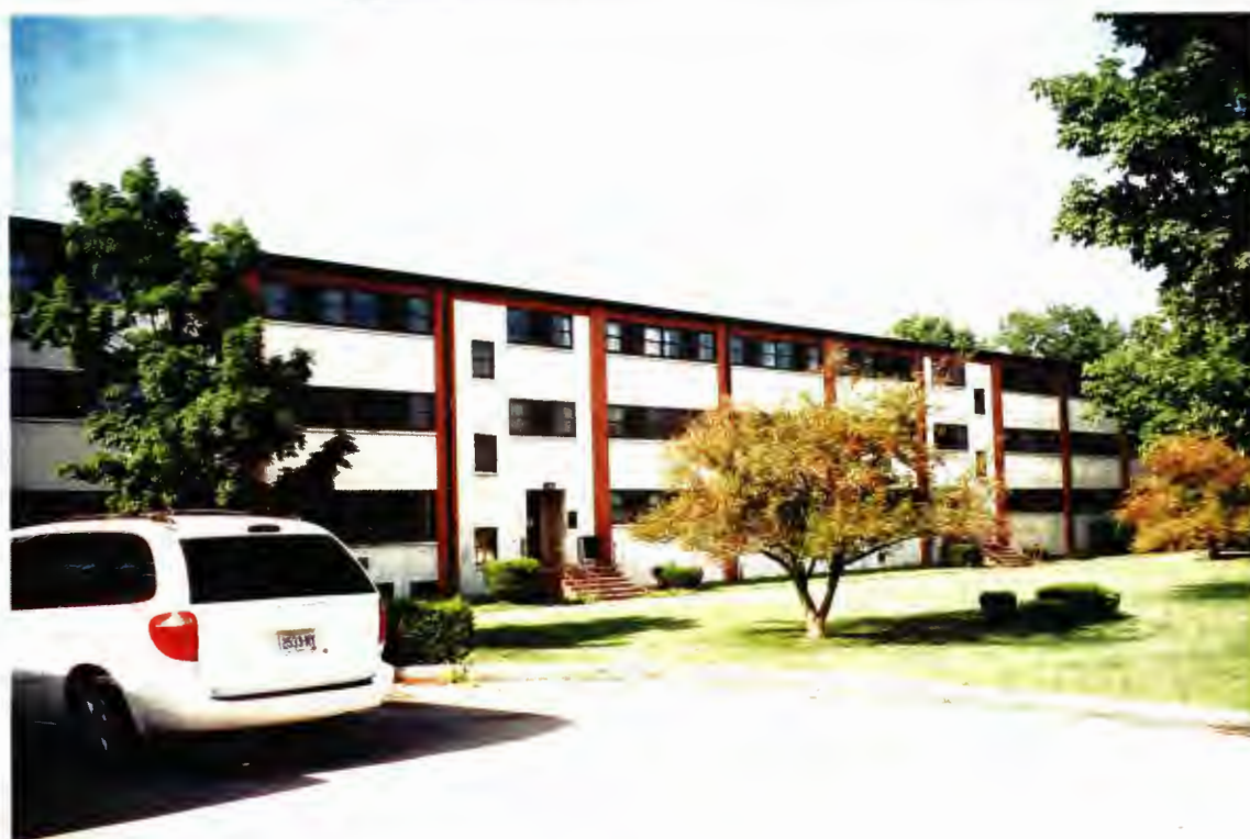
Building 1479 – south elevation of the handle
