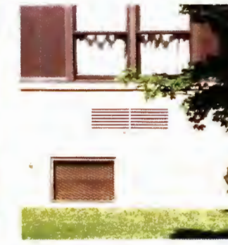
Building 2376 - basement window filled with brick and new air conditioning vent
