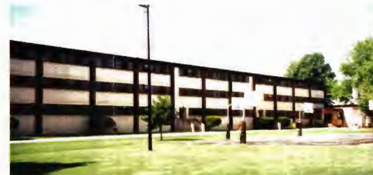
Building 2379 - north elevation of the handle portion containing the barracks
