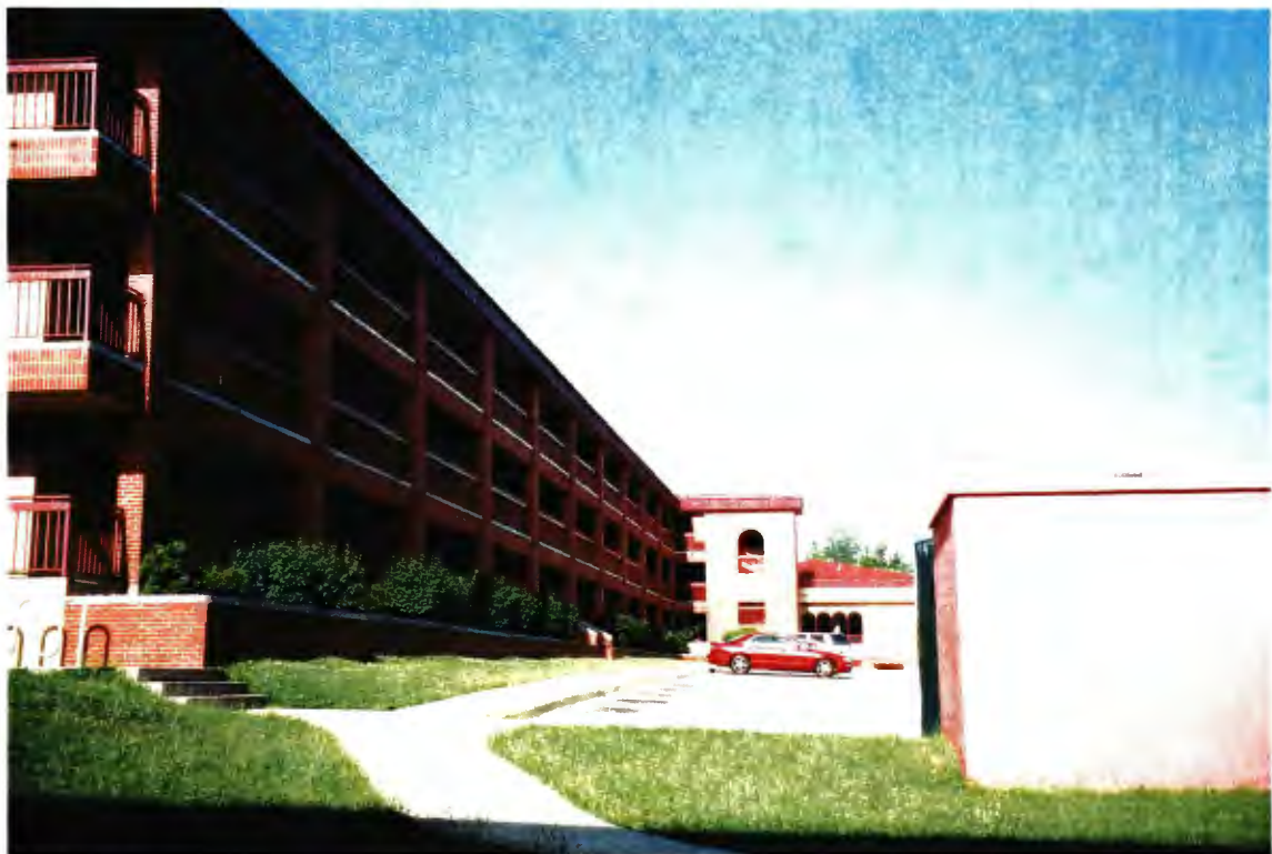
Building 1483 – north side of the handle portion where the barracks are located
