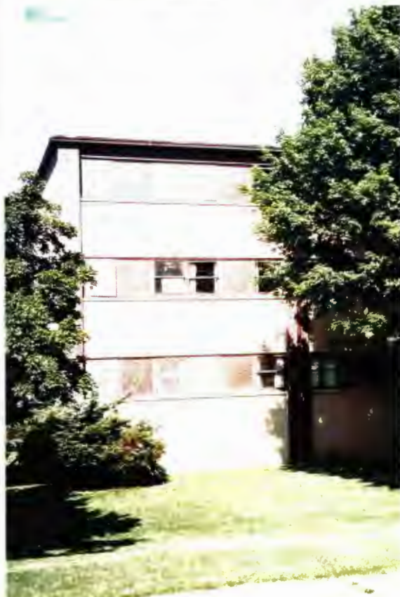
Building 2376 – one bay on the east elevation
