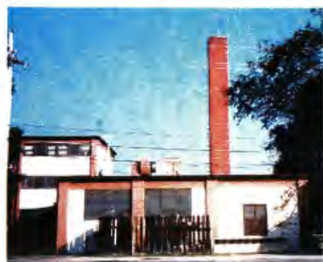
Building 297 - southeast elevation of the head portion containing the kitchen
