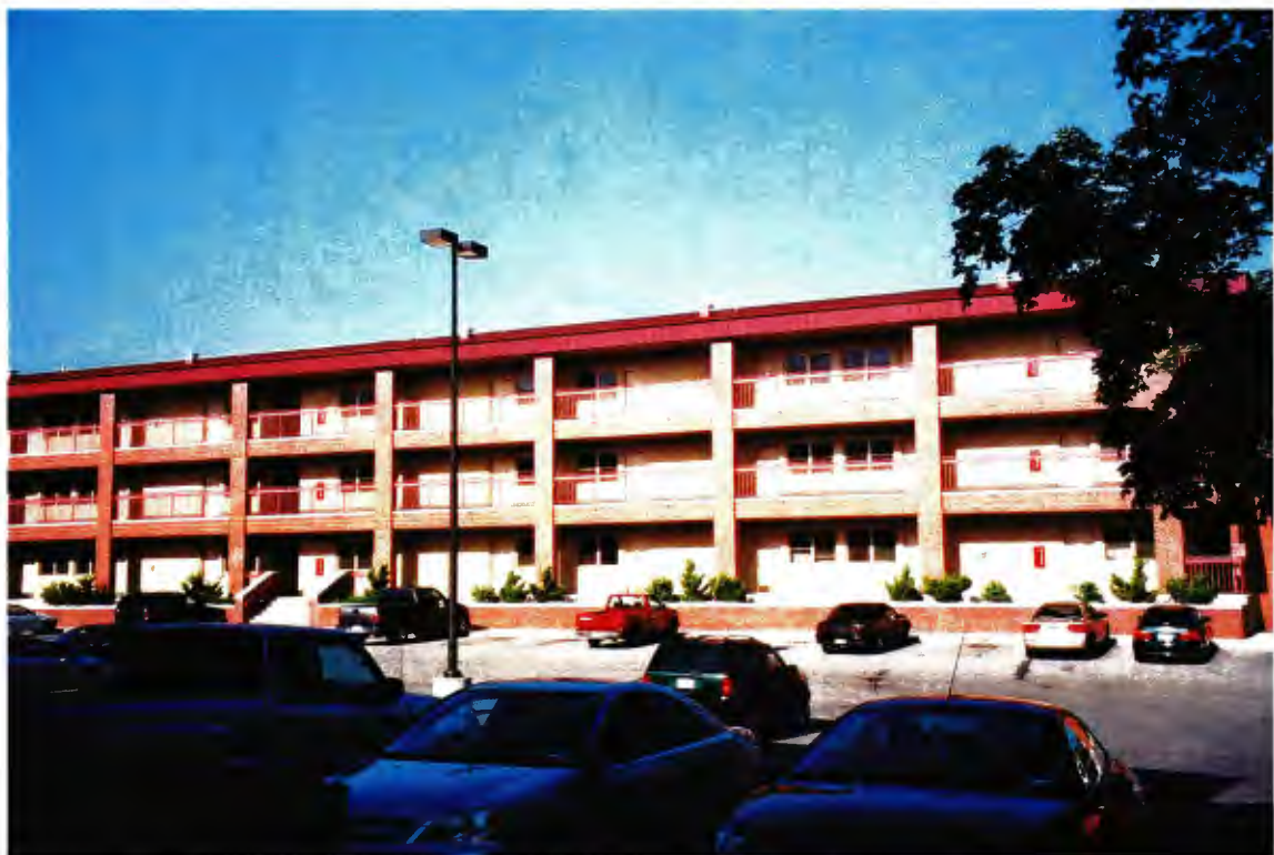
Building 1485 – east elevation of the handle portion of the renovated building
