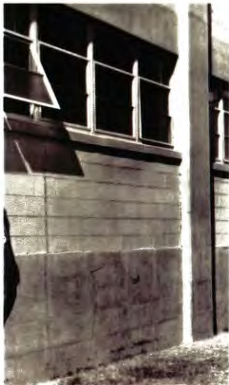
Original unpainted exposed concrete and concrete block with original steel awning windows
