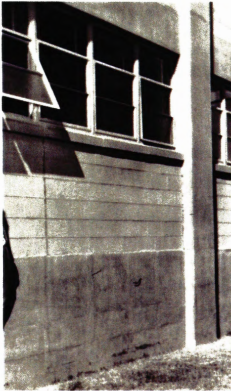
Original unpainted exposed concrete and concrete block with original steel awning windows
