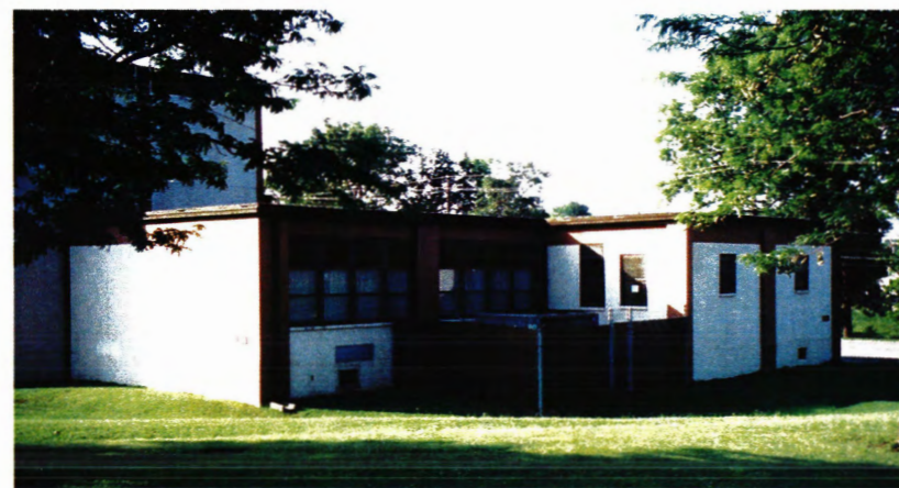
Building 296 - oblique view of northeast and northwest elevations of the tail portion containing the mess hall
