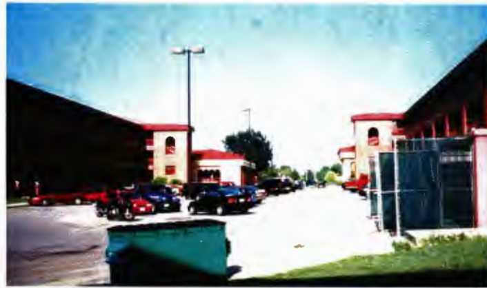
Building 1482 on left and Building 1483 on right-renovated 11 bay hammerhead barracks
