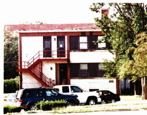
Building 1481 - north elevation
