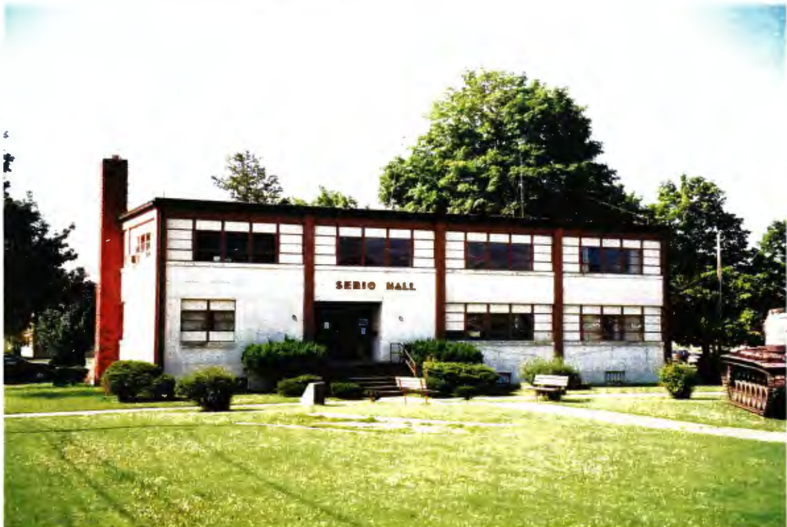
Building 2370 – north elevation
