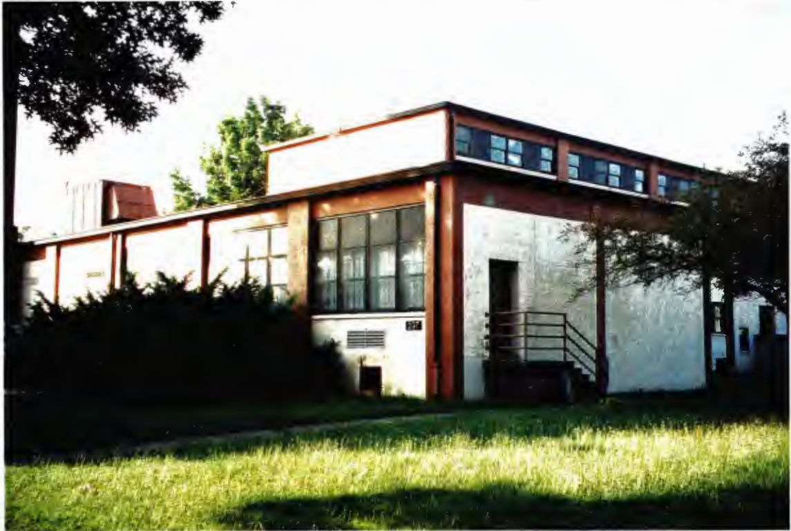
Building 297 – north elevation of the tail where the mess hall is located
