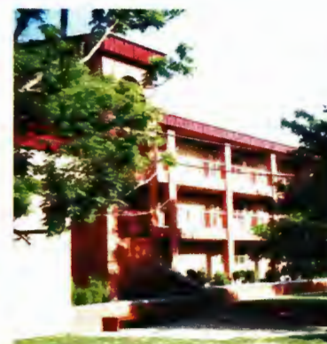
Building 1486 - east elevation of handle portion containing the barracks with addition of exterior brick balconies
