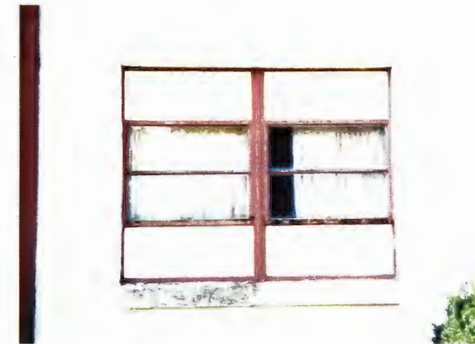
Building 2370 - original steel awning windows with replacement panels
