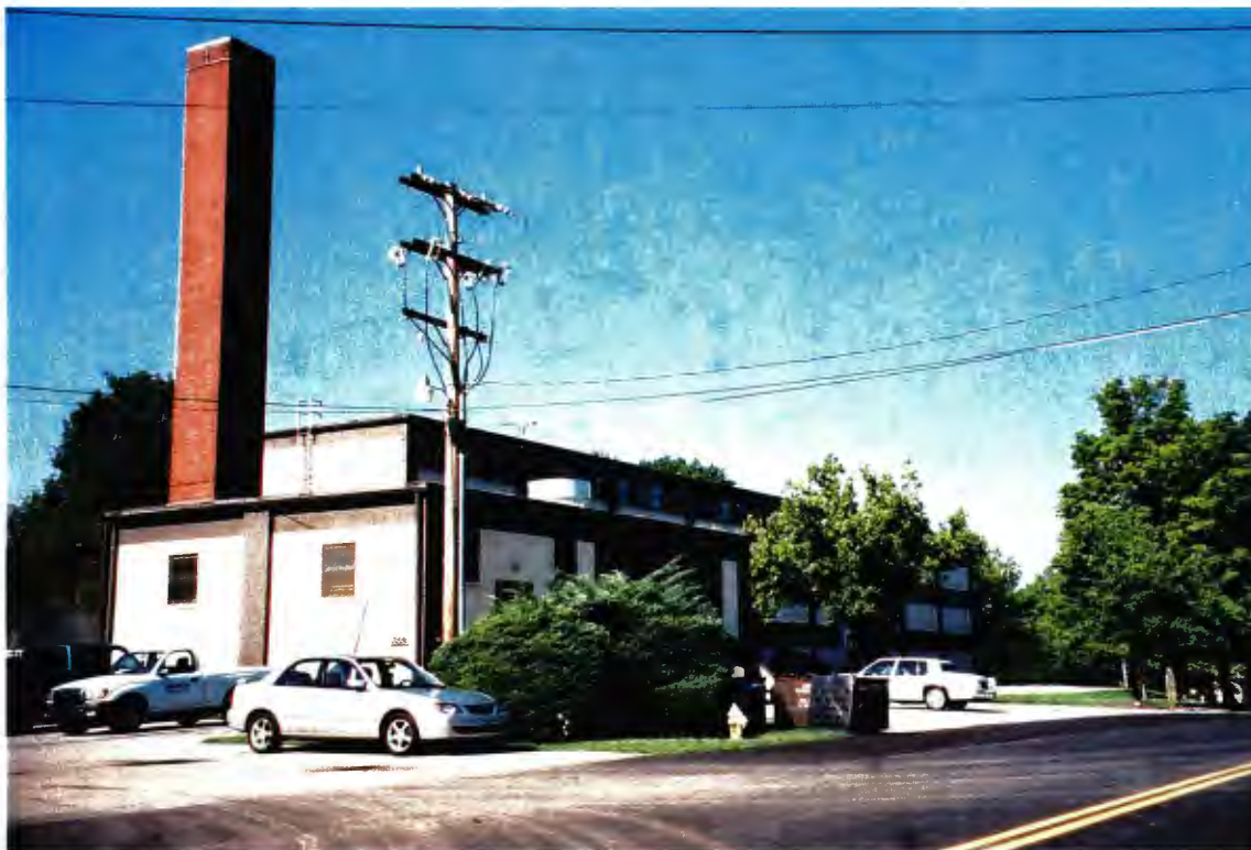
Building 6553 – oblique view of the north and east elevations
