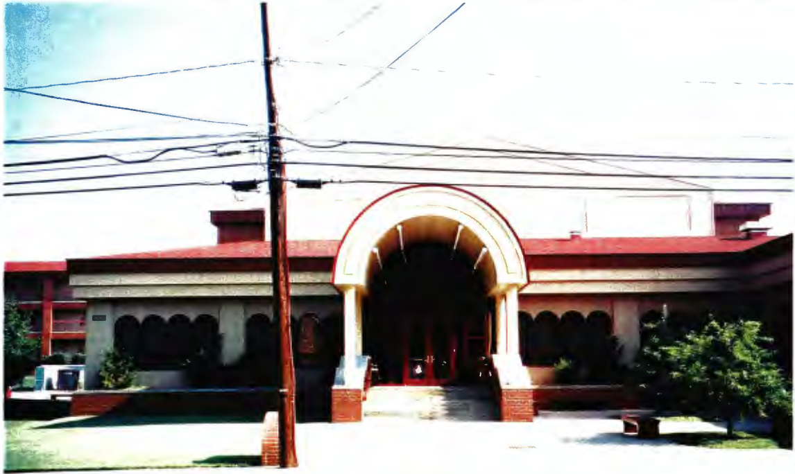
Building 1485 – new front entrance into the building, located on the south elevation
