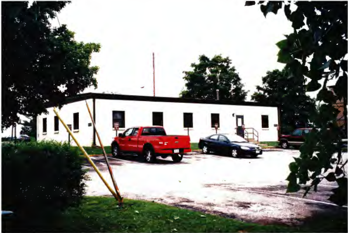
Building 6538 – north elevation
