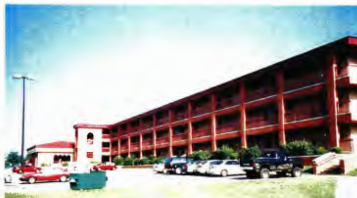
Building 1484 - south elevation of handle portion containing the barracks with addition of exterior brick balconies and large circulation tower
