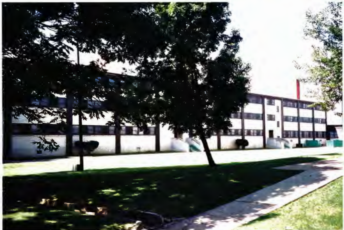
Building 2380 – north elevation of the handle portion
