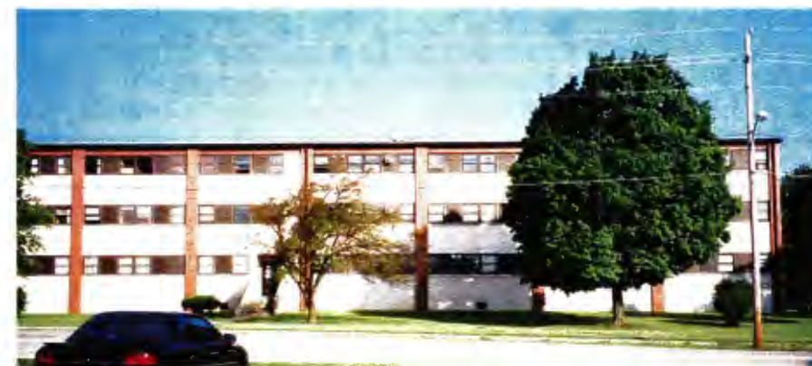
Building 298 - southeast elevation of the handle portion containing the barracks
