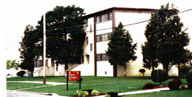
Building 2381 - oblique view east and south elevations of the handle portion containing the barracks
