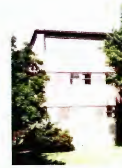
Building 2376 - one bay on east elevation
