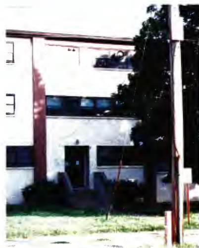
Building 297 - entrance bay on southeast elevation
