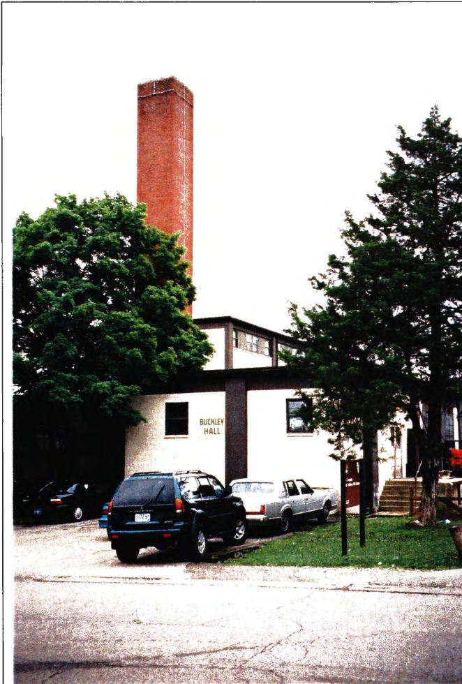
Building 6540 – east elevation with large brick chimney
