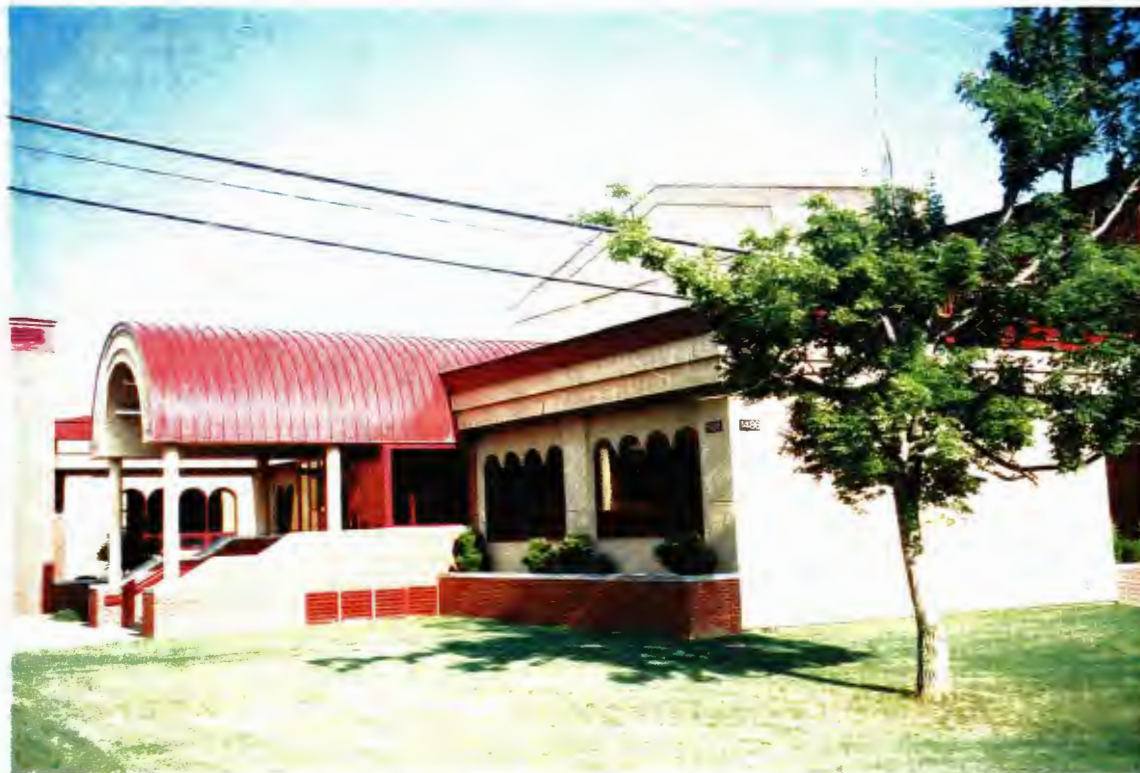
Building 1486 – new front entrance into the building, located on the south elevation
