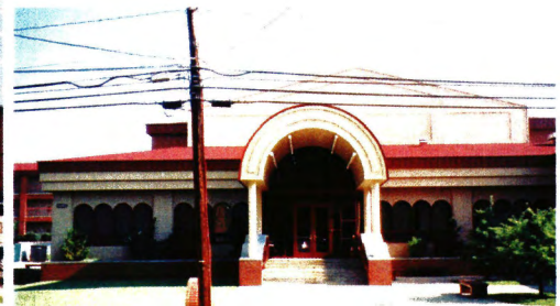
Building 1485 with 1994 renovation
