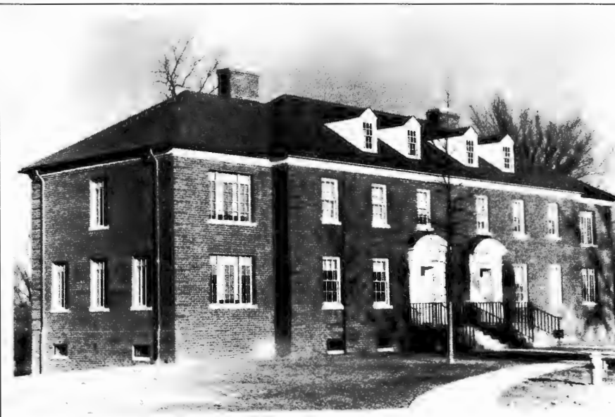
Figure 21: Permanent brick duplexes constructed for field officers and their families (Images of America: The United States Army at Fort Knox).
