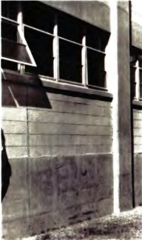
Original unpainted exposed concrete and concrete block with original steel awning windows
