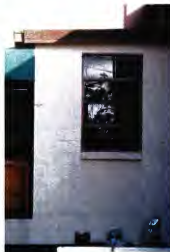
Building 297 - original steel awning window located on southeast elevation
