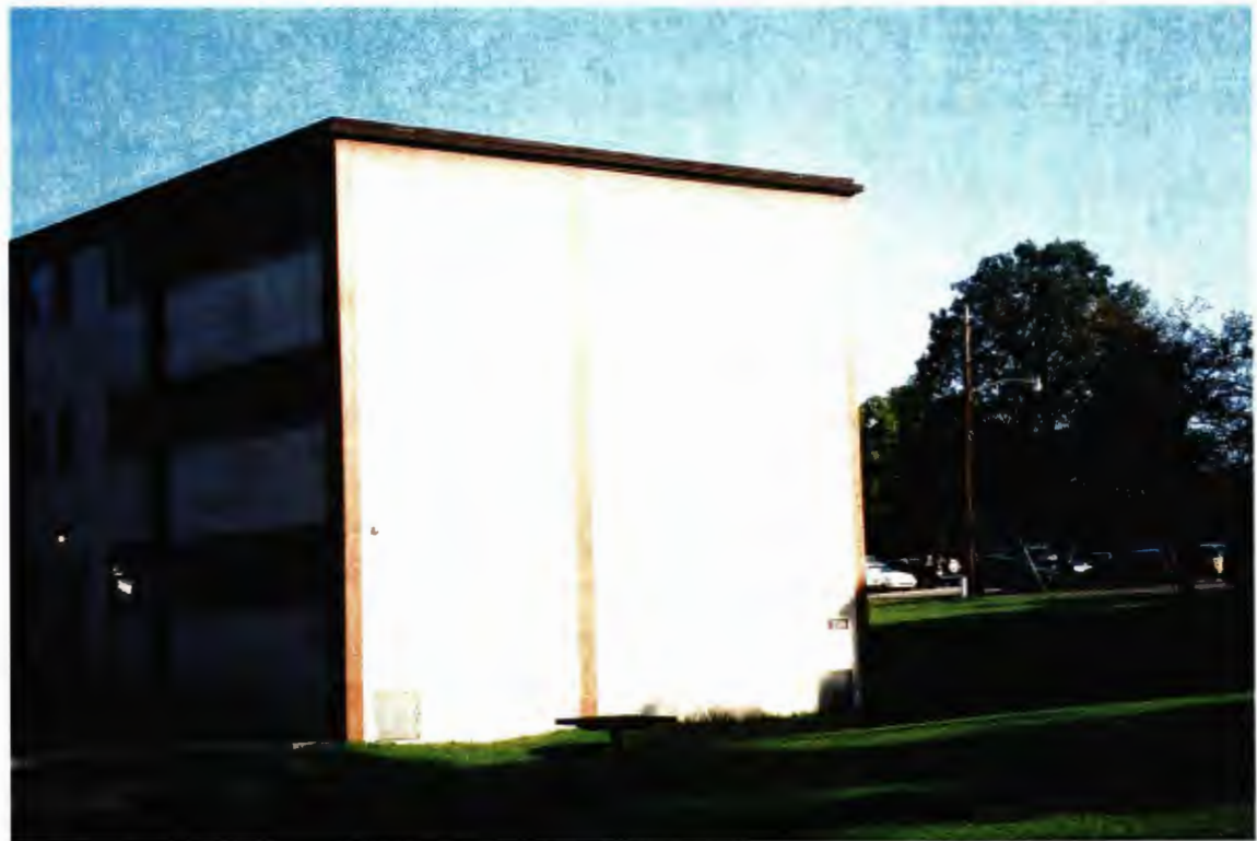
Building 296 – east elevation of the handle
