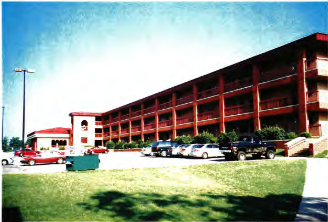
Building 1484 – south side of the handle portion of the renovated building
