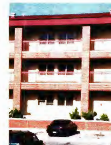
Building 1485 - close up of a renovated bay on east elevation
