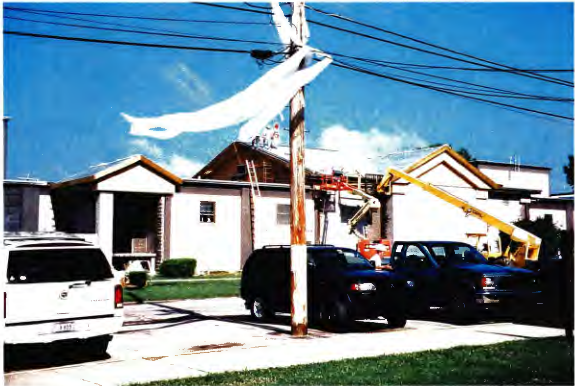
Building 6556 is located on the right of the new addition that connects to Building 6557 on the left
