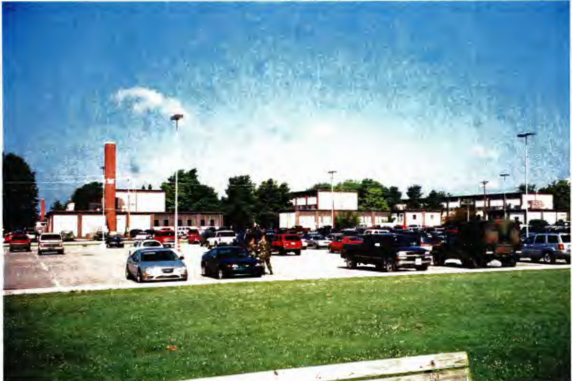
East elevations of Buildings 2373, 2374, and 2375 (left to right)
