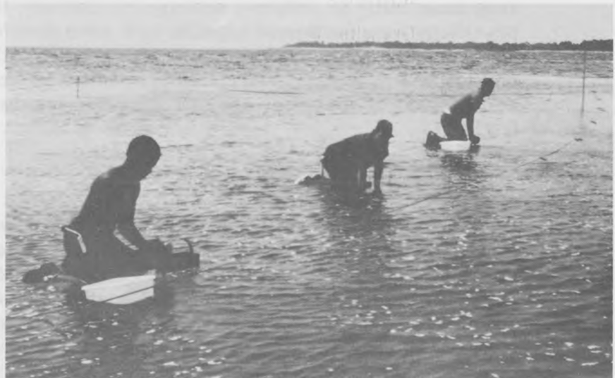
Seagrass transplanting operation on dredged material near Port St. Joe, Florida. In the absence of mechanical techniques, seagrass transplantation is now a labor-intensive effort.
