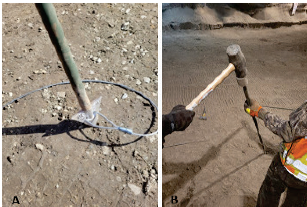
Figure 4-6. Arrowhead anchor installation. (A) Drive rod nested against arrowhead. (B) Two operators needed to install.
