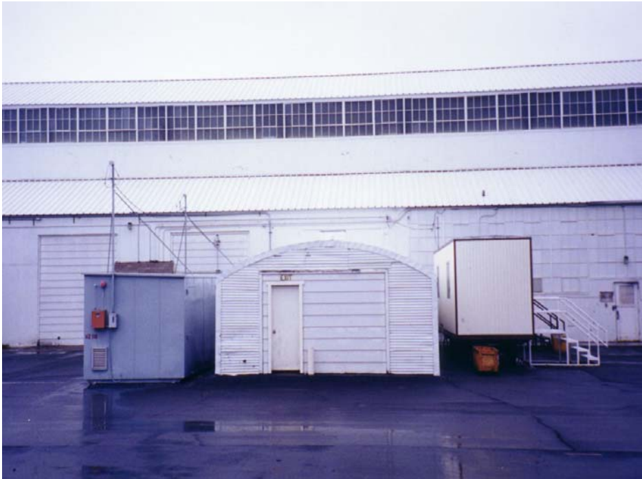
Figure K3. Main compressor room enclosure.
