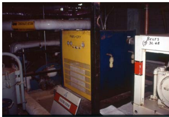
Figure G4. Building 345: 25 hp GD compressor. Figure G5. Building 345: ineffective air dryer.
