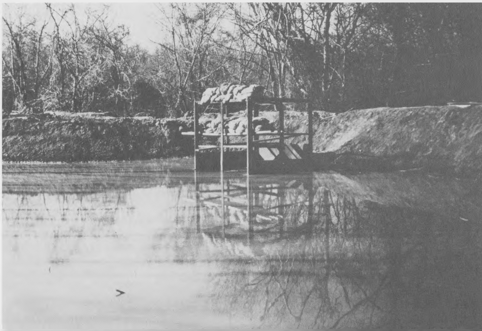
Photo 10. Richmond, Va., disposal area; view of ponded area in compartment 3 showing sluice used for effluent discharge
