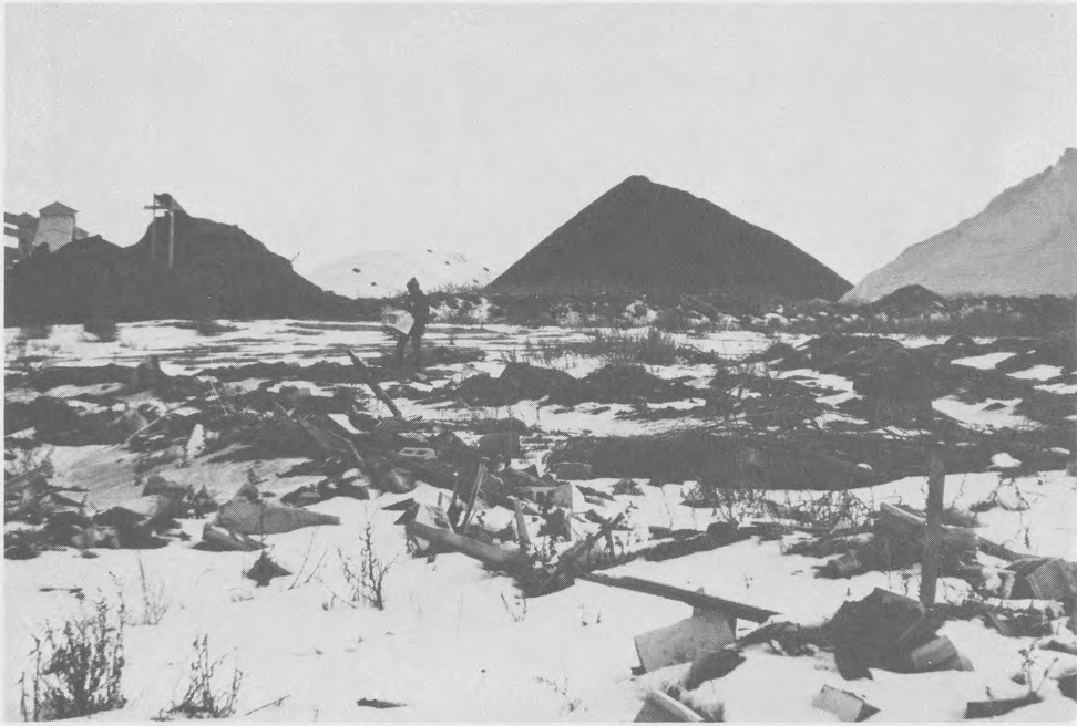
Photo 5. Grand Haven, Mich., disposal area; postdisposal view of containment area showing solid waste within the site and stockpiles of limestone, coal, and salt in the background beyond the dike. Influent pipe is shown to the upper left
