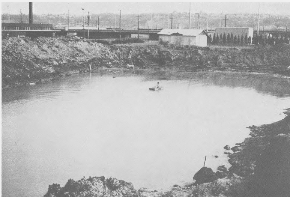
Photo 14. Seattle, Wash., disposal area; turbid water in compartment 2 resulting from precipitation of colloidal iron complexes in the aerated surface water. Effluent pumpout was from far right-hand corner
