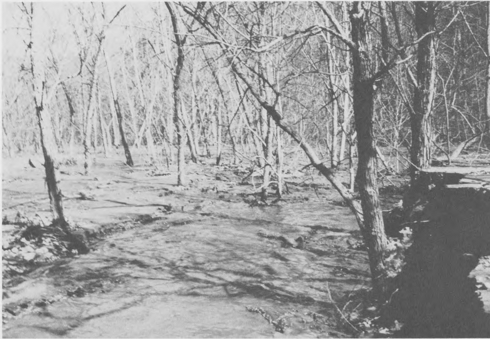
Photo 9. Richmond, Va., disposal area; view of overland flow in compartment 1 showing trees partly buried by sandy sediment
