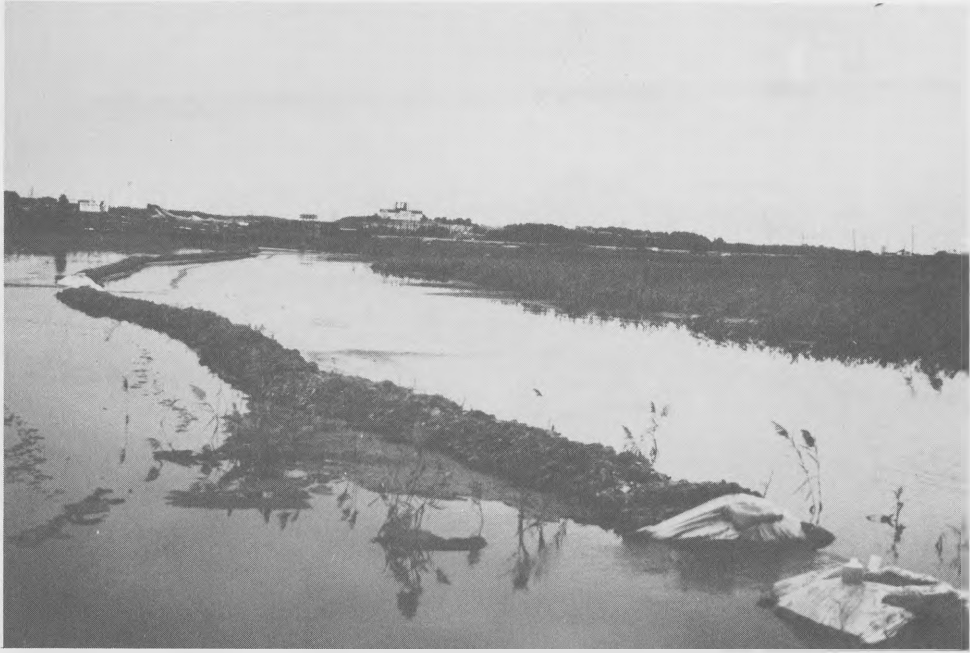
Photo 1. Sayreville, N. J., disposal area; cross-dike between compartments 2 and 3 and thick vegetation ( Phragmites communis ) in compartment 2
