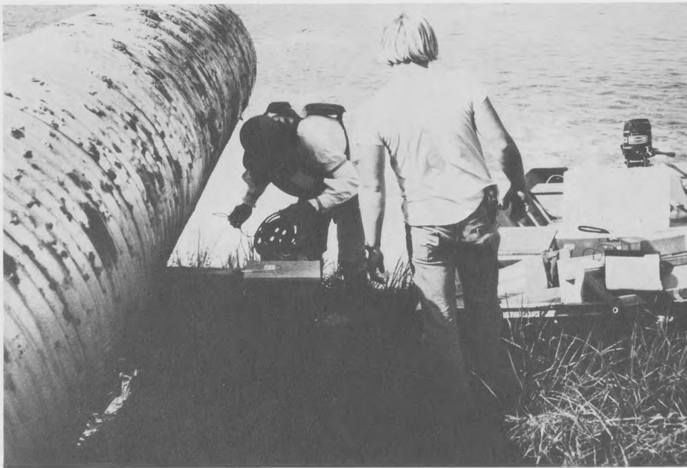
Photo 20. Southport, N. C., disposal area; view of effluent collection at end of sluice discharge pipe
