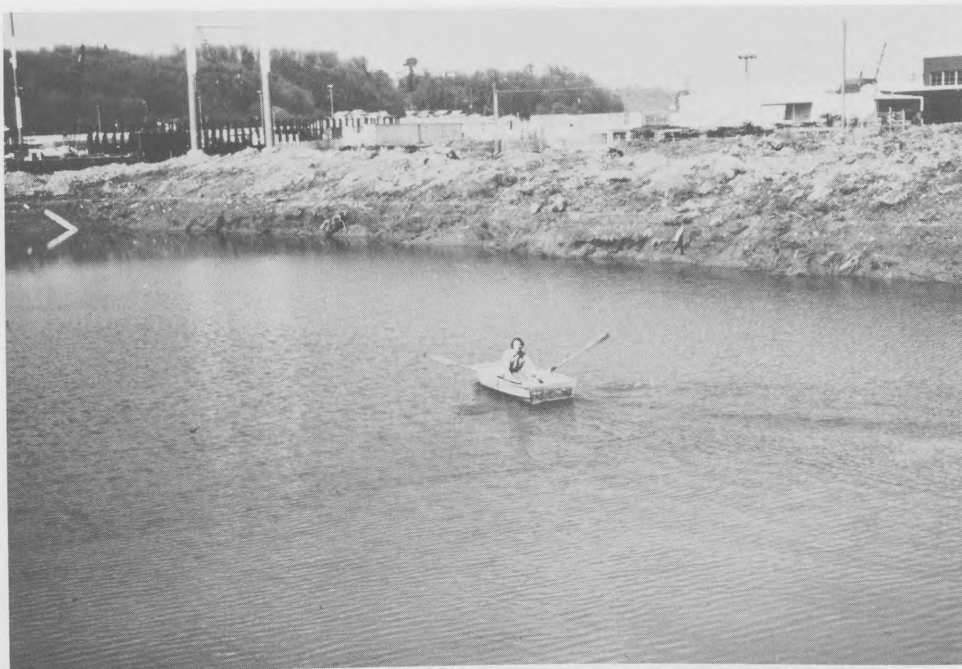
Photo 15. Seattle, Wash., disposal area; clear water in compartment 1 resulting from inhibition of iron hydroxide precipitation by highly reduced dredged material on bottom
