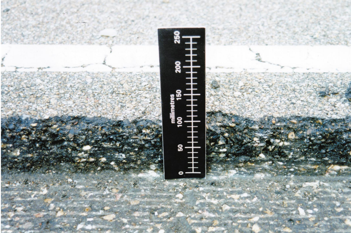
Figure 40. Milling depth on USAEWES whitetopping test section
