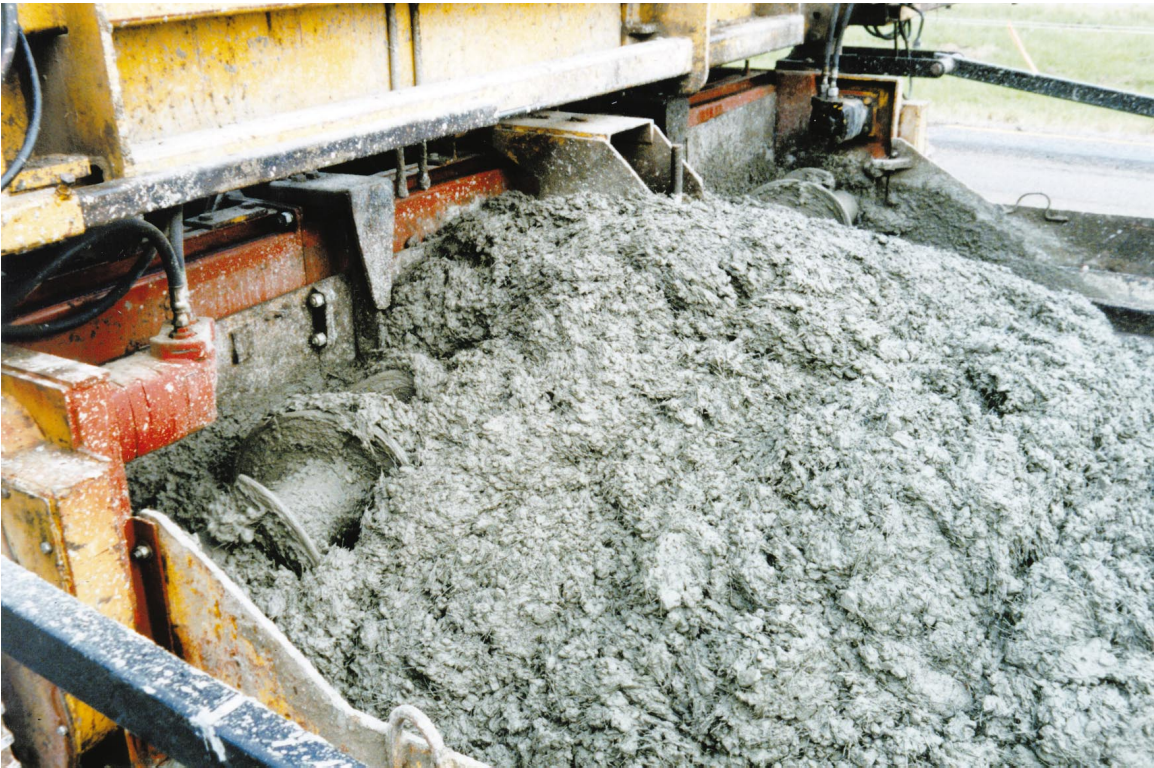
Figure 42. FRC entering slip-form paving machine on USAEWES whitetopping test section
