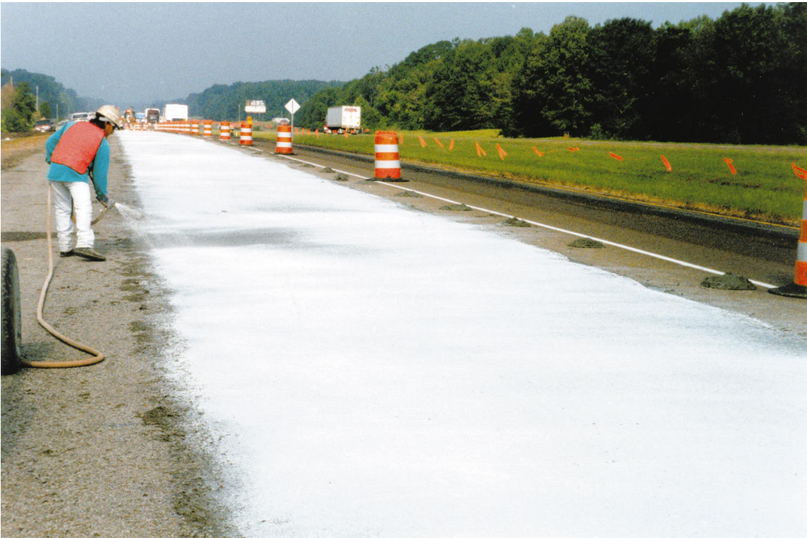
Figure 46. Application of curing compound on USAEWES whitetopping test section
