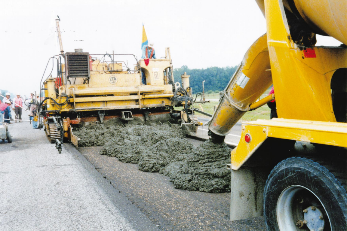
Figure 41. FRC discharged in front of slipform paving machine on USAEWES whitetopping test section
