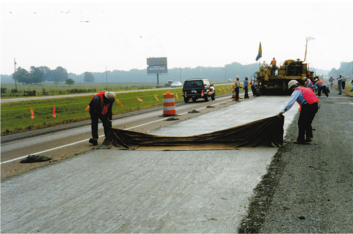
Figure 45. Burlap drag finish on USAEWES whitetopping test section
