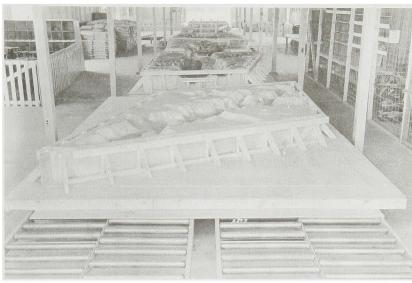
prepared subgrade using the traditional template method. This involved cutting sheetmetal templates to cross sections obtained from topographic maps and set about 2 ft apart to the correct elevation on the model site in positions located by a
