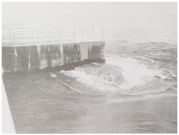
South wing wall, Old River Low Sill Control Structure, prior to collapse in 1973 flood
