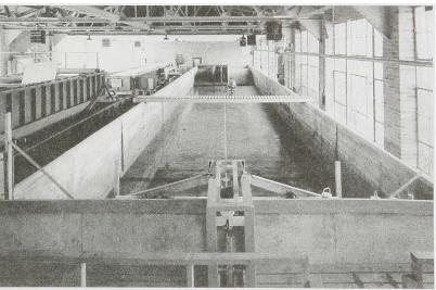
Large flume for breakwater tests
