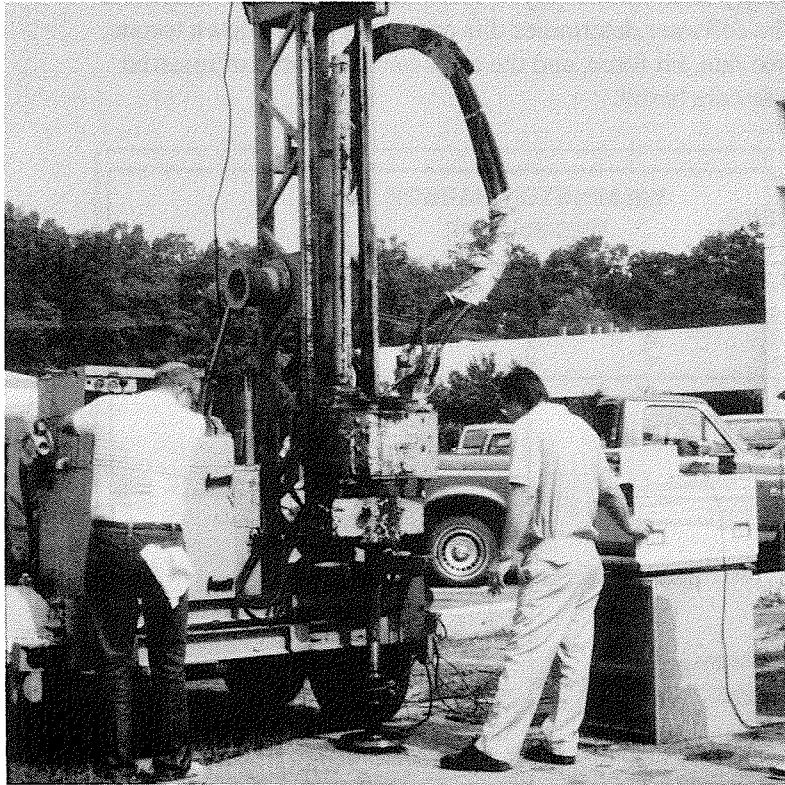
Figure 8. Setup to obtain actual calibration of torque from DPR pressures using torque cell and reaction disk
