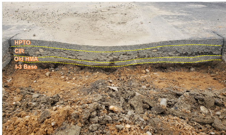
Figure 44. Example of pavement trench cut at position 1 in CIR3%FAC section.
