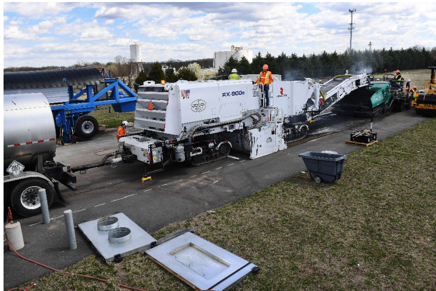
Figure 1. Cold in-place recycling equipment.
