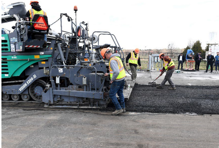
Figure 3. CIR mix placement.
