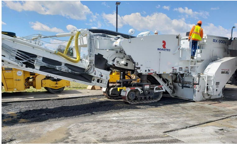
Figure 2. CIR milling process.
