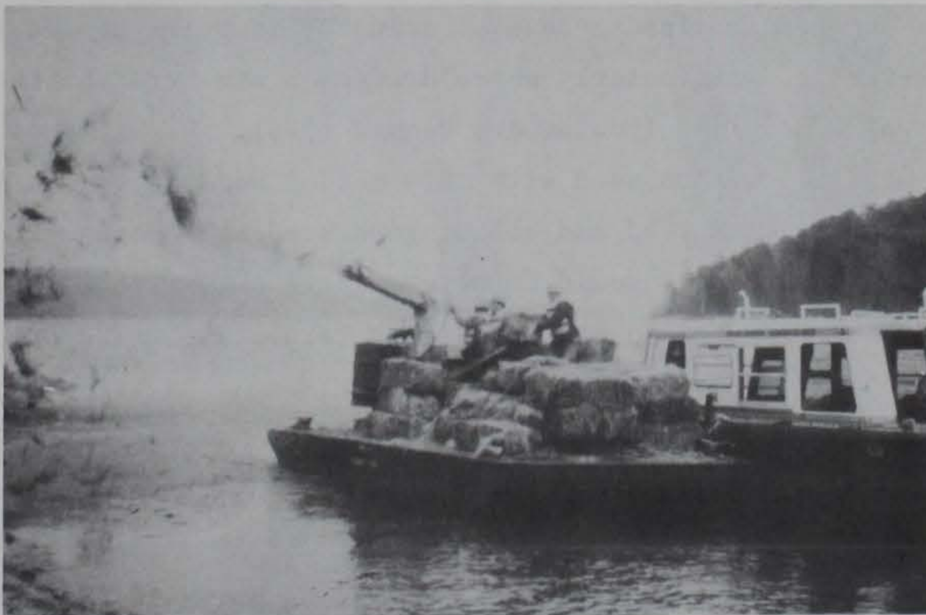
Figure 13. Hydroseeding shorelines from a barge, Lake Ouachita, Arkansas
