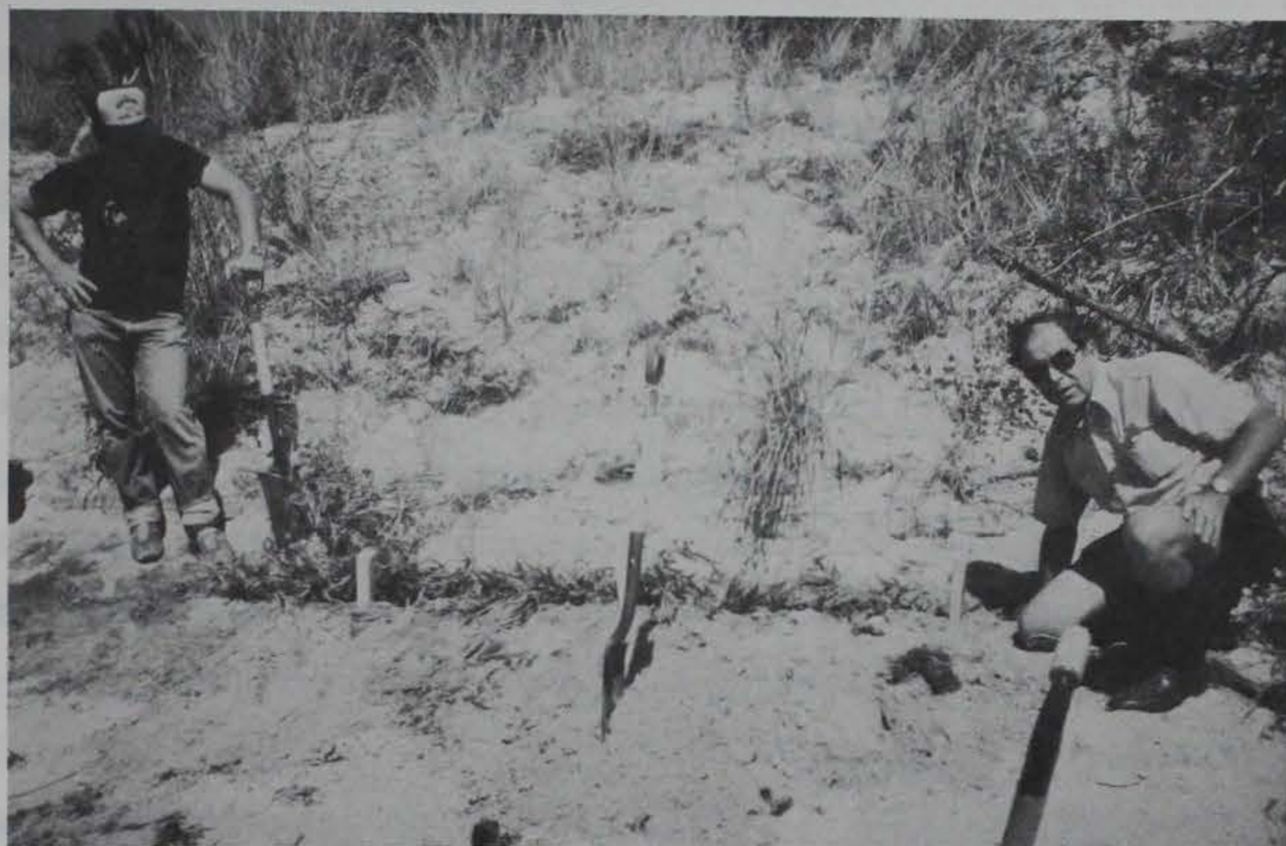
Figure 28. Completed wattling installation
