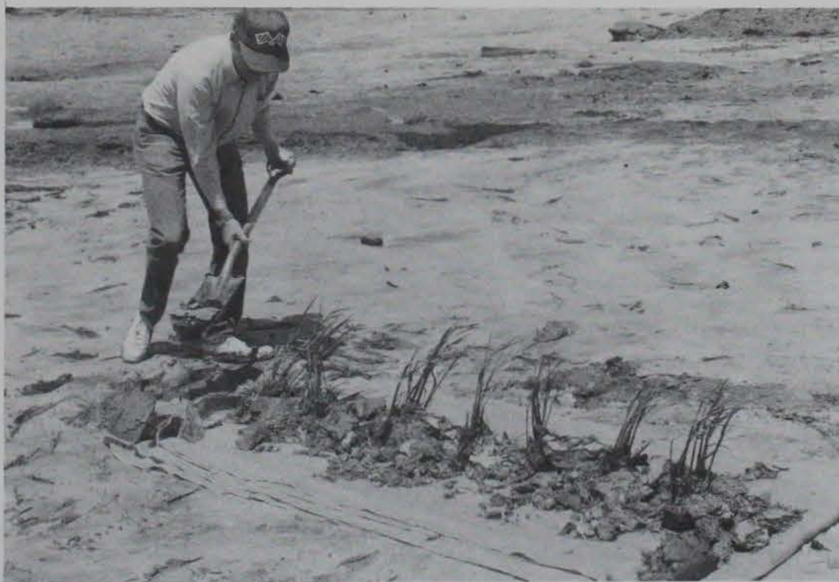
b. Clumps placed on burlap at intervals, along with soil and fertilizer
