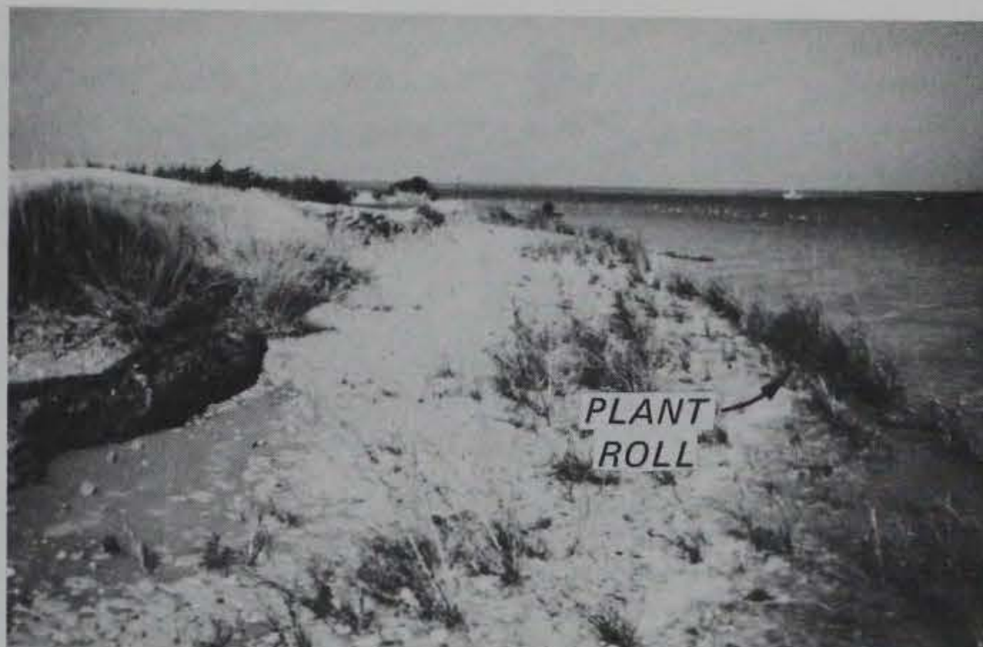
e. Plant roll installed parallel to shoreline
