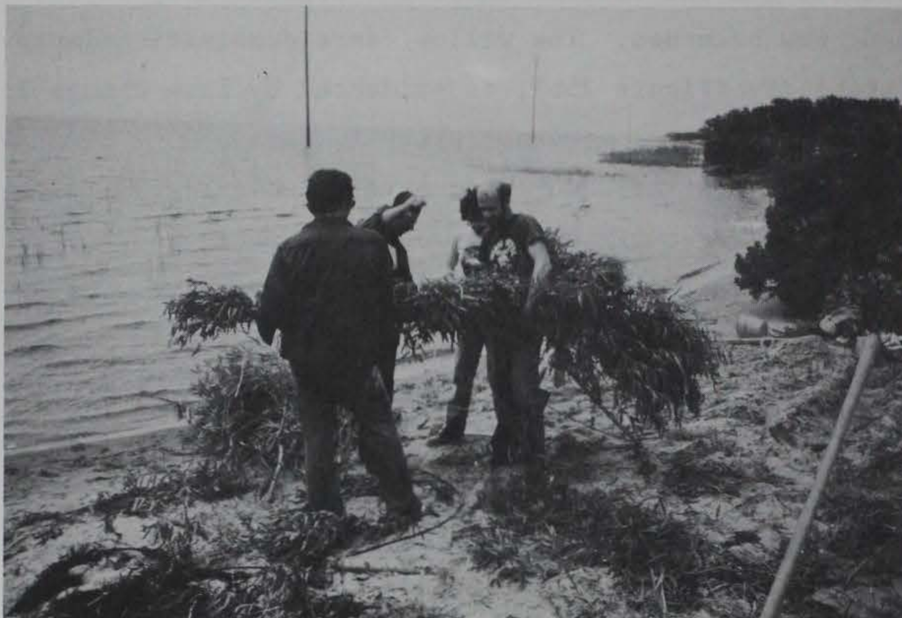
Figure 26. Assembly of a wattling bundle
