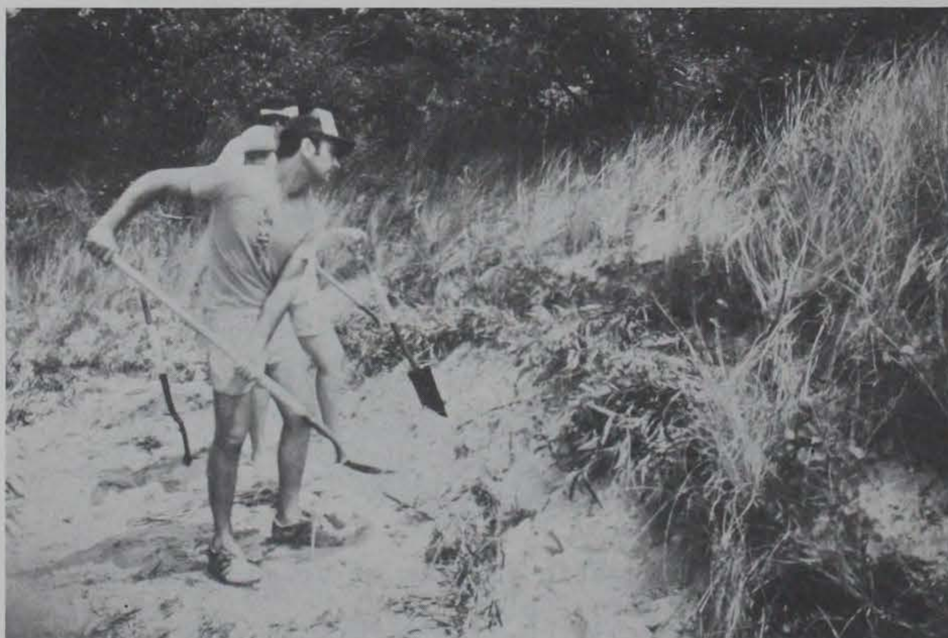
Figure 30. Installed section of brush layering
