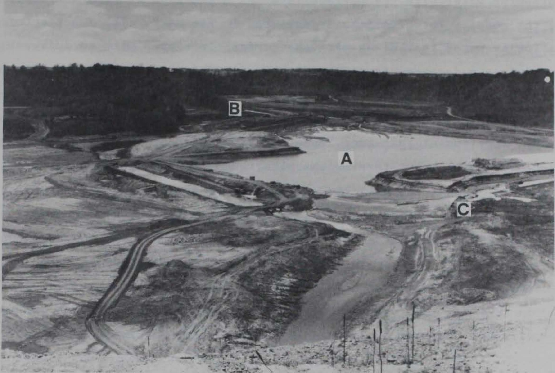
Figure 7. Eau Galle Reservoir, 3 months before dam completion (A is located in the borrow pit, B is located at the inflow of the Eau Galle River, and C is located at the inflow of Lohn and Lousy Creeks)
