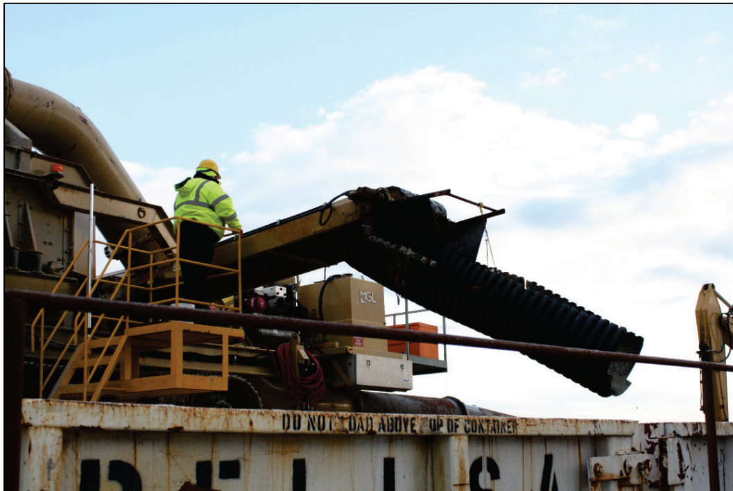
Figure 19. FRS unit modified for use in a beach nourishment project in Deal, NJ, that involved MEC.
