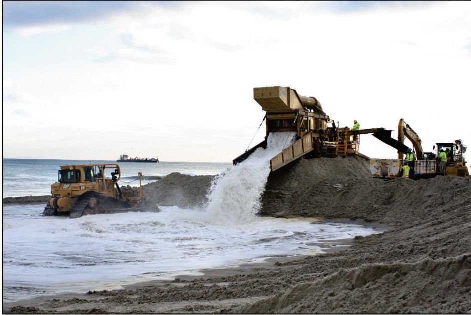
Figure 15. FRS discharge flume depositing undersized material (slurry consisting predominantly of water and sand) onto beach. Note Manson hopper dredge Glenn Edwards in background, pumping ashore.
