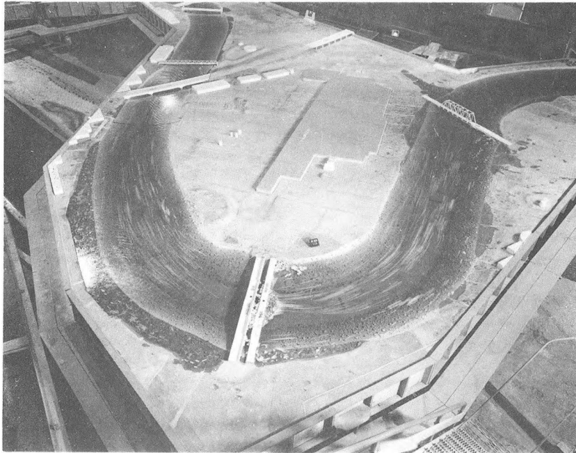
From bridge B-10 to B-8
