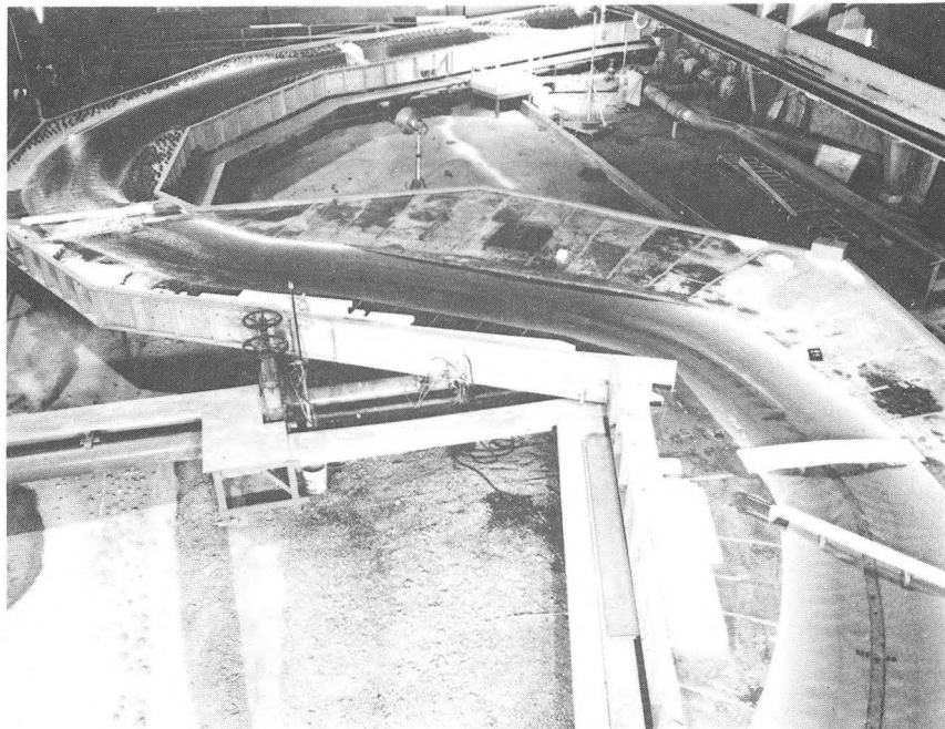
From bridge B-7 to B-5
