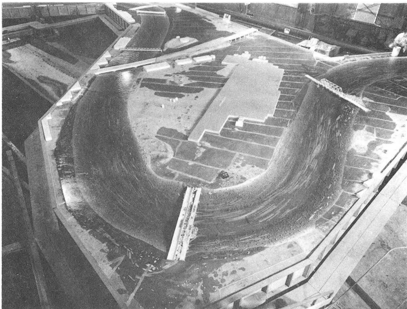
From bridge B-10 to B-8
