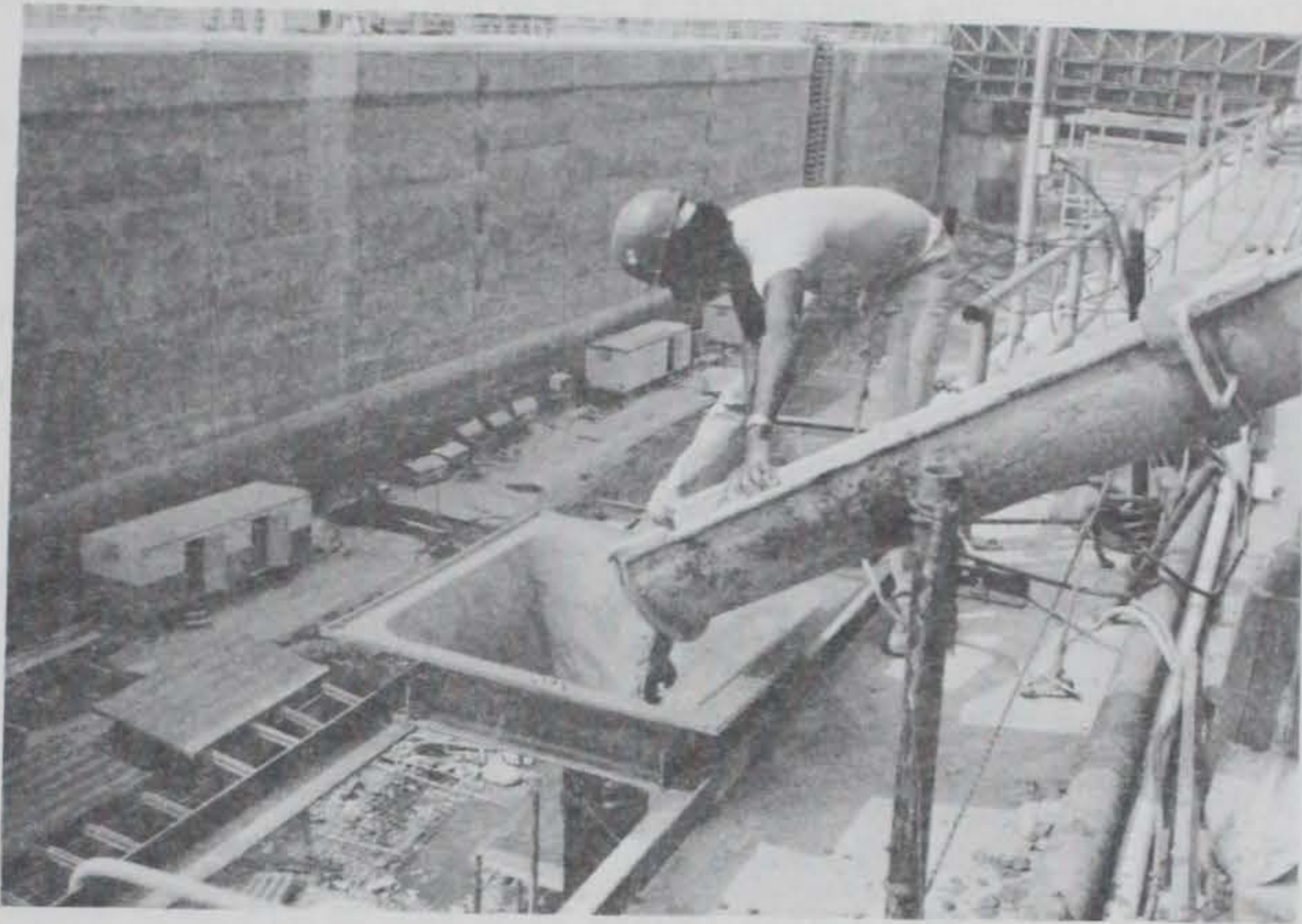
Figure 153. Placing concrete on the landside wall, Lockport Lock
