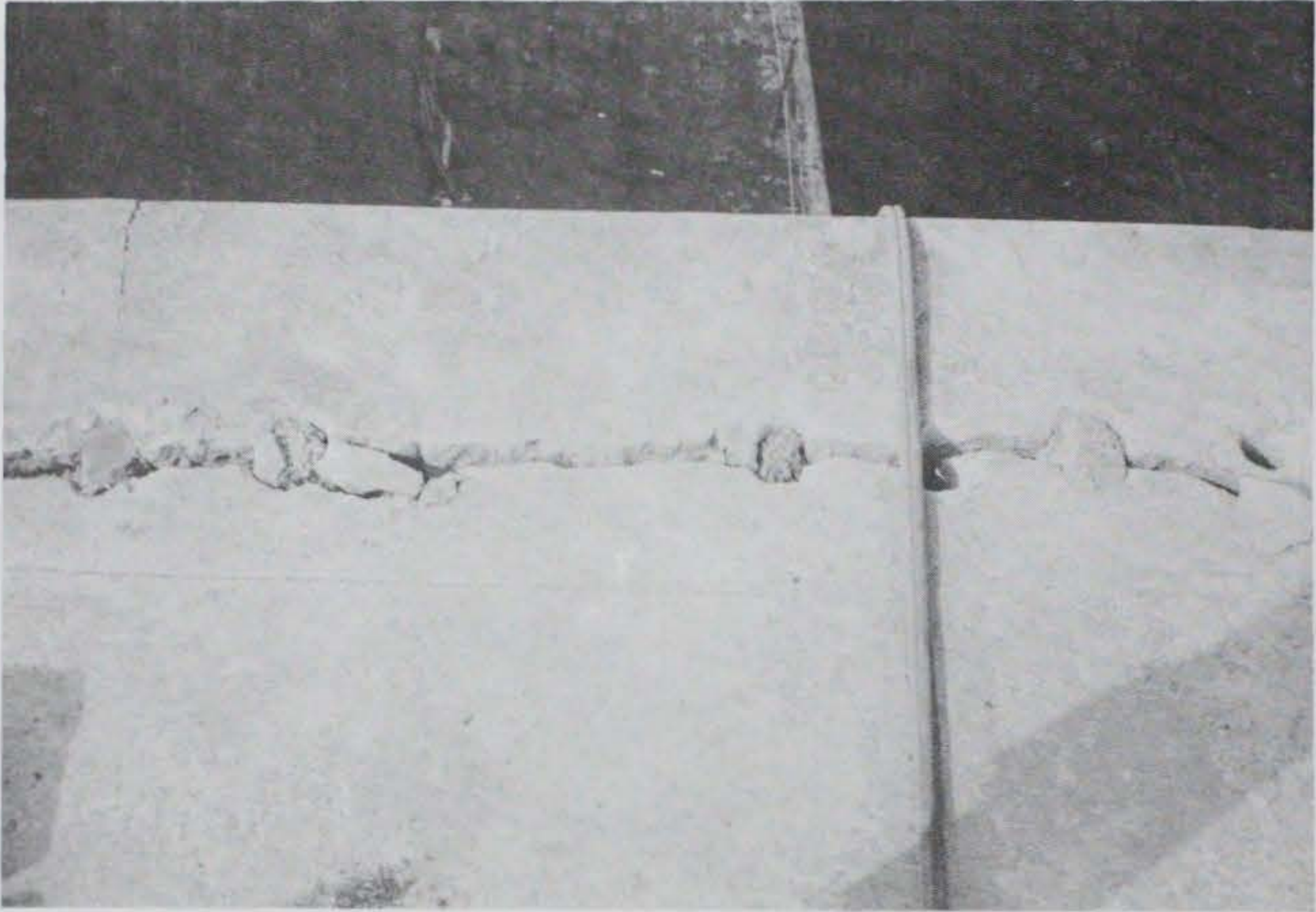
a. Top of lock wall
