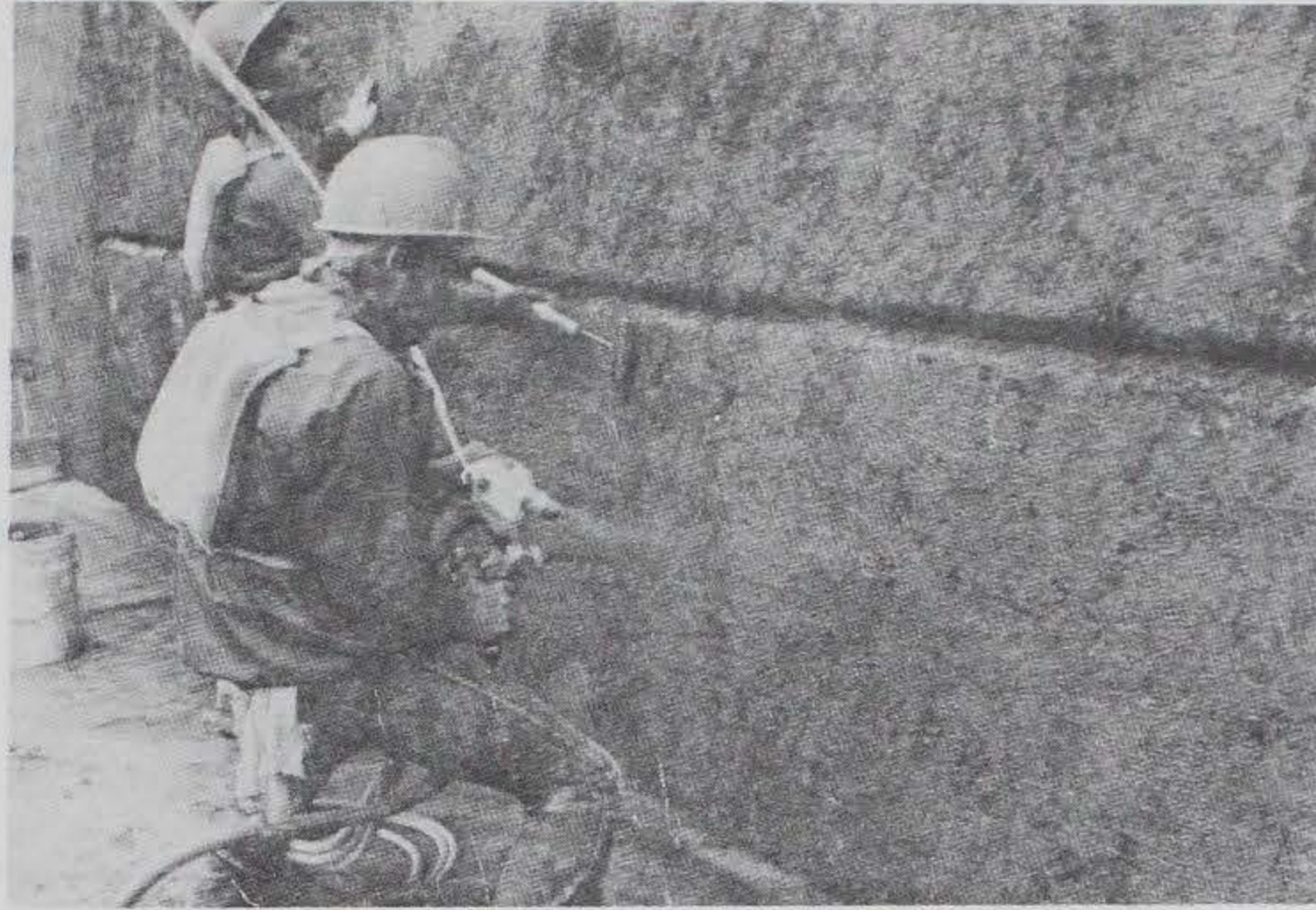
Figure 109. Application of latex-modified, glass fiber-reinforced shotcrete, Lower Monumental Lock
