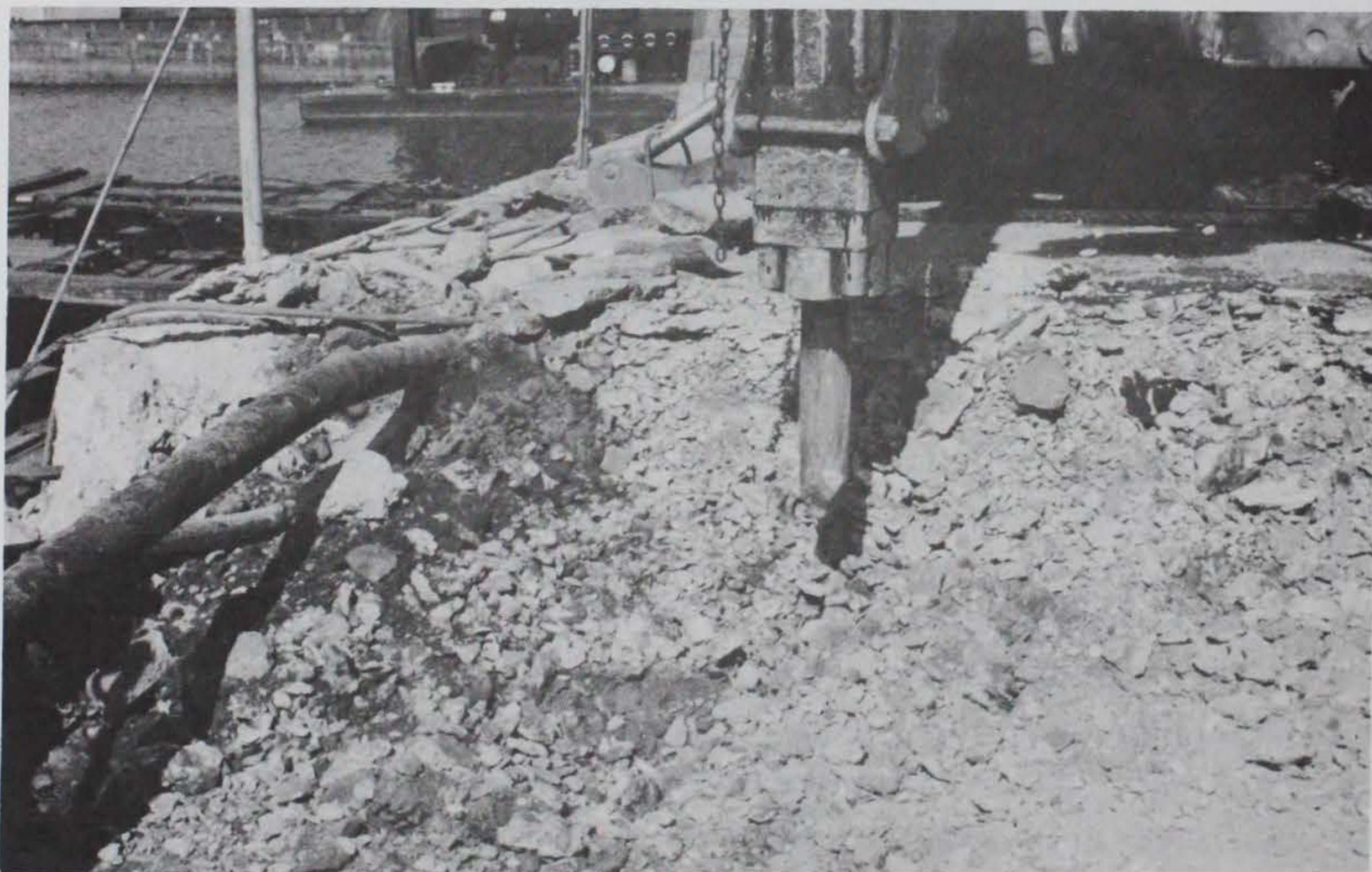
Figure 67. Concrete removal with Hoe Ram Impactor, October 1978, Lock No. 3, Monongahela River
