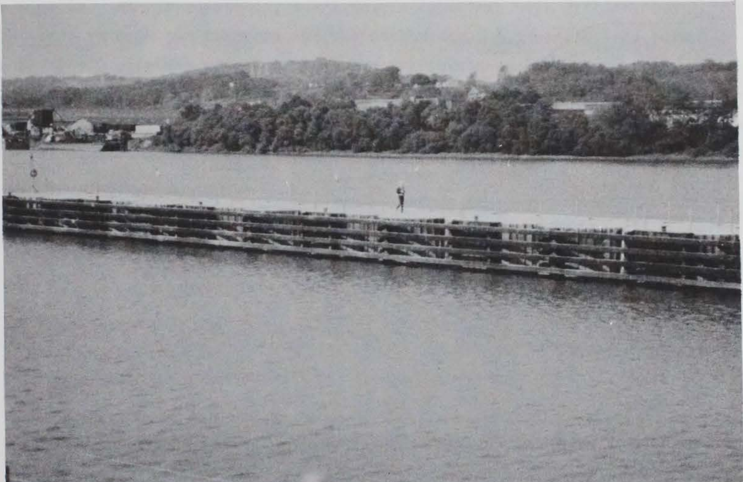
Figure 51. Upper guard wall extension, October 1977, Lock No. 3, Monongahela River
