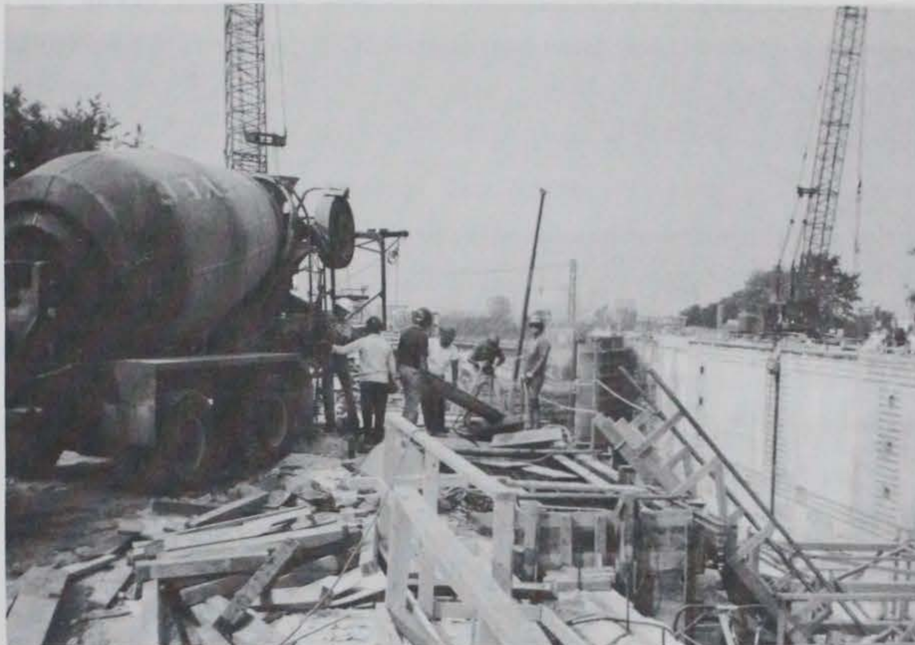
a. Vertical face of lock wall
