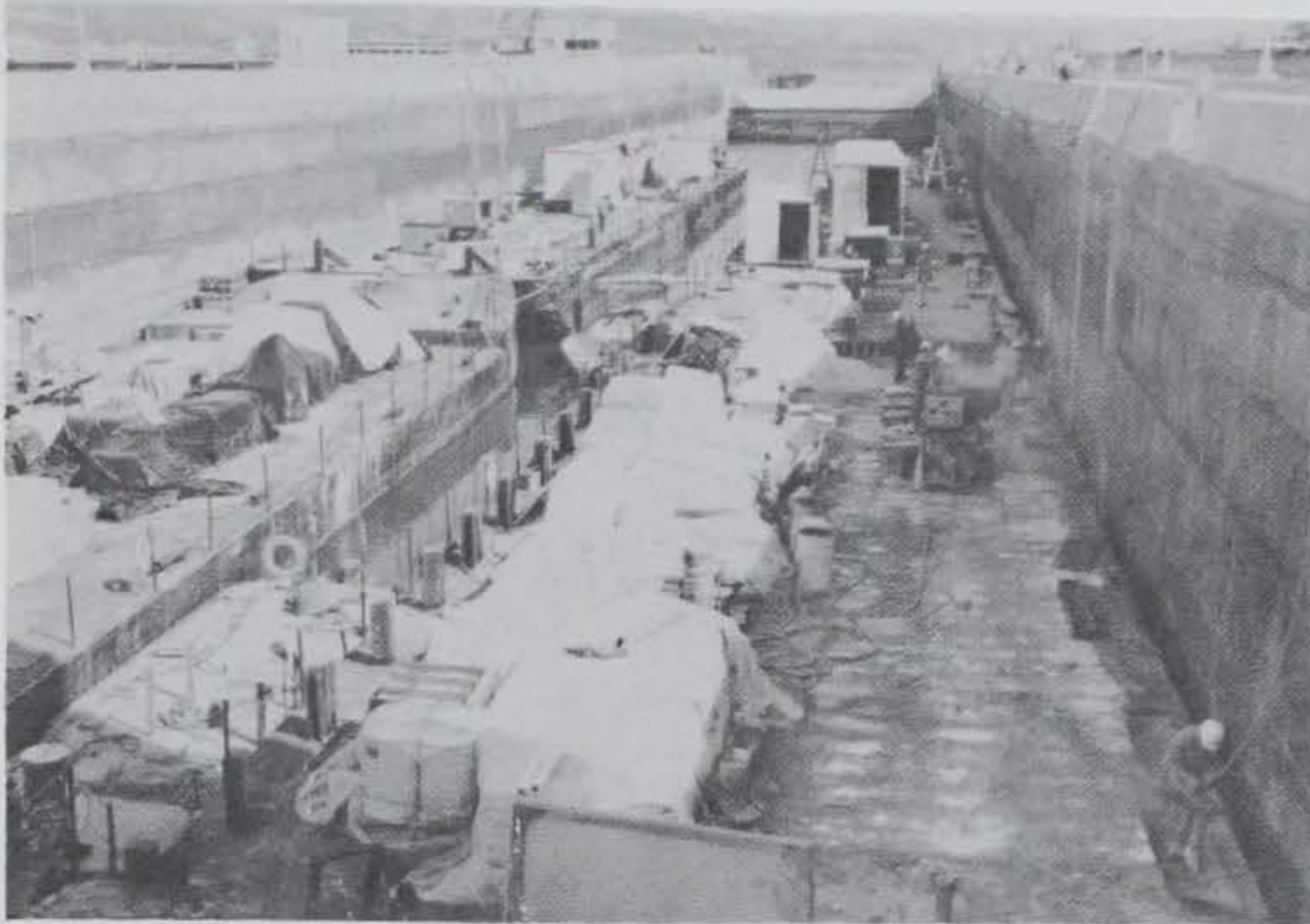
a. Coating application near upper lifts
