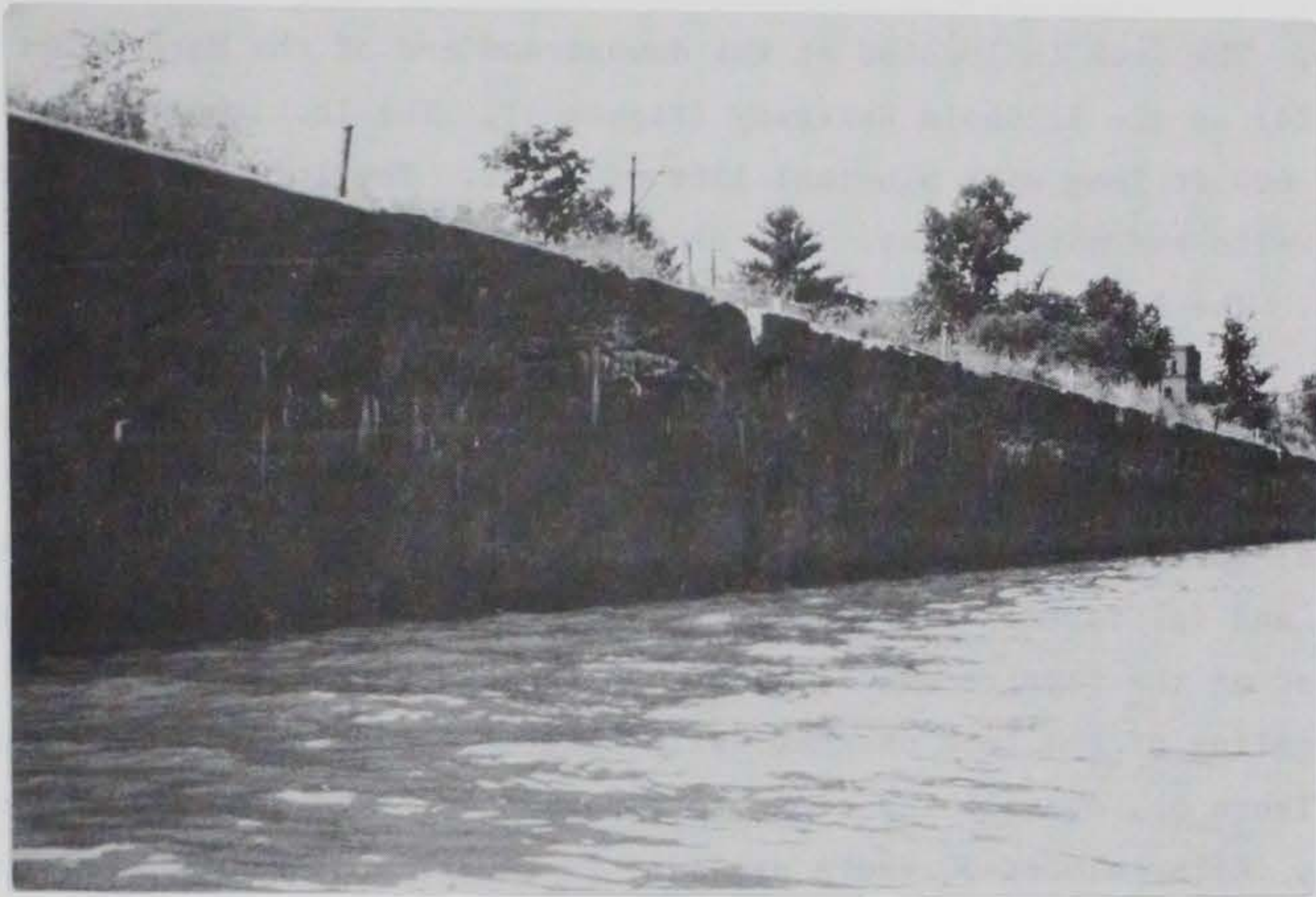
a. Overall view
