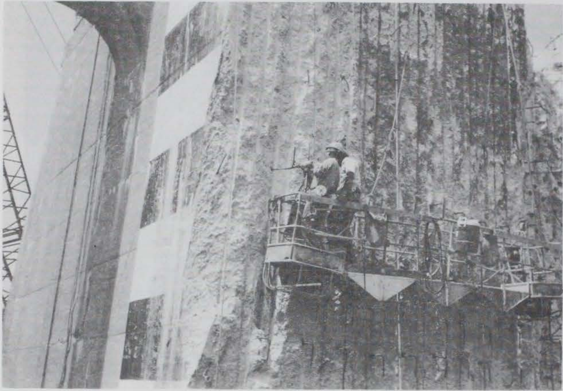
a. Installation of dowels
