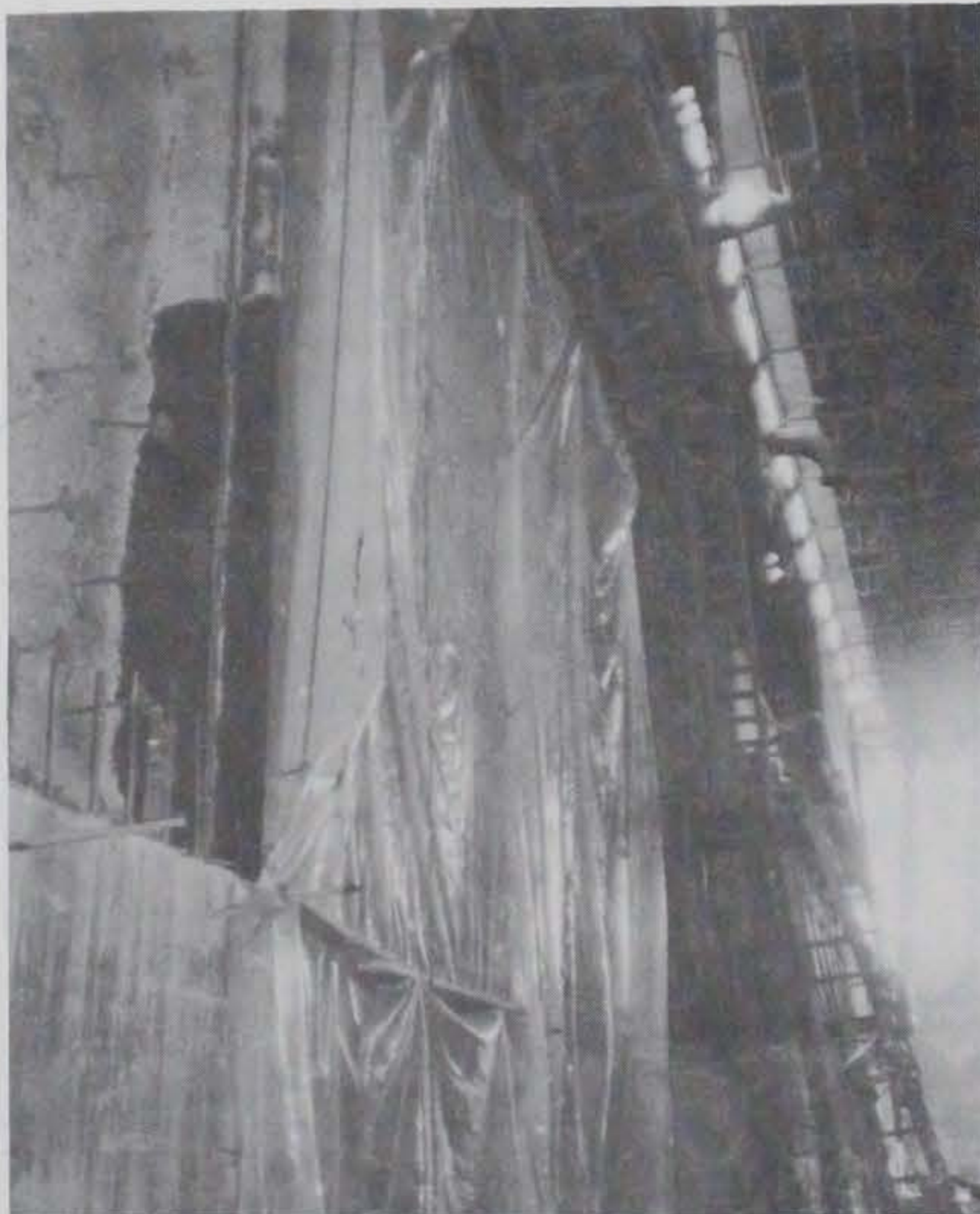
b. Concrete surface covered with polyethylene
