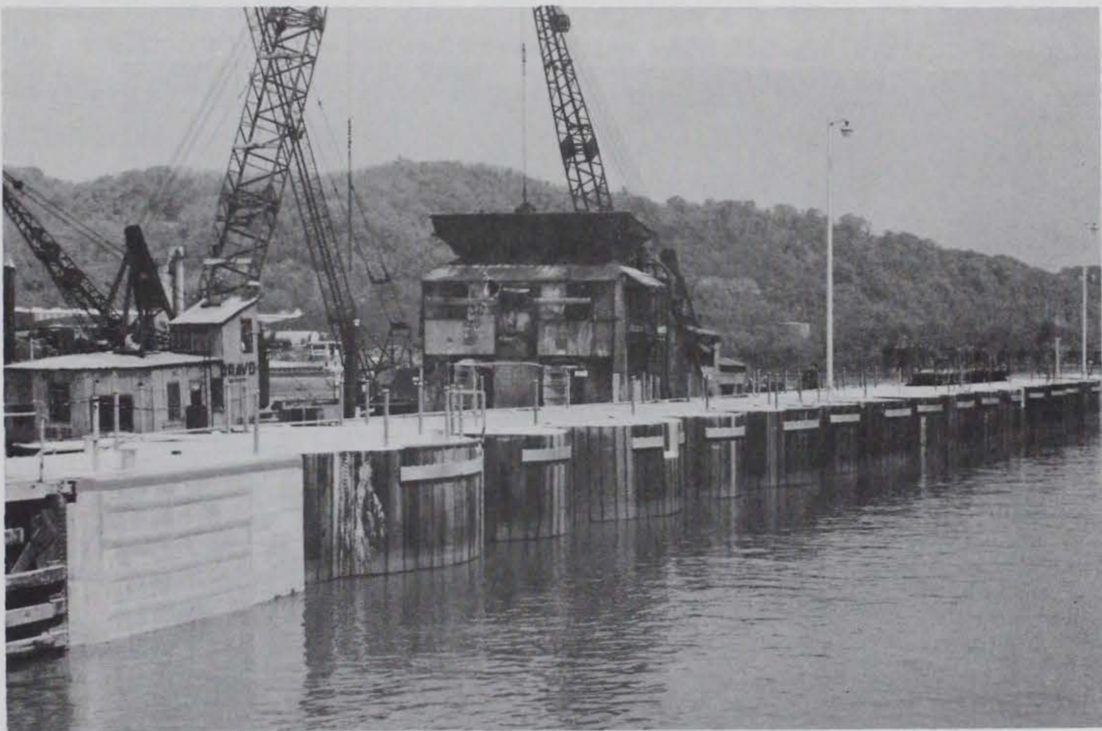
Figure 63. Completed river wall extension, May 1980, Lock No. 3, Monongahela River
