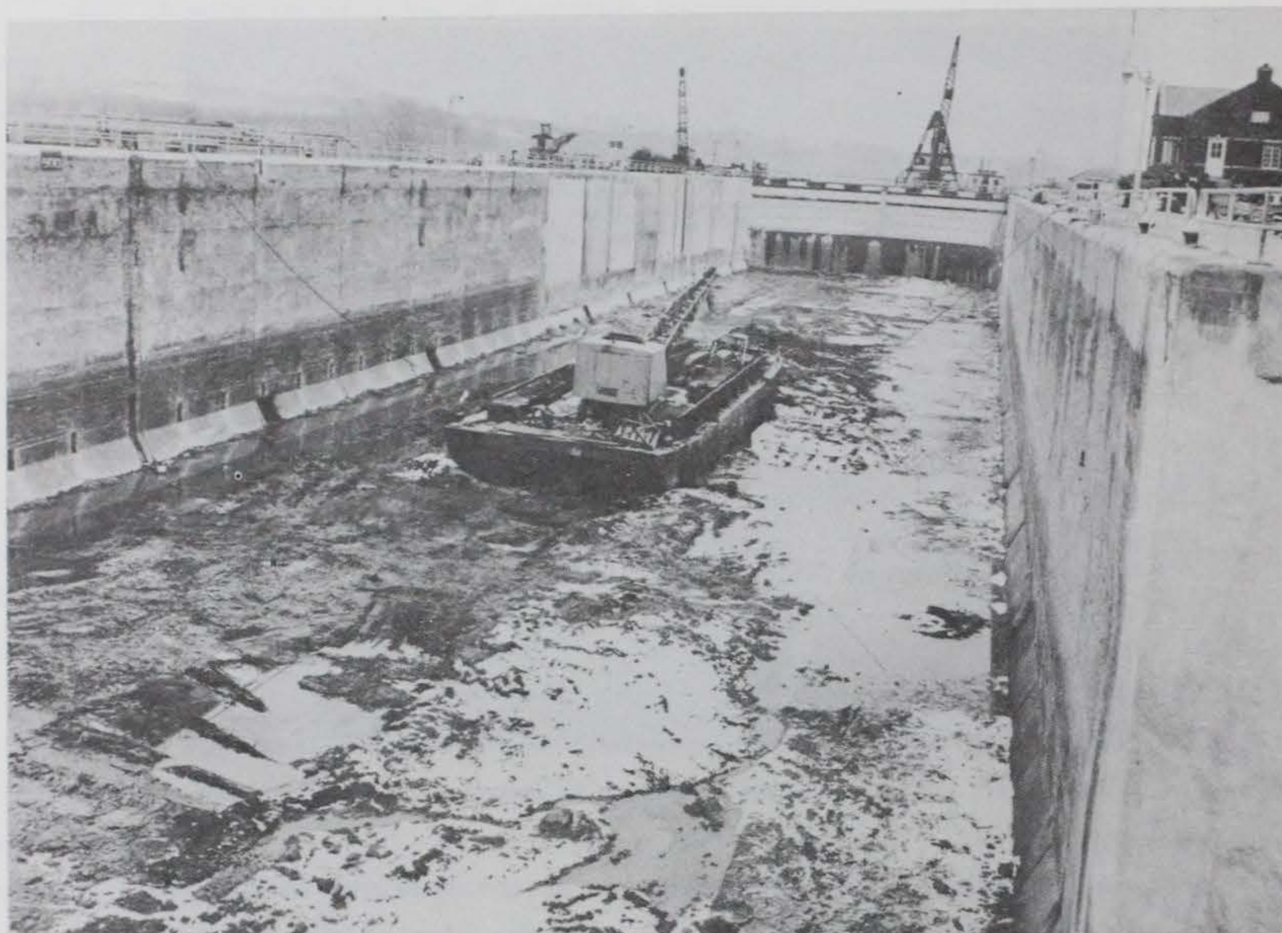
Figure 28. Chamber immediately prior to reflooding after 1954 repairs, Dresden Island Lock
