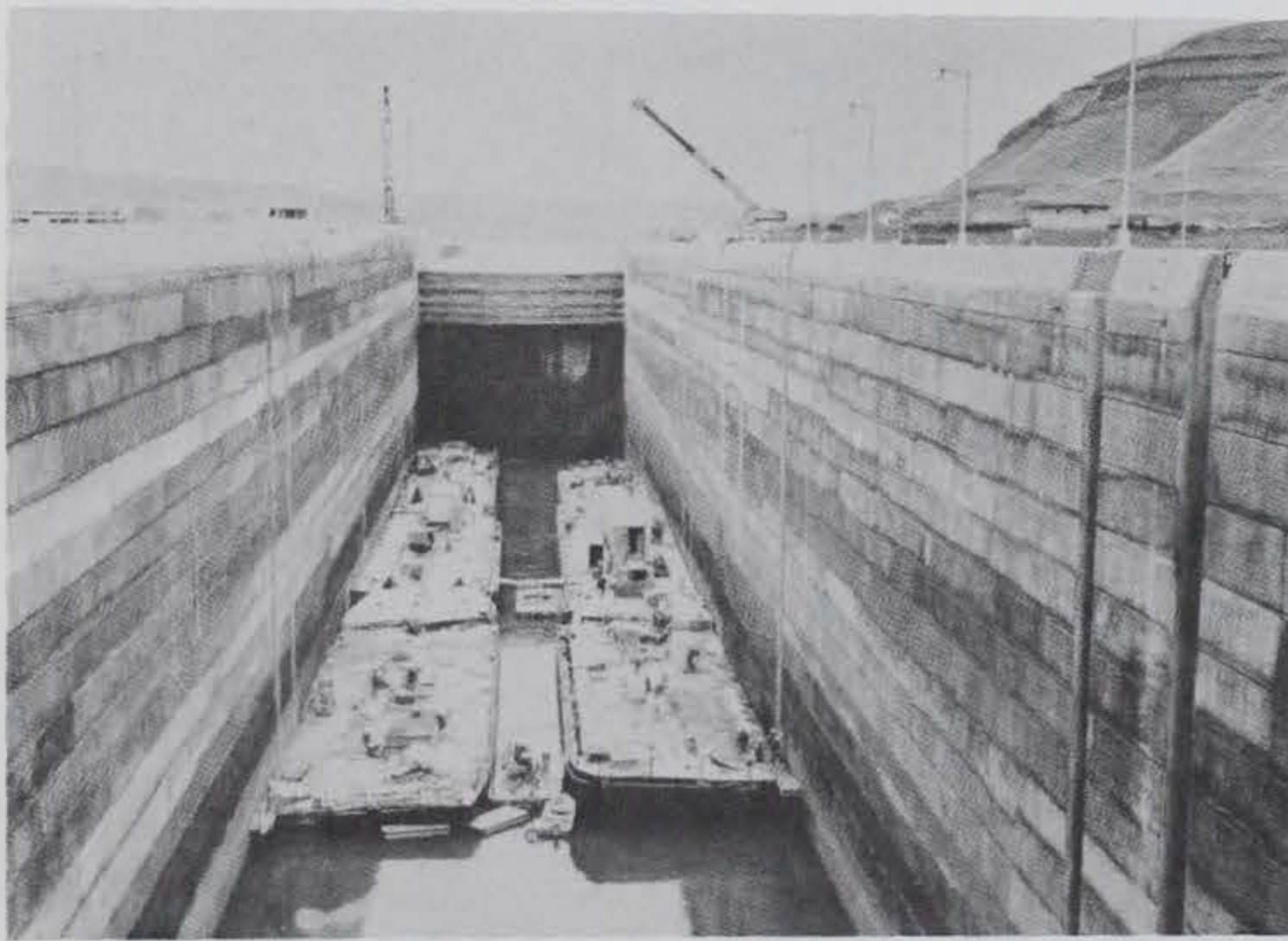
b. Coating application about 75 percent complete
