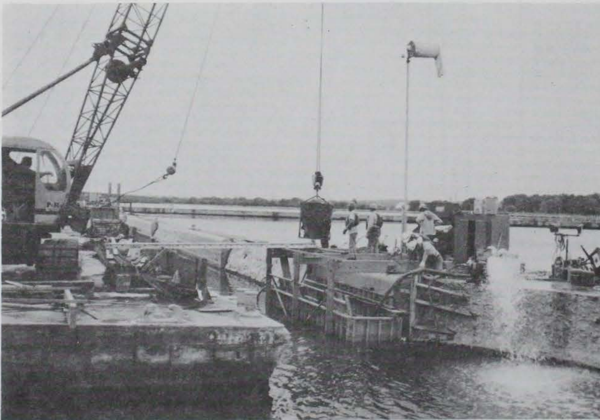
b. Placing concrete
