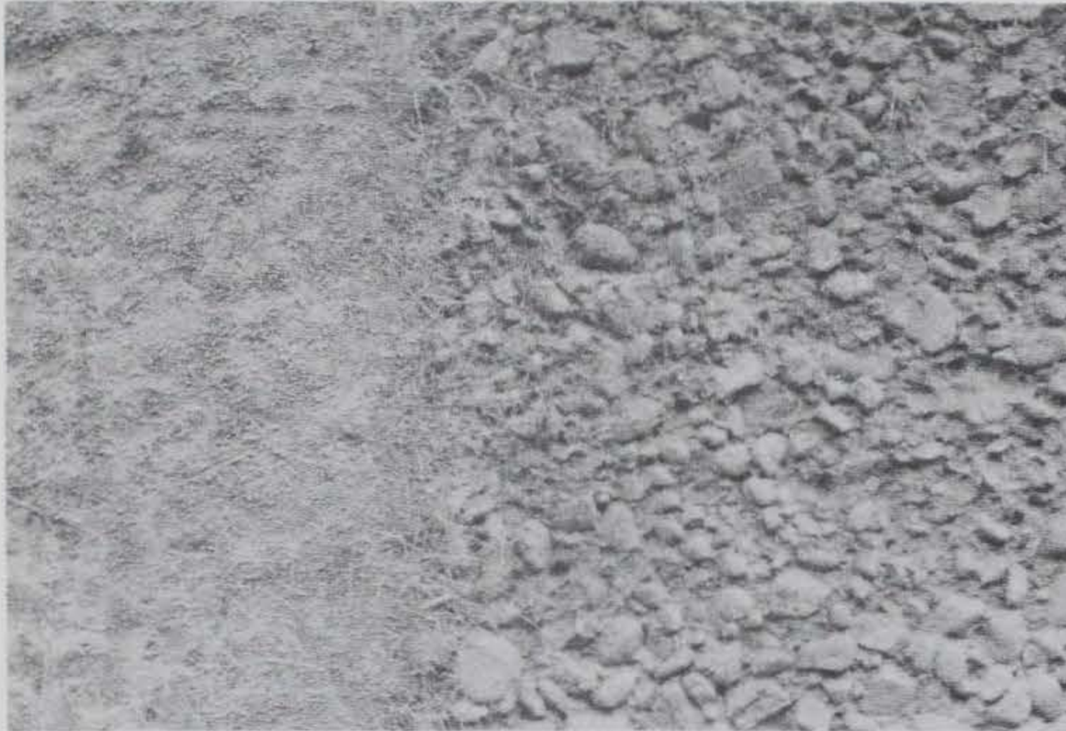
a. Coating of rough, severely deteriorated concrete
