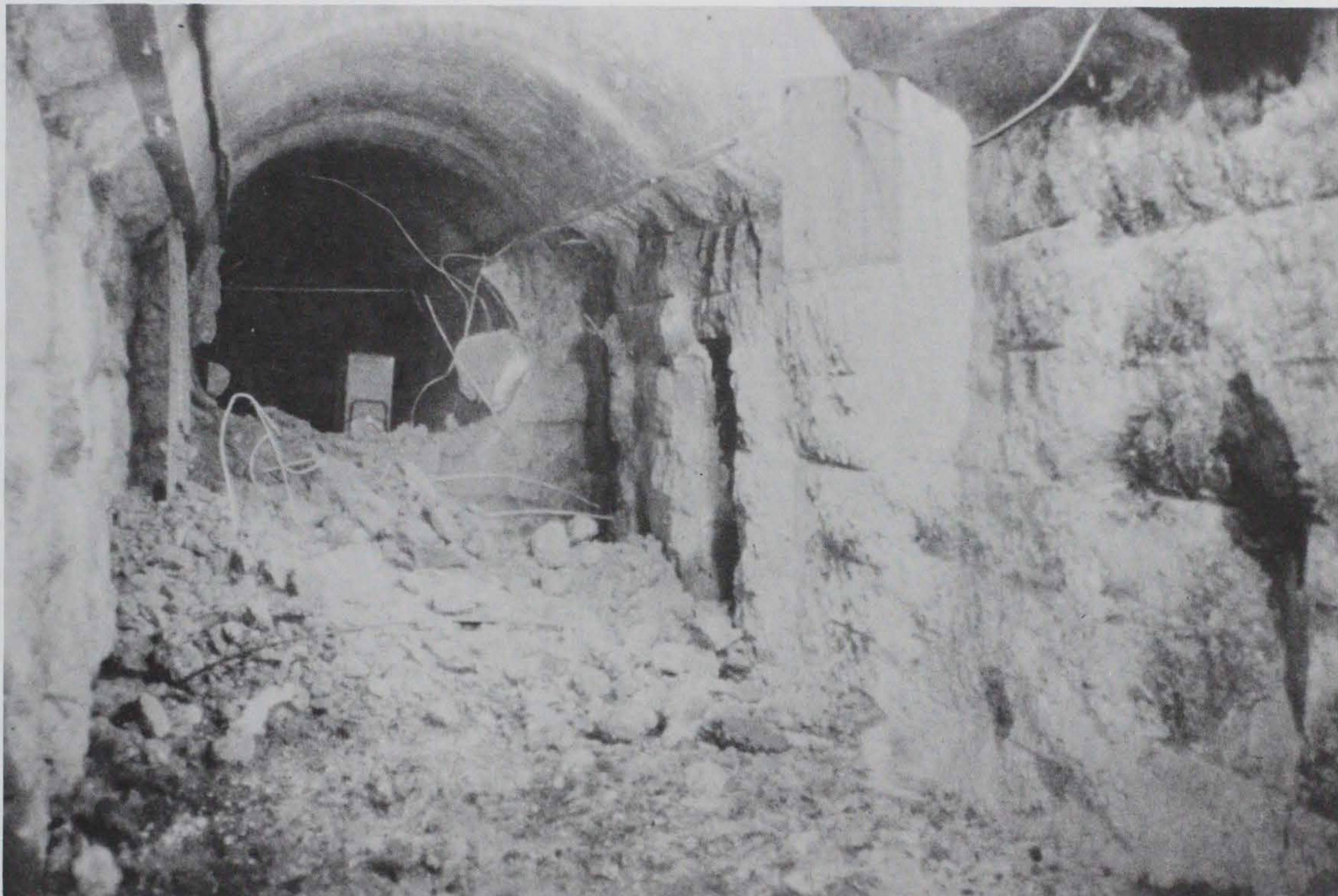
Figure 85. Concrete removal using explosives, Lock No. 1, Mississippi River
