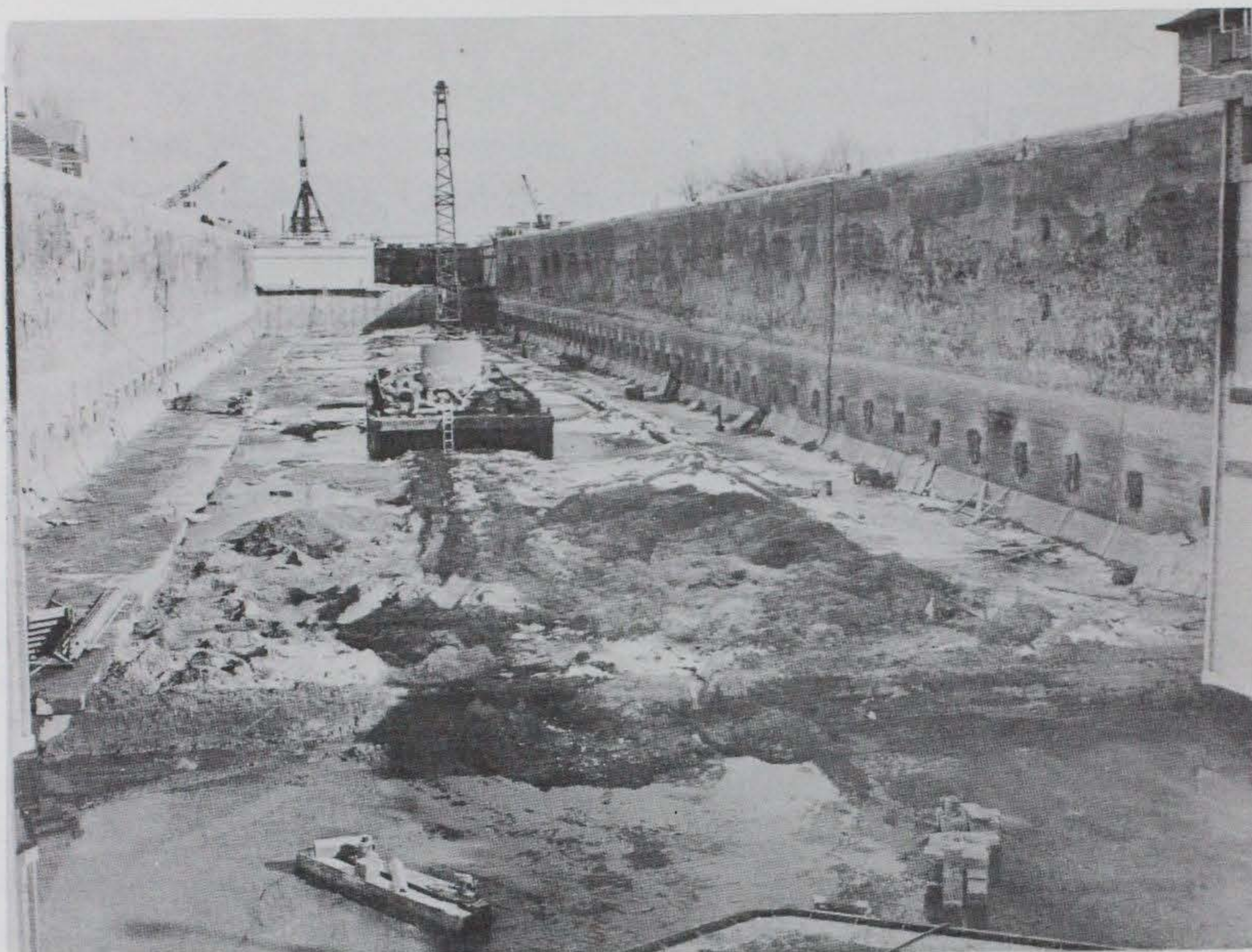
Figure 5. Lock chamber dewatered for repairs, 1952, Marseilles Lock
