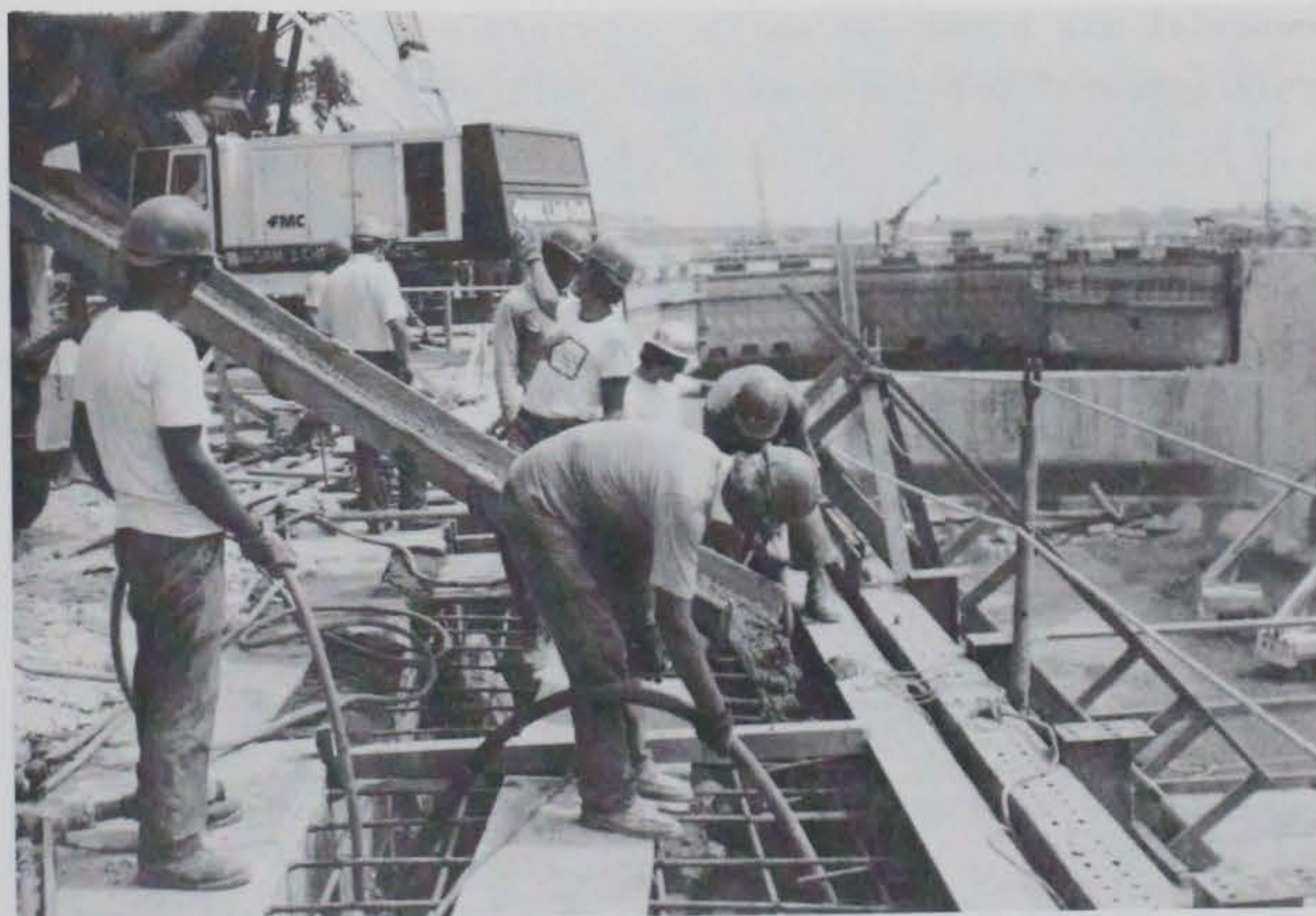
b. Top of lock wall
