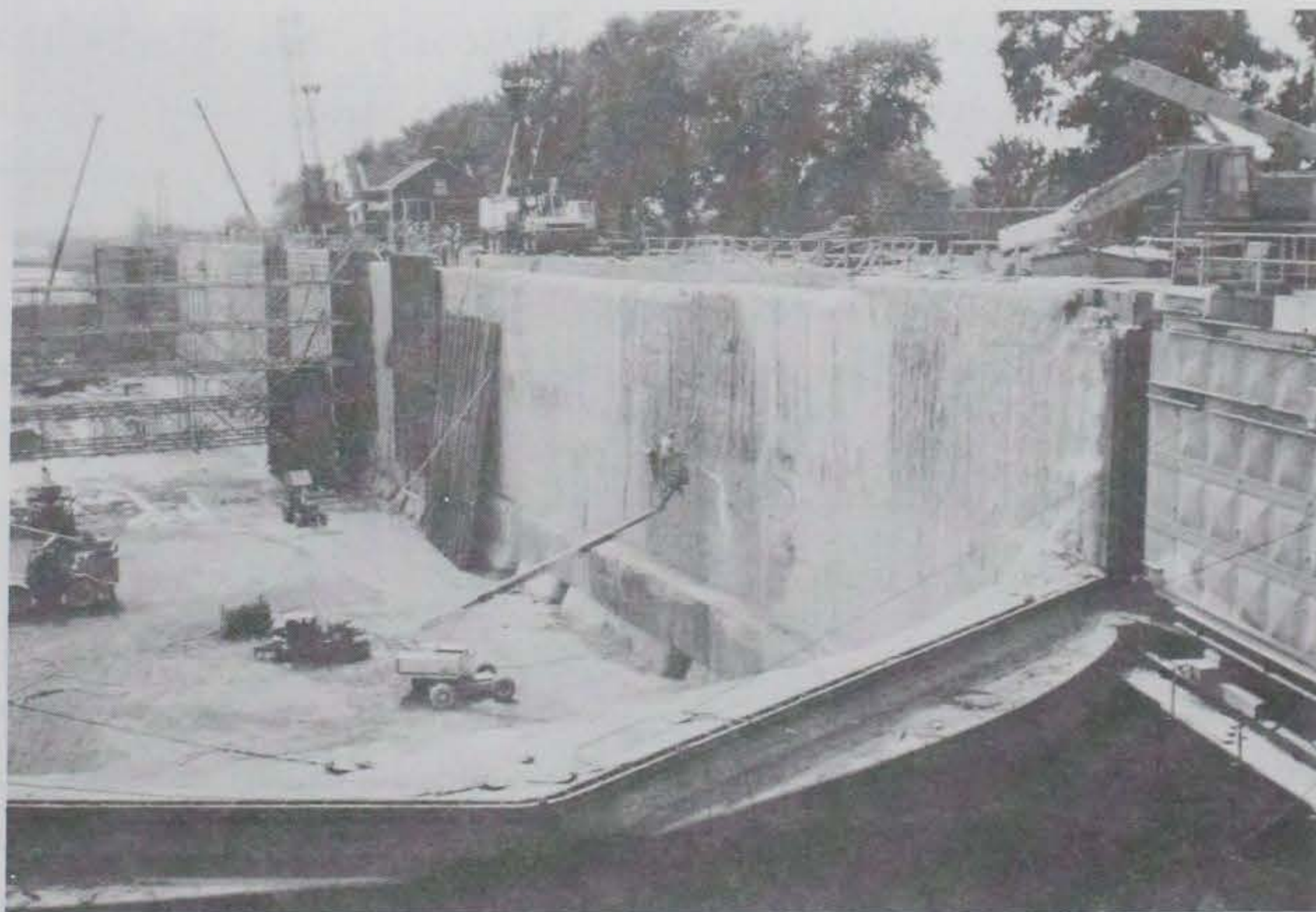
Figure 171. Water blast cleaning of concrete surface, Brandon Road Lock
