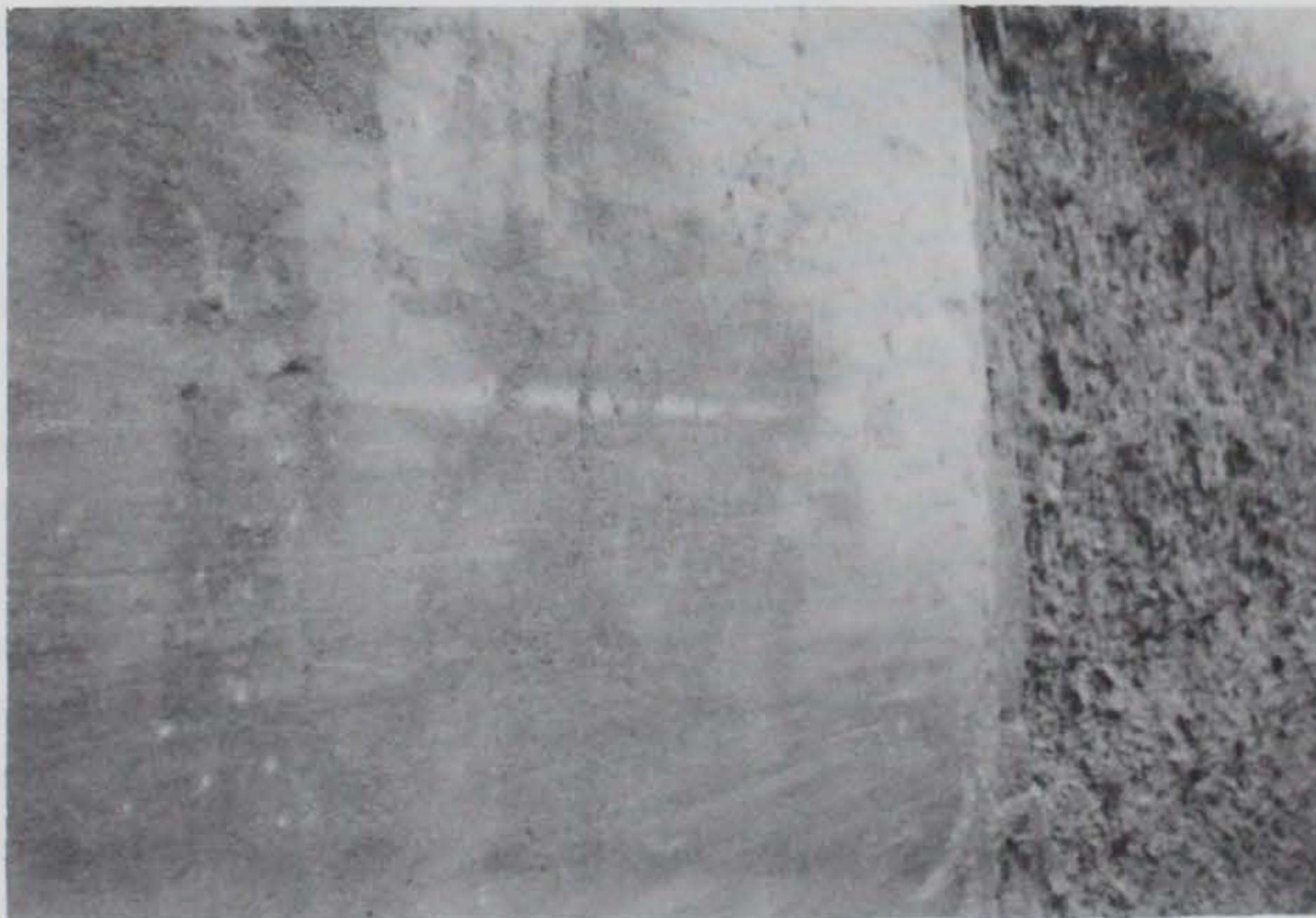
b. Interface between shotcrete (left) and original concrete
