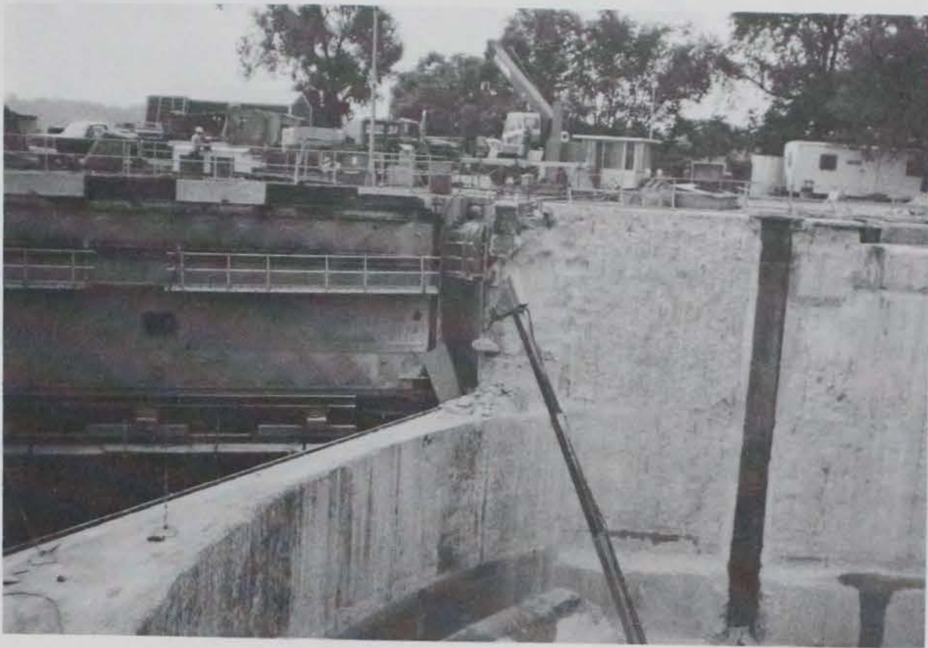
Figure 182. Concrete removal near upper miter gate, Brandon Road Lock
