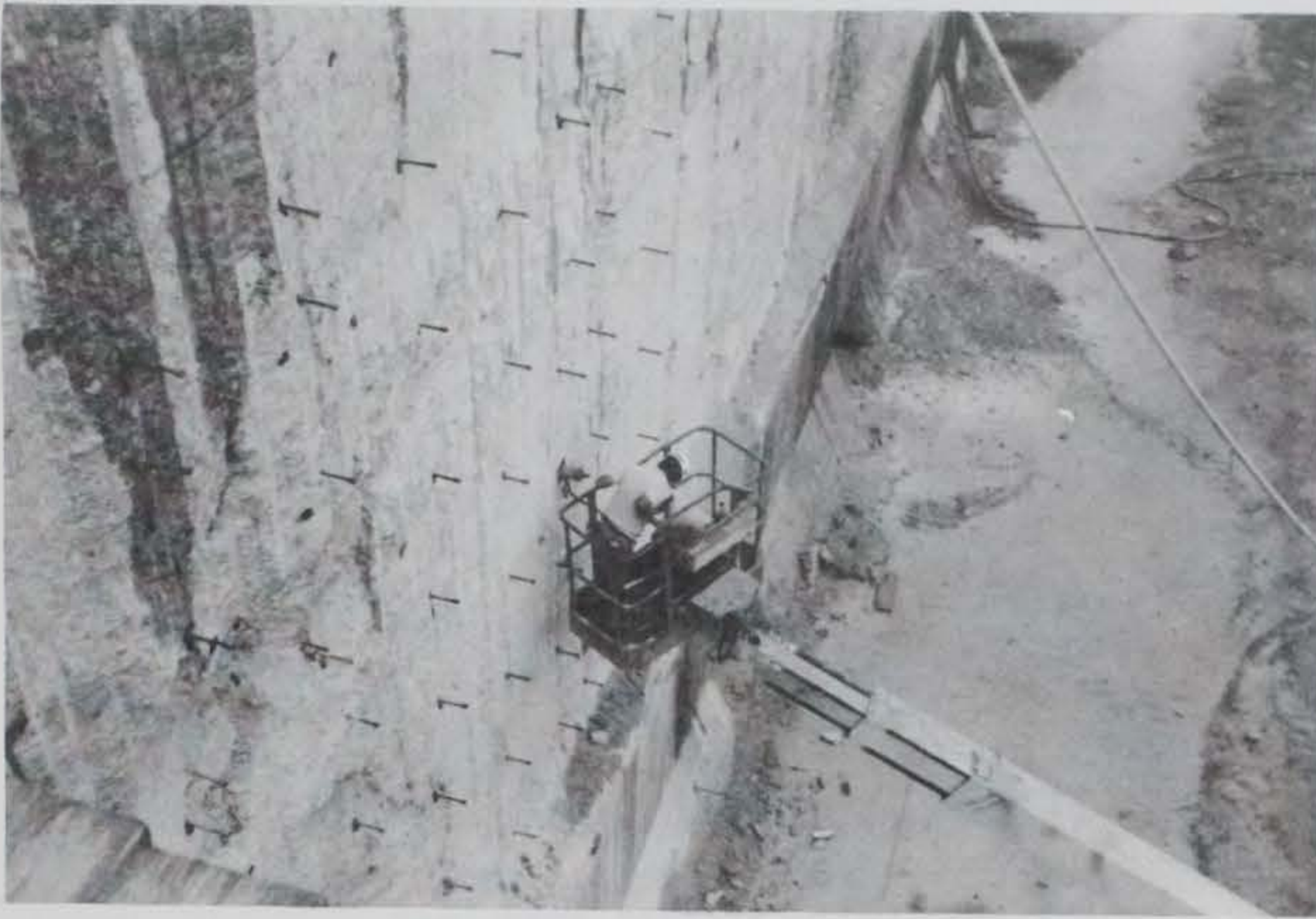
Figure 173. Load testing selected dowels, Brandon Road Lock
