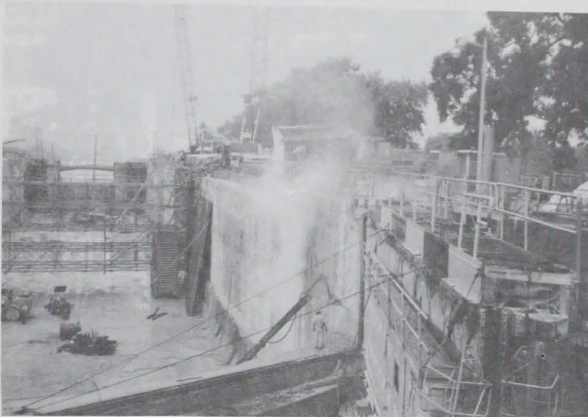
a. Overall view
