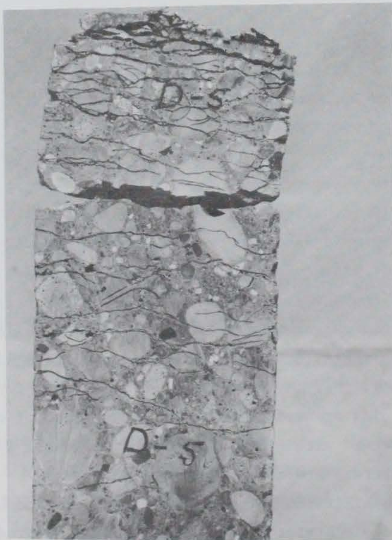
Figure 31. Typical concrete deterioration, 1977, Dresden Island Lock
