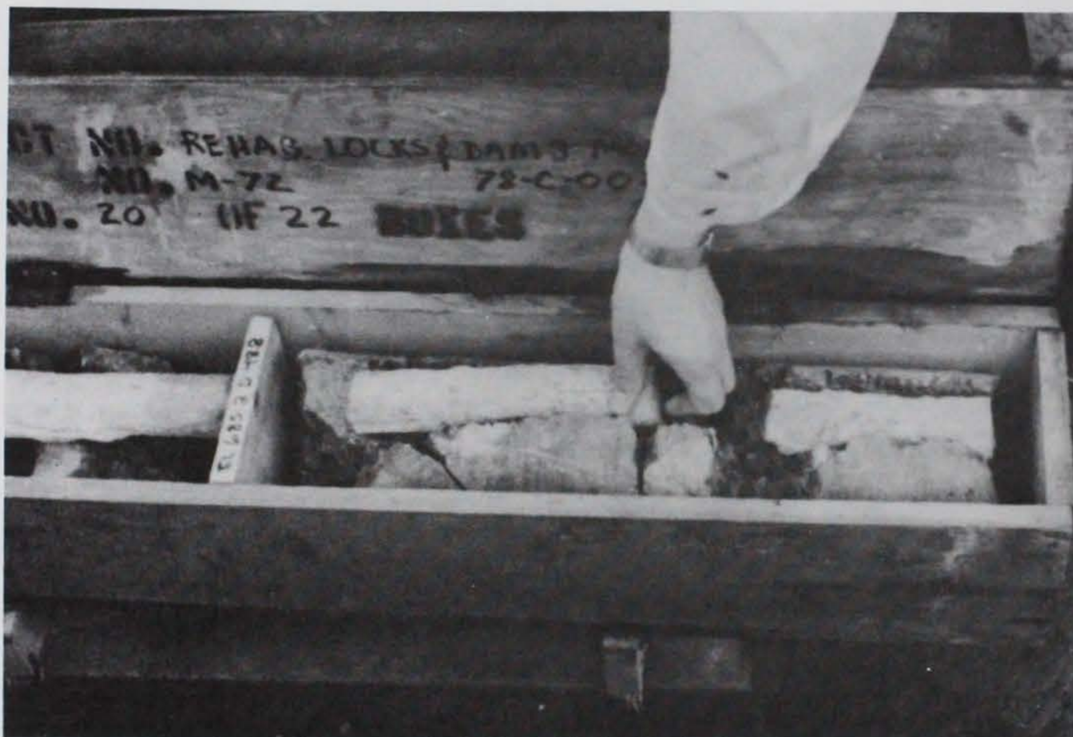
Figure 59. Core from hole where failed anchor was removed, Lock No. 3, Monongahela River
