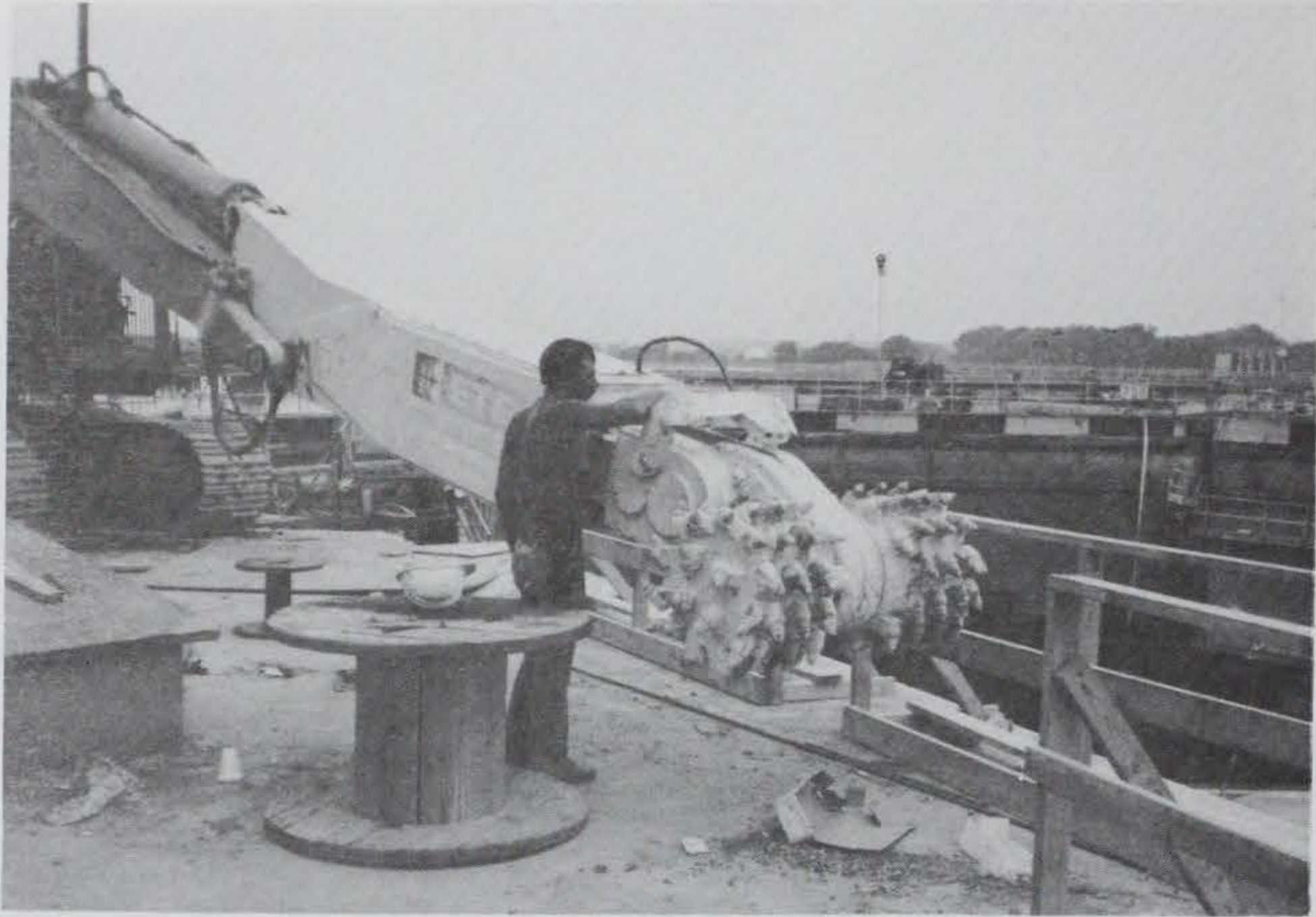
a. Overall view
