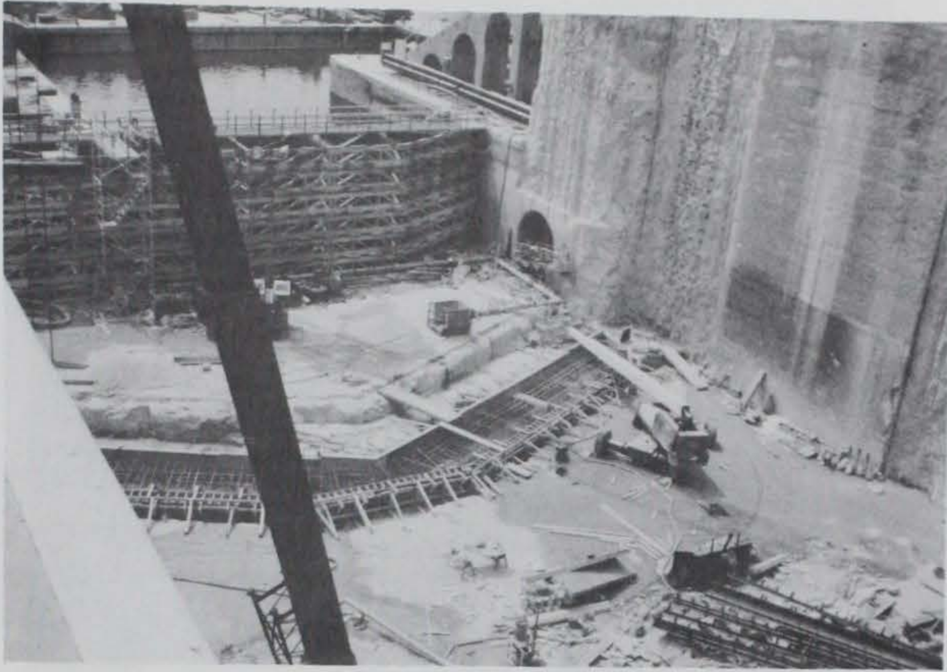
a. Overall view
