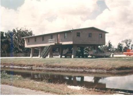
Example of a typical flood proofed structure
