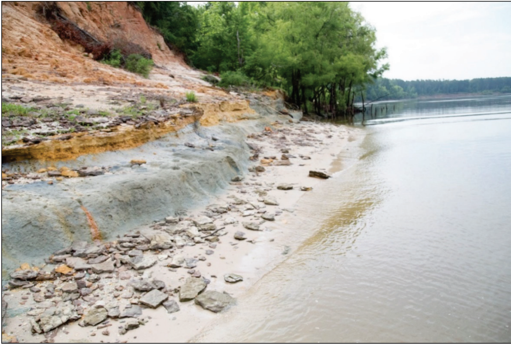
Figure 8. Heavily consolidated silts and clays along the bank of the Tombigbee River.
