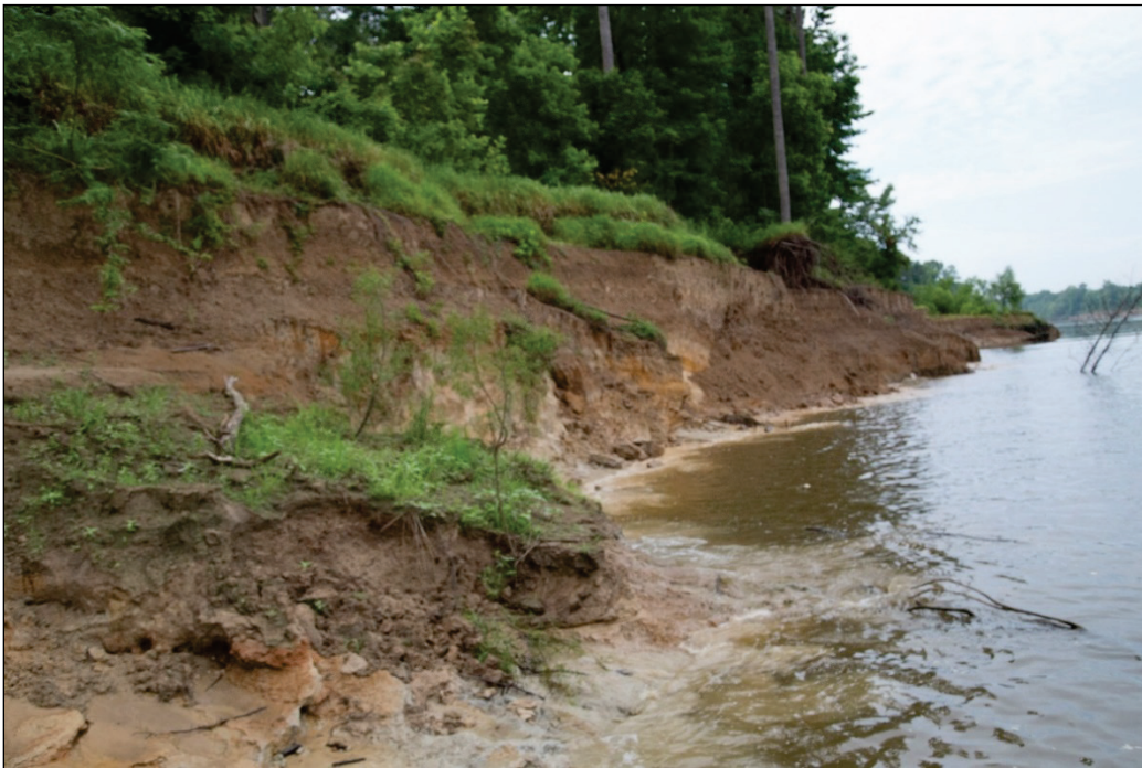
Figure 9. Active bankline erosion
