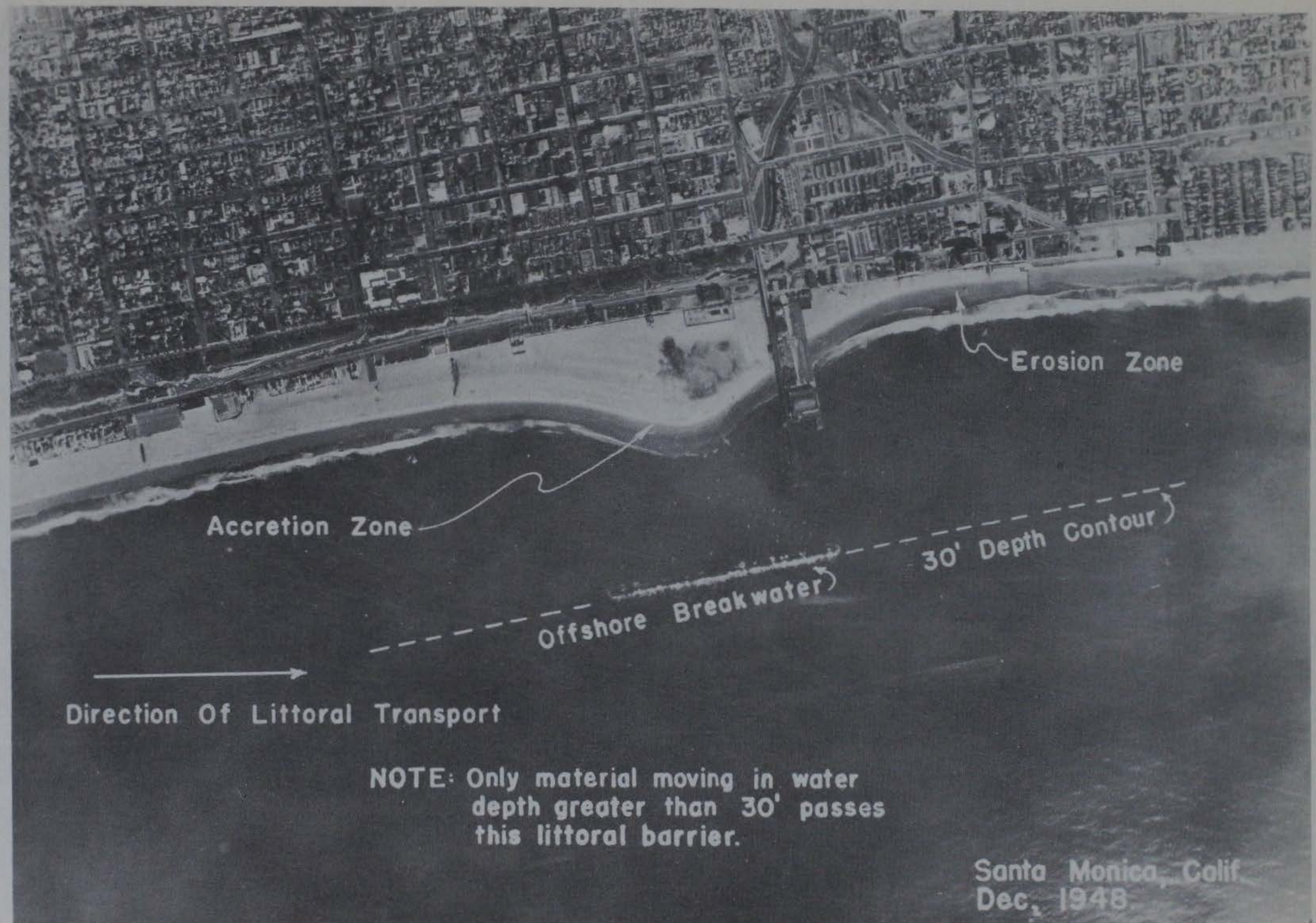
FIGURE 58. SUBSTANTIALLY COMPLETE LITTORAL BARRIER
