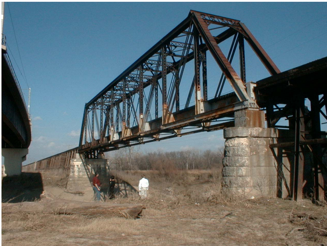
FIGURE 3-5, ATSF Bridge, Dallas Floodway
