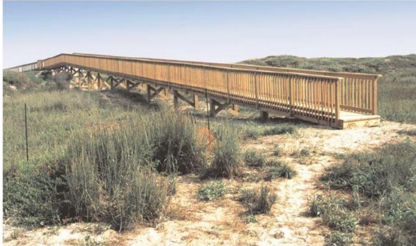
Figure 4-5: Typical Walkover Ramp
