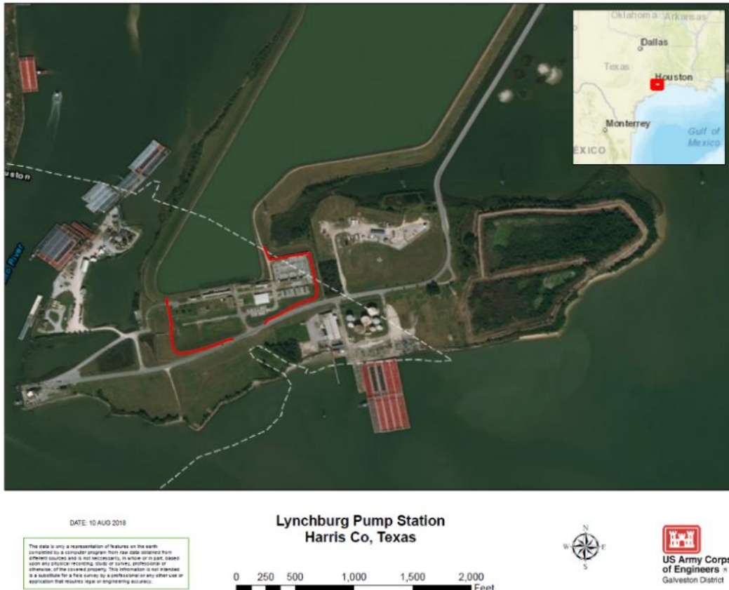
Figure 1-4: Lynchburg Pump Station
