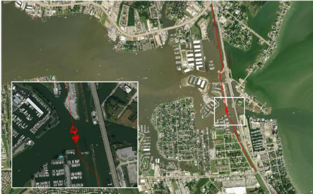
Figure 2-52: Clear Lake Gate System.
