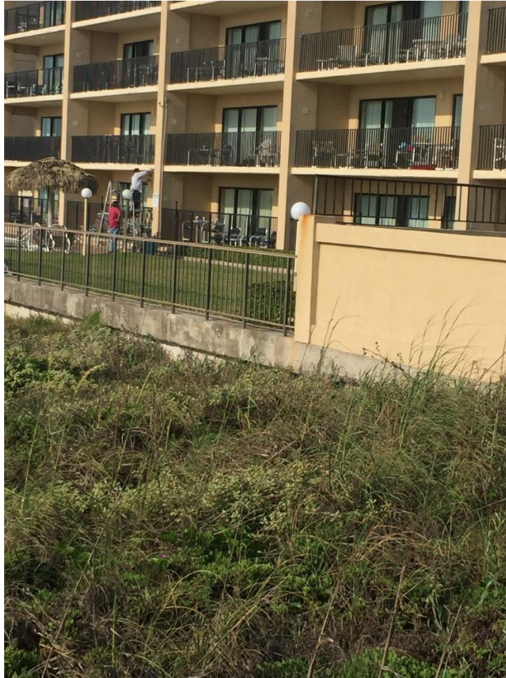
Figure 45: Example of retaining wall at South Padre Island
