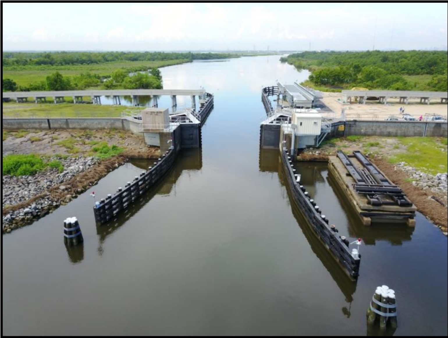
Figure 36 - Example Sector Gate (HSDRRS, Bayou Bienvenue Gate at Back Levee)
