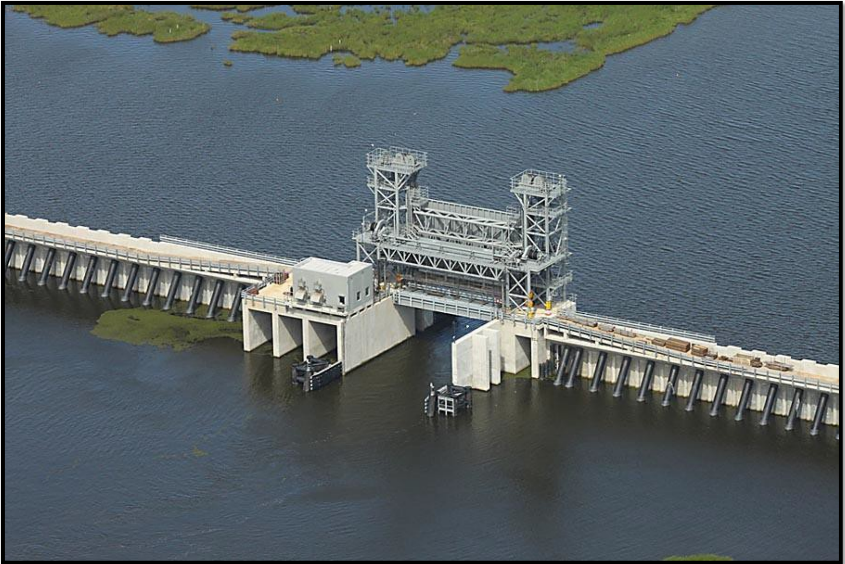
Figure 35 - Example Vertical Lift Gate (HSDRRS, Bayou Bienvenue Gate at Surge Barrier)
