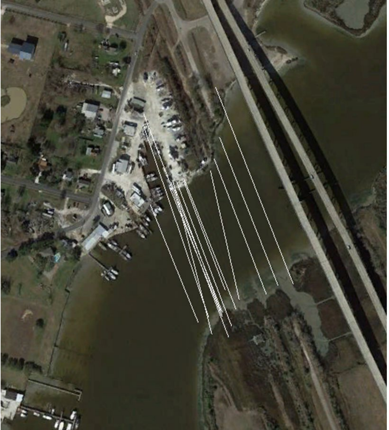
Figure D.2. ROW Pipelines - Dickinson Bayou
