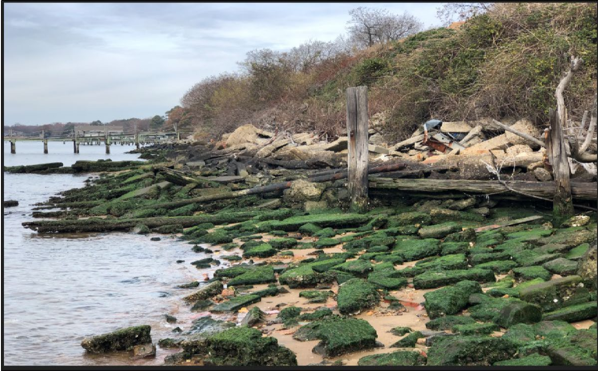
Figure 1-5. View facing northwest of the debris.
