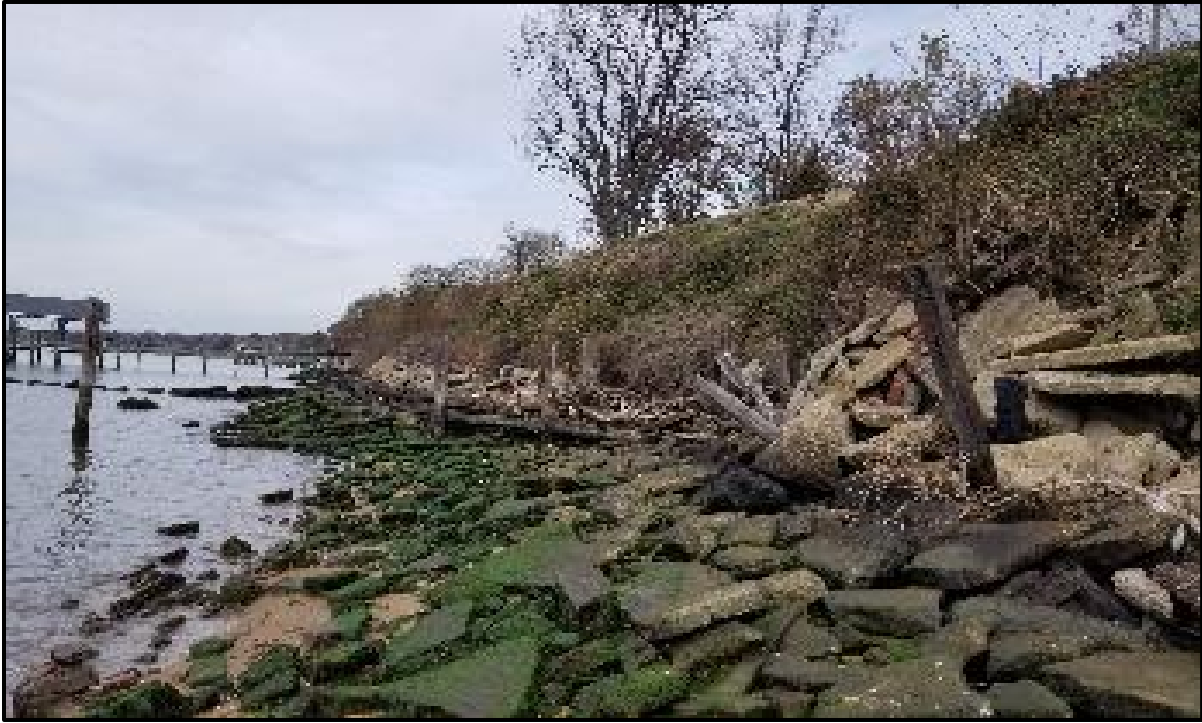
Figure 2. View facing northwest.
