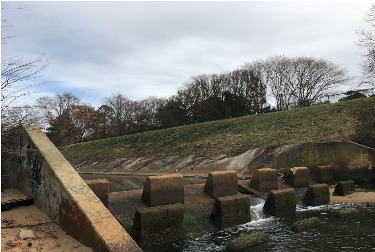
Figure 6-1. Vegetated slope adjacent to Government Ditch. Image taken 2/06/19.
