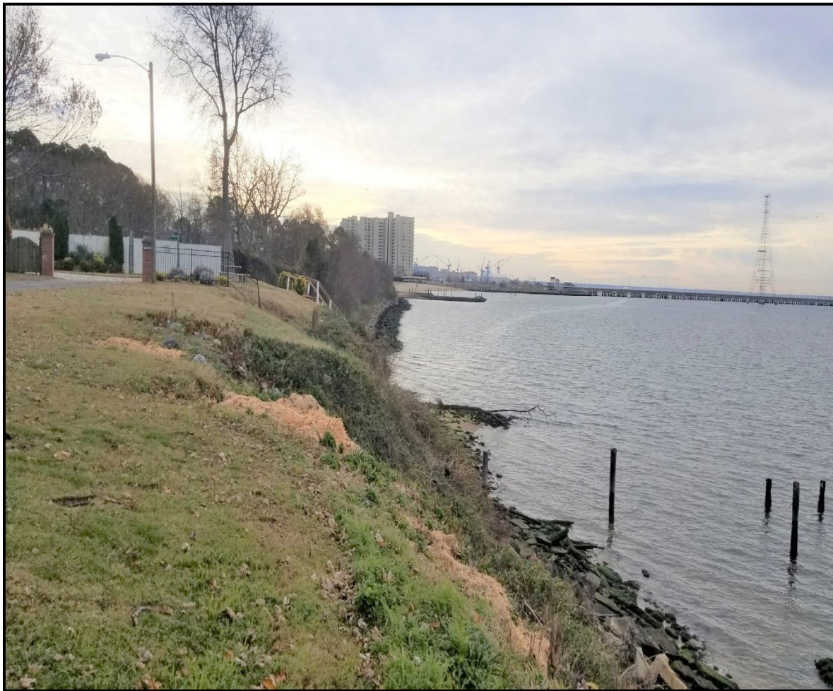
Figure 1-2. View facing southeast of eroding shoreline at project site along
