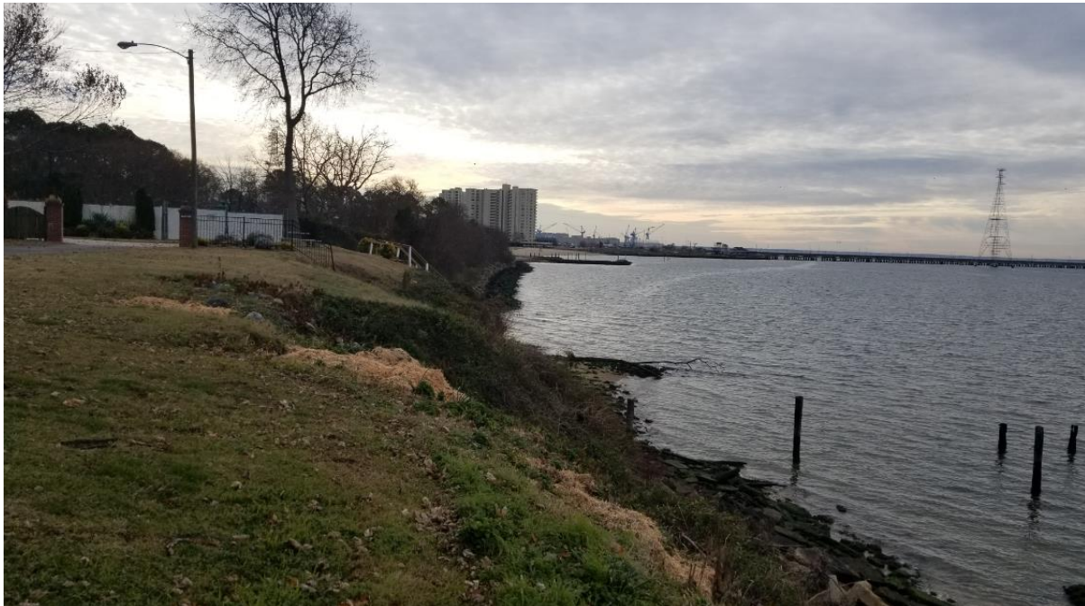
Figure 3.1 Shoreline erosion from the top of the bank in the southern end of the project area
