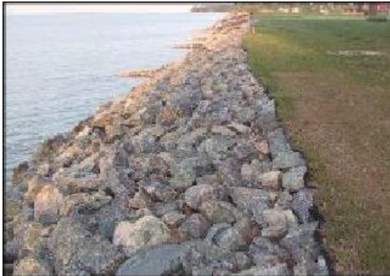
Figure 2.1 Typical Rock Revetment
