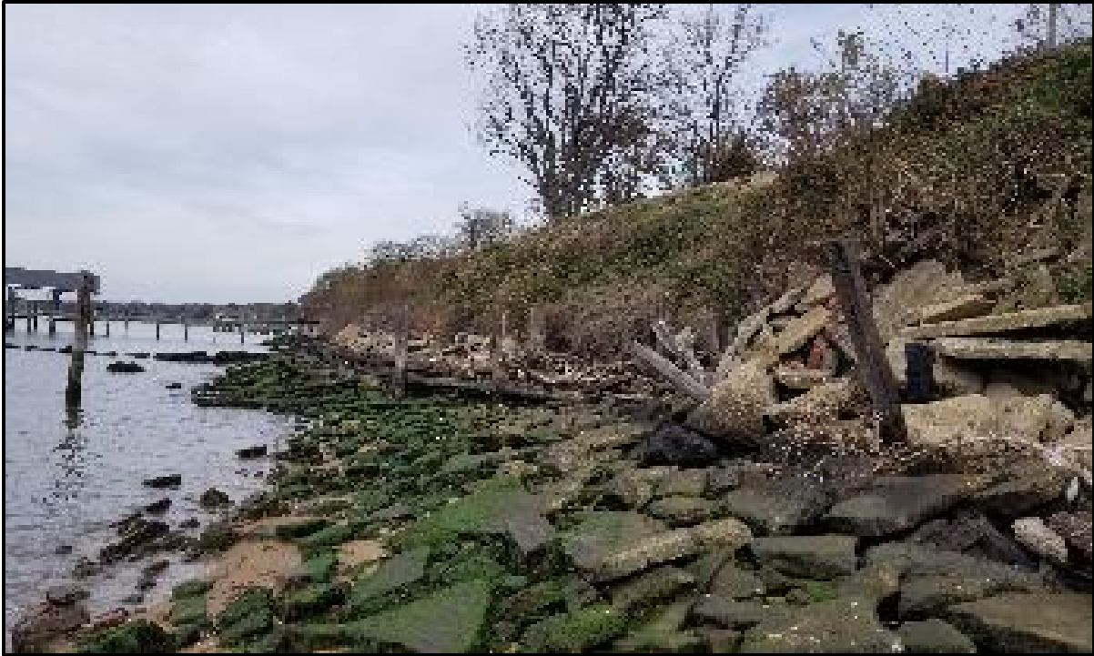
Figure 2. View facing northwest.
