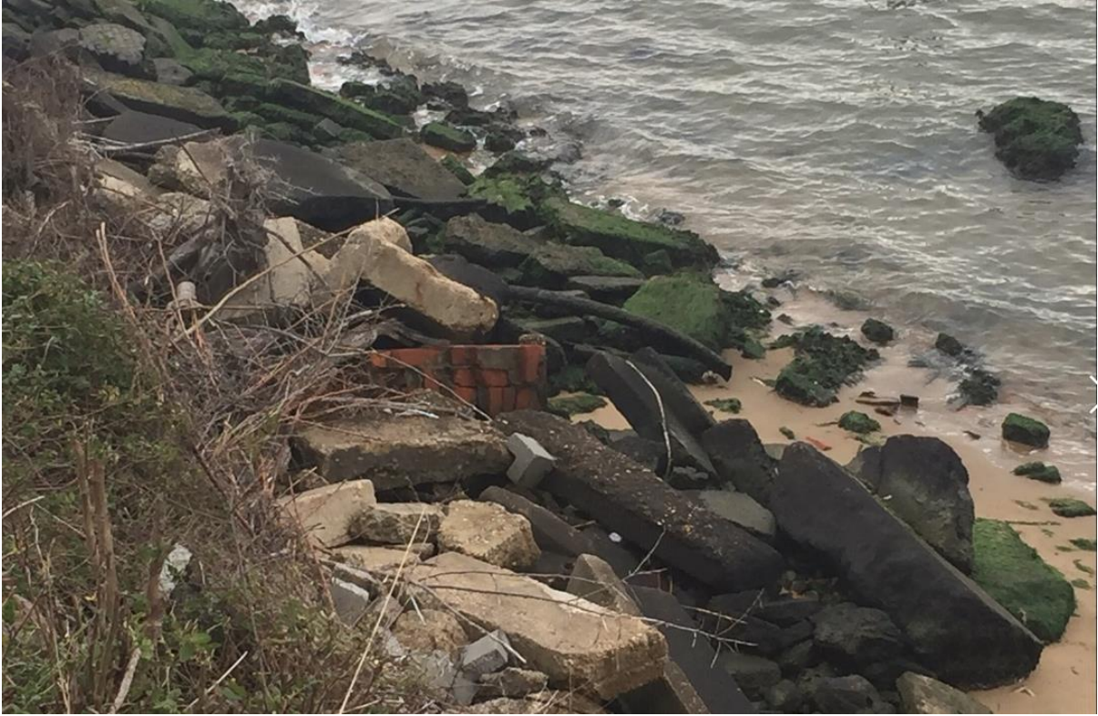
Figure 3.2 Rip rap/debris at the toe of the existing slope
