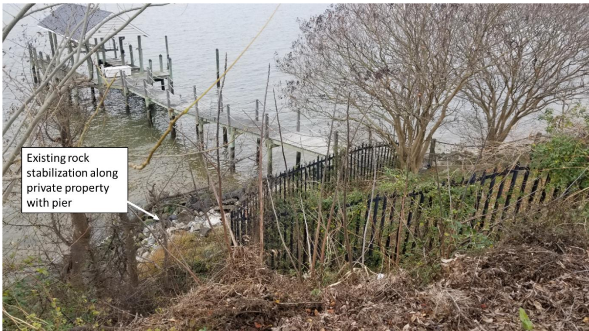
Figure 3.6 Private pier and existing rock stabilization within project area
