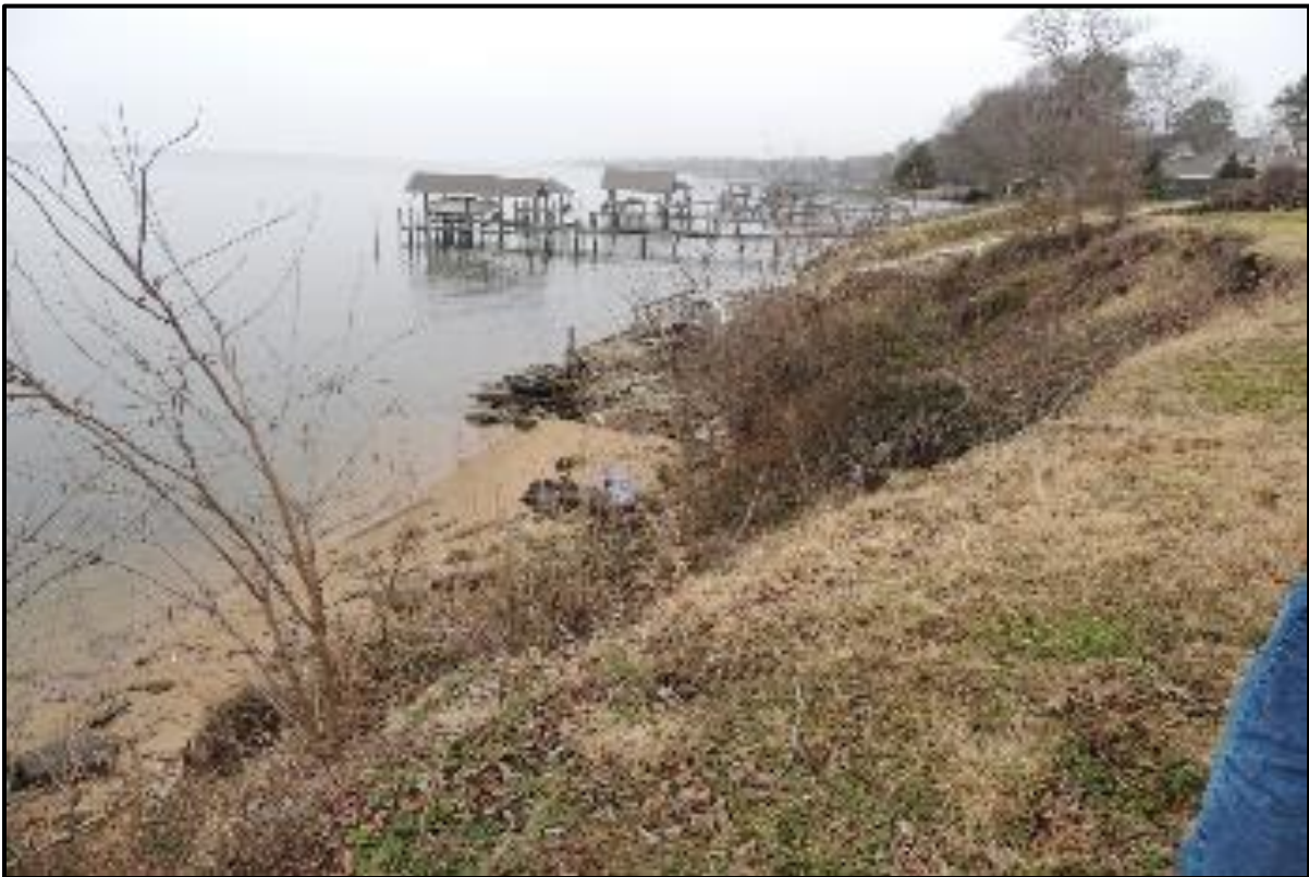
Figure 3. View facing northwest.
