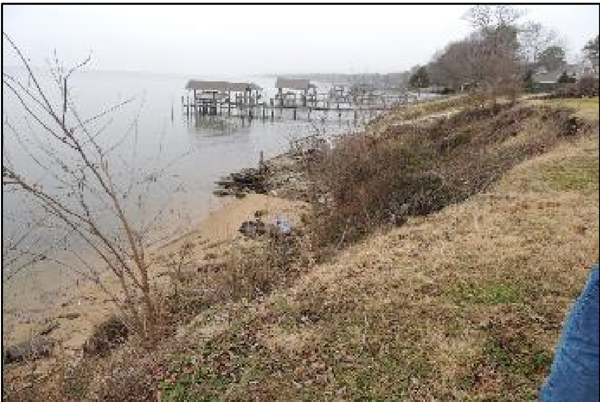
Figure 3. View facing northwest.
