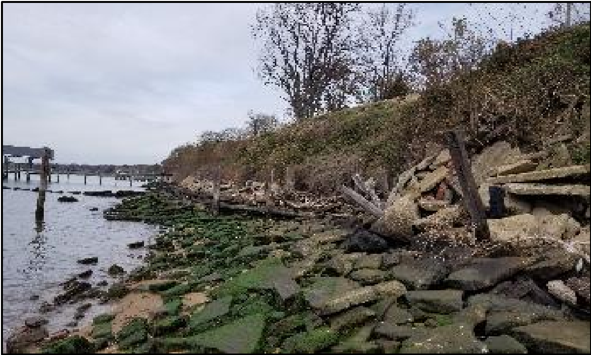
Figure 2. View facing northwest.
