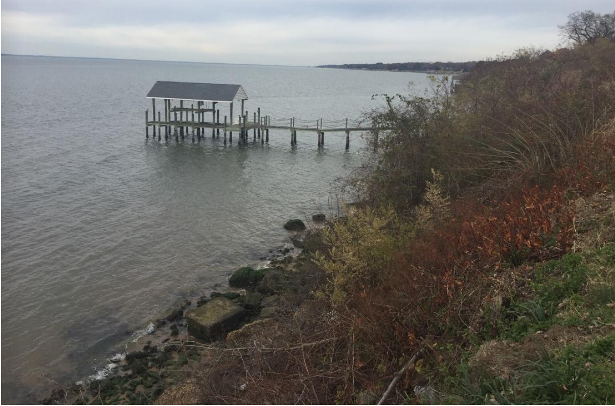
Figure 3.3 Existing slope vegetation along the southern end of the project area
