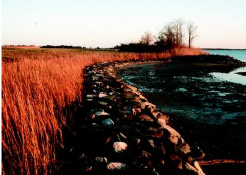
Figure 2.2 Stone sill with marsh planting on Chester River, Kent County, Md.
