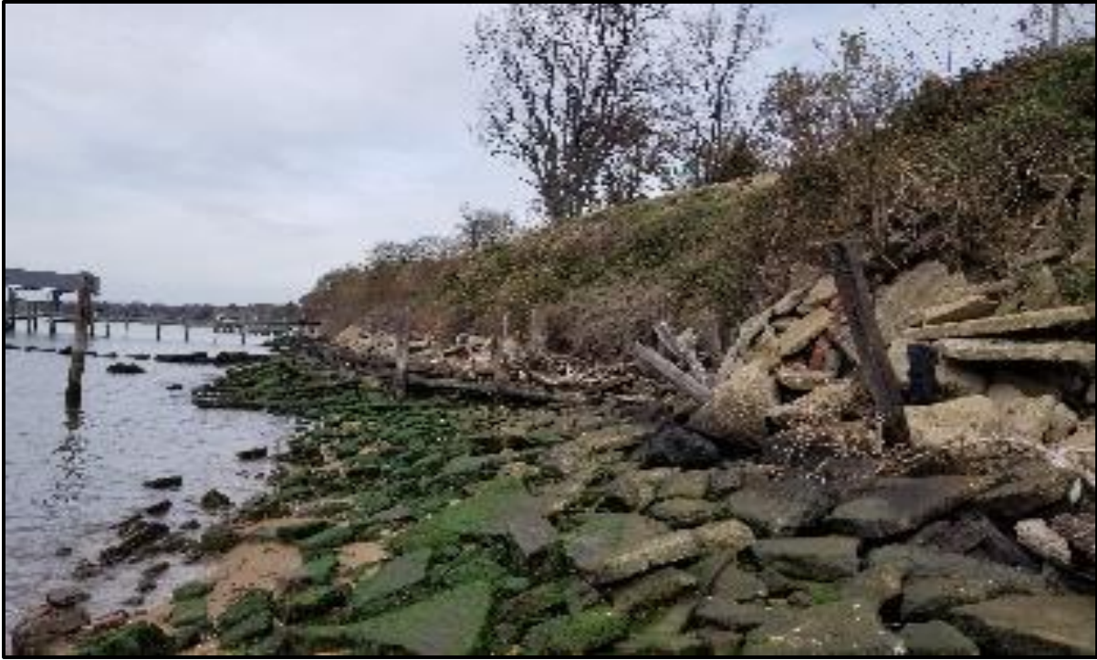
Figure 2. View facing northwest.
