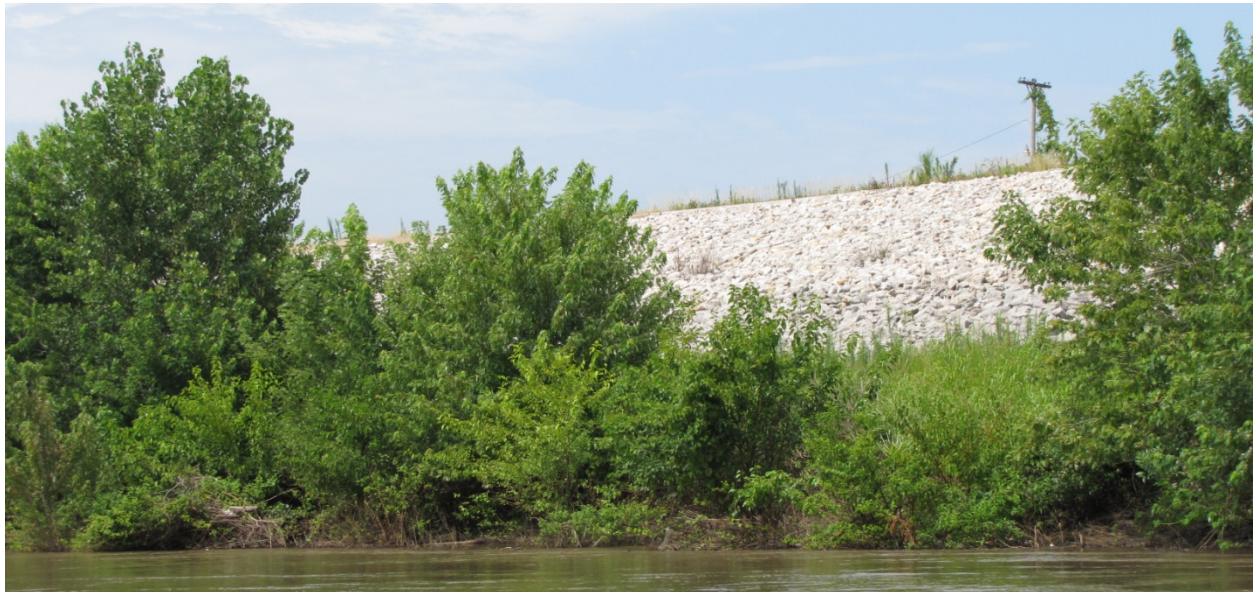
Figure 3. 22. Land accretion inside of a riprap embankment
