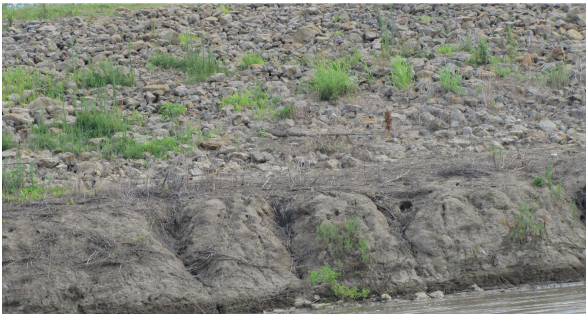
Figure 3. 11. Deposition and land accretion adjacent to a levee. RM 85.8.
