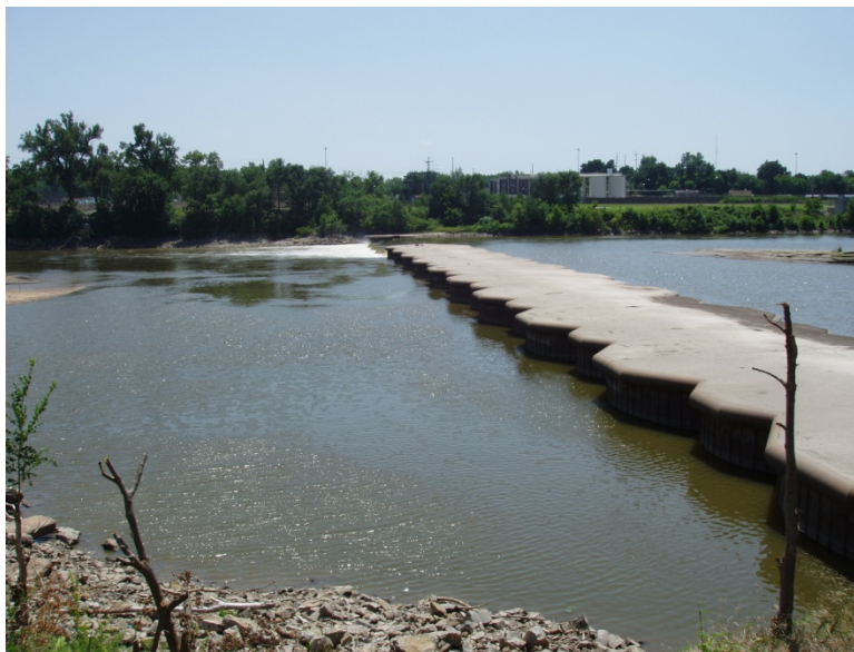
Figure 3. 9. The weir downstream of the Topeka water intake. Flow = 2,080 cfs.
