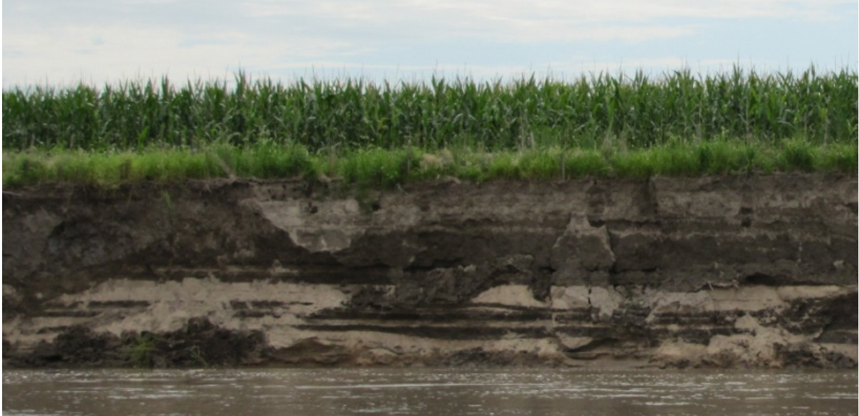
Figure 3. 3. An eroding, vertical bank. RM 167.5.
