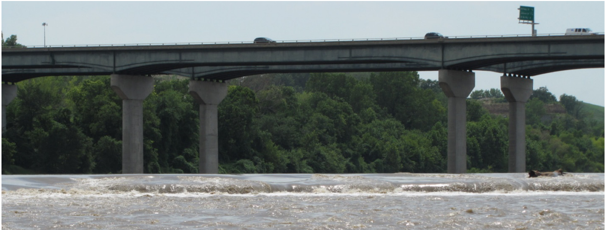
Figure 3. 20. Johnson County Water One Weir.
