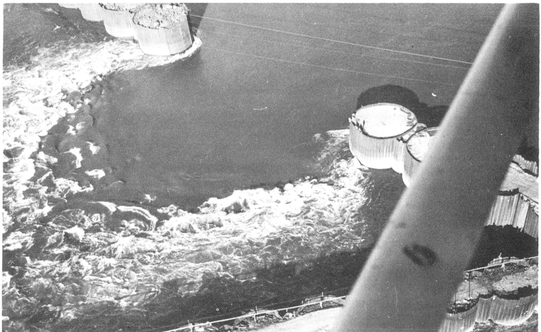
Fig. 28 - Second Tetrahedron Fill nearing completion Aerial view of Water Surface
