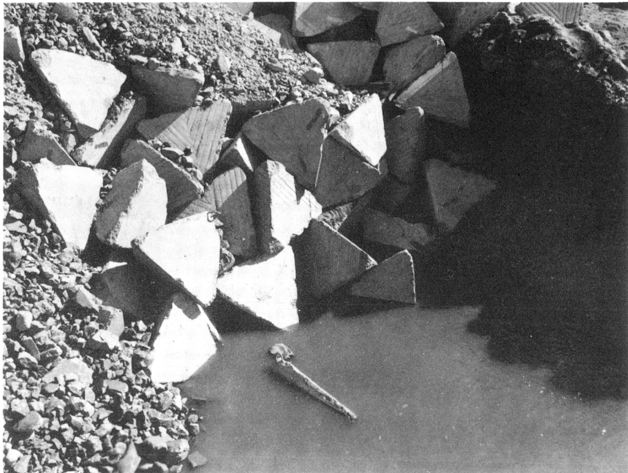
Fig. 48 - Toe of Tetrahedron Fill after unwatering (W.S. El. 218.4)
