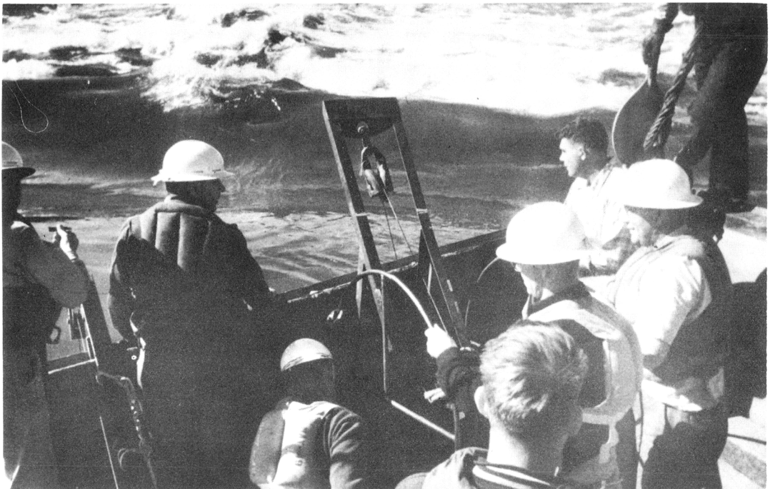
Fig. 22 - Sounding party at work after completion of First Tetrahedron Fill
