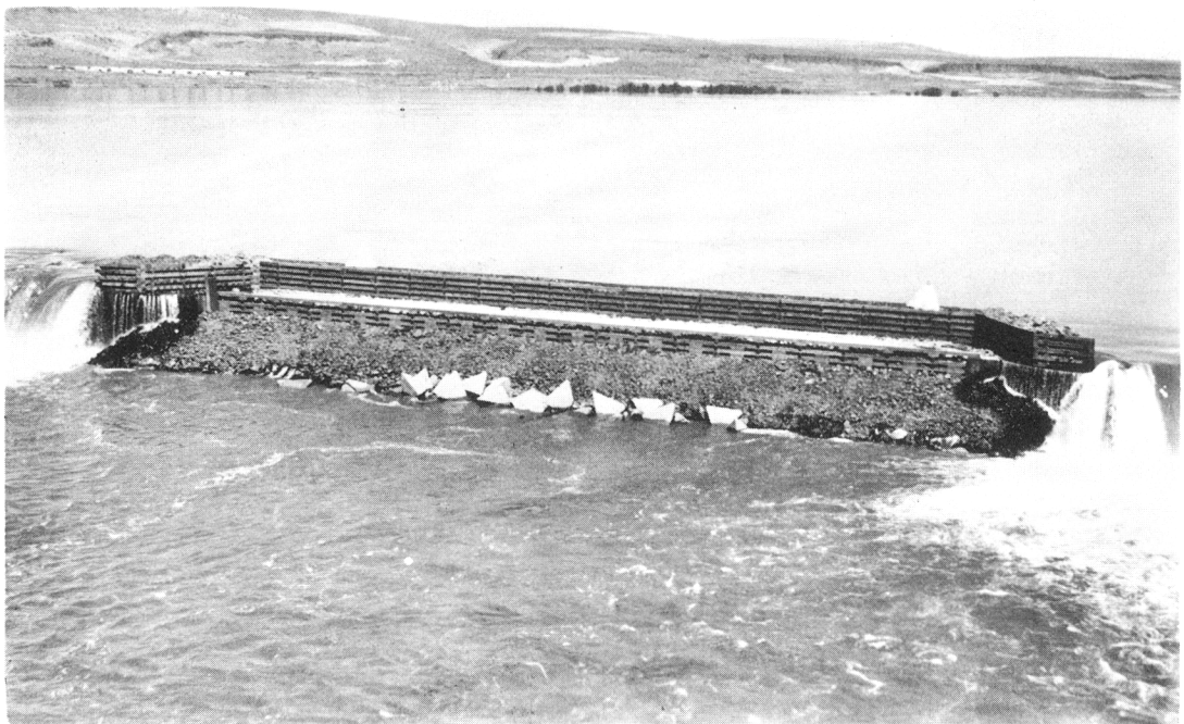
Fig. 50 - Closure Fill during 1951 high water Looking upstream
