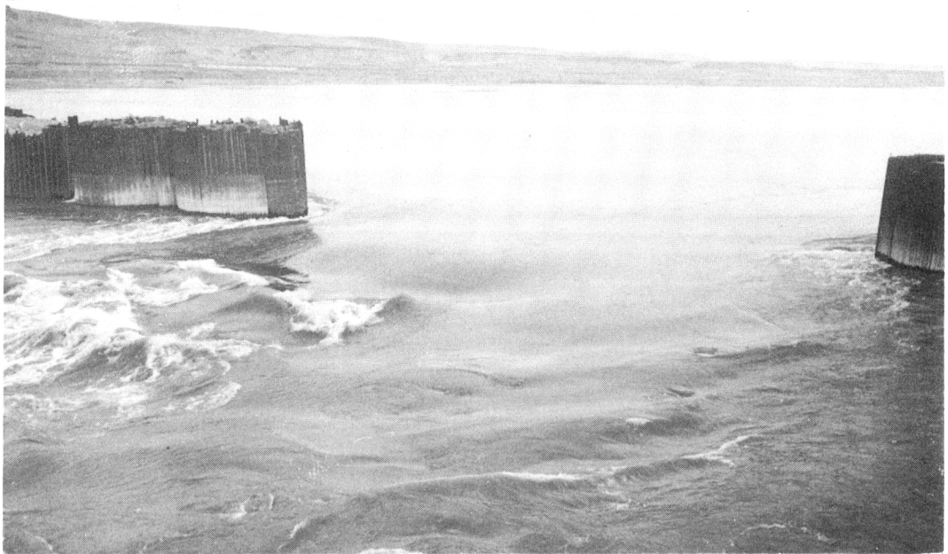
Fig. 19 - First Tetrahedron Fill View of Water Surface after completion
