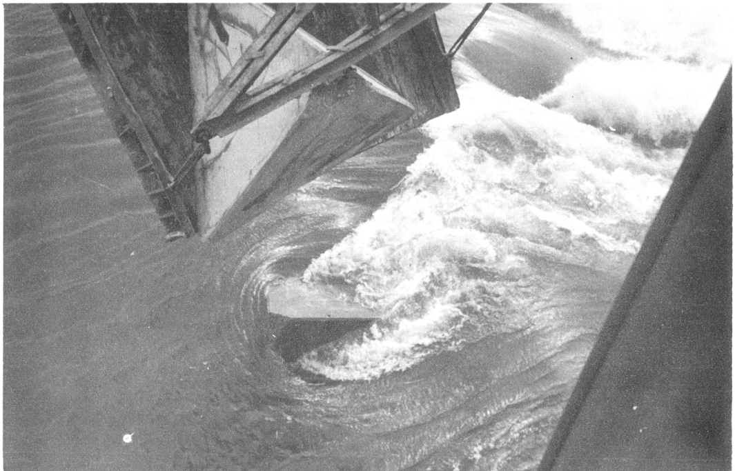
Fig. 36 - Fifth Tetrahedron Fill in progress. Drops to stop "slick" near Cell 17
