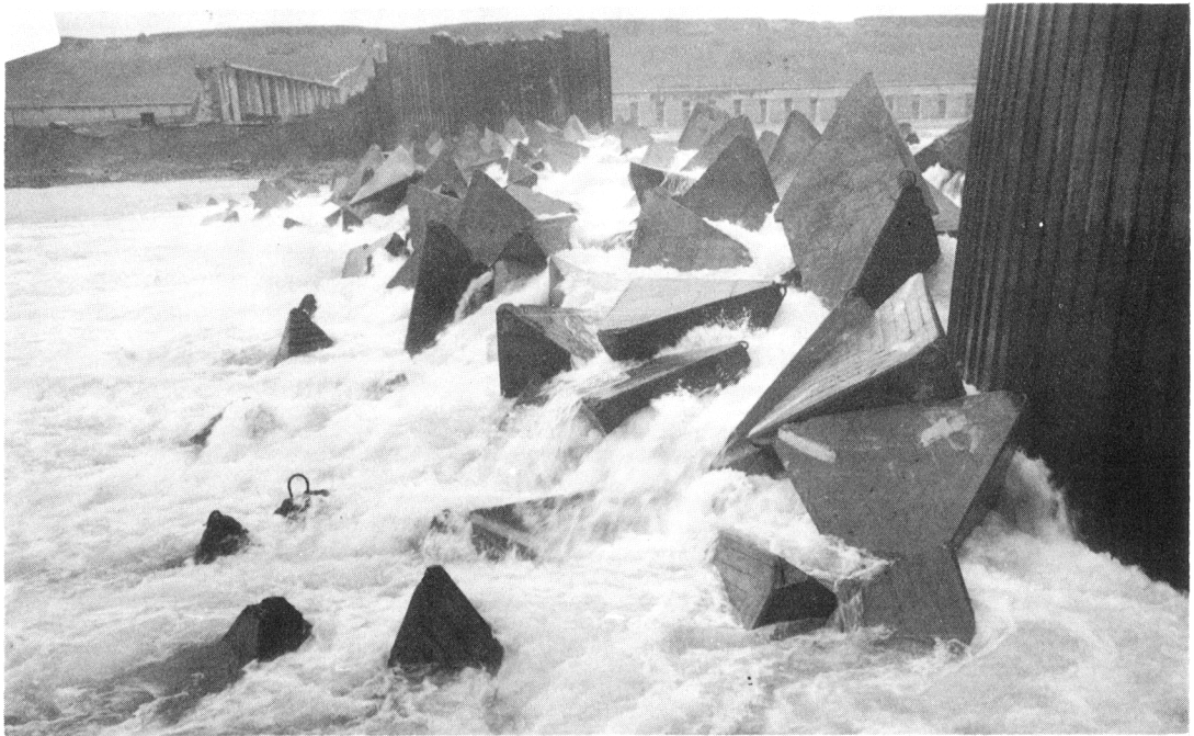
Fig. 41 - Sixth Tetrahedron Fill under construction Looking upstream
