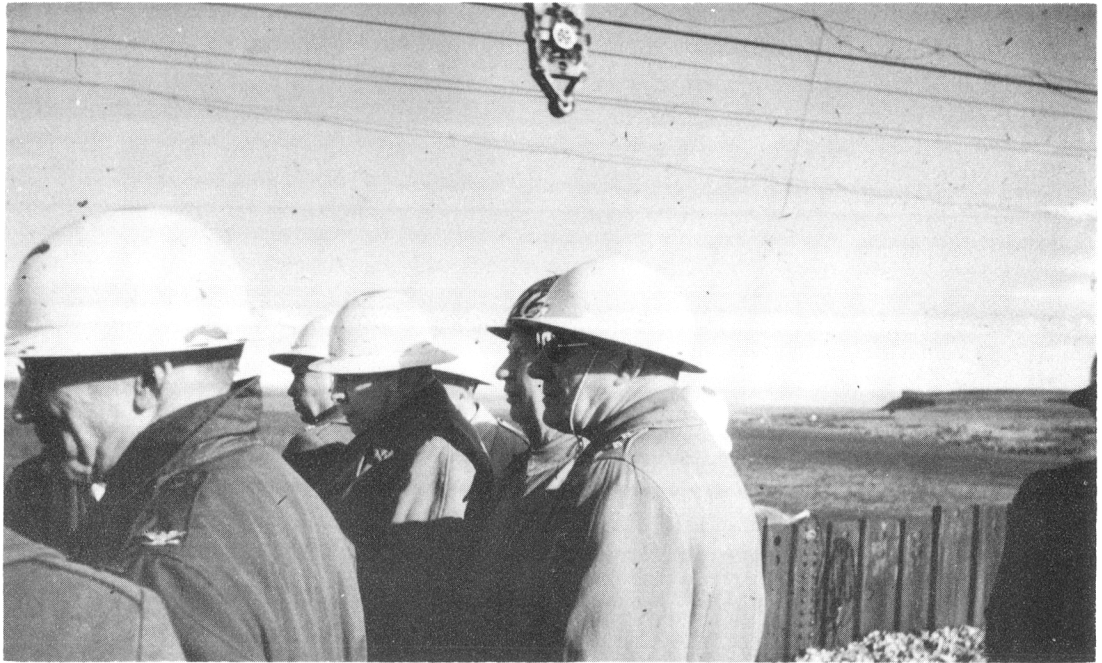
Fig. 39 - General Pick, Chief of Engineers, and other dignitaries inspect closure operation 16 Nov. 1950
