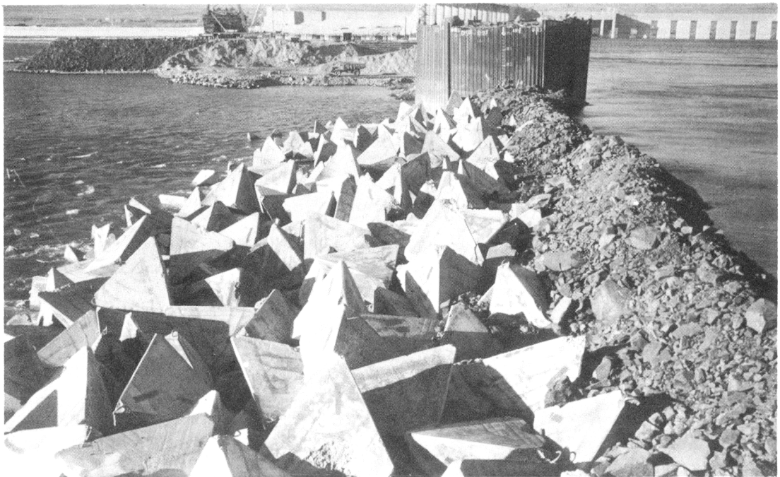
Fig. 42 - Sixth Tetrahedron Fill under construction with some C-stone in place
