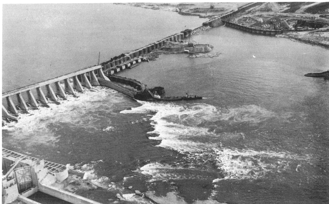
Fig. 44 - Columbia River flow diverted through low spillway bays
