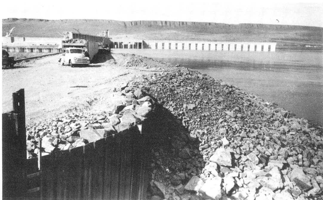
Fig. 46 - Closure Fill and Timber Crib completed
