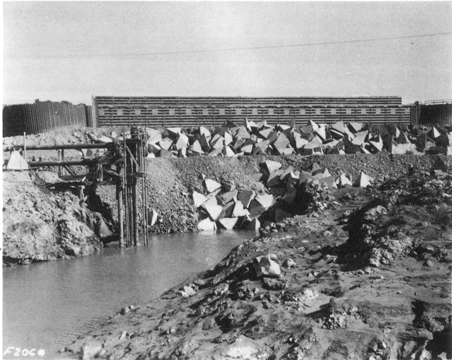
Fig. 47 - Downstream View of Closure Fill after unwatering (W.S. El. 218.4)
