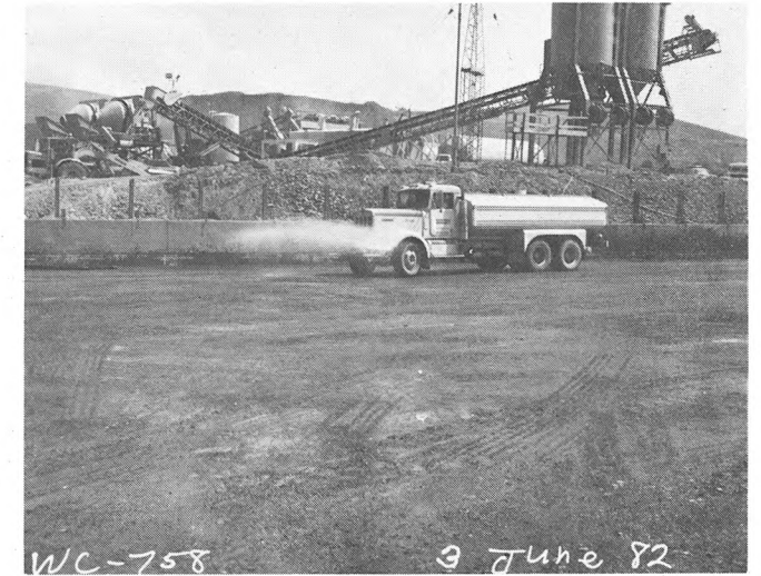
WATER TRUCK MISTING THE SURFACE TO KEEP THE LIFT SURFACE DAMP.
