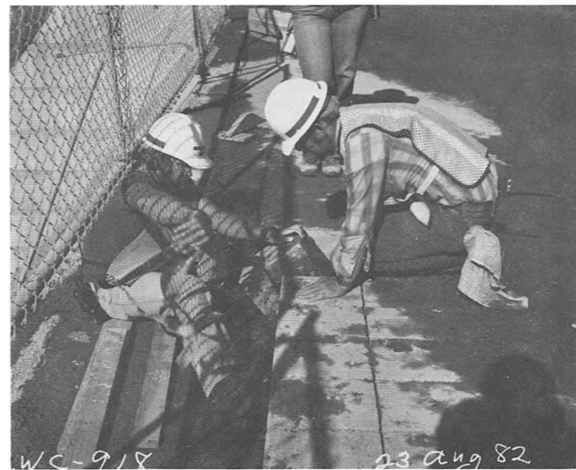
REMOVING TEST BLOCKS FROM THE DAM.
