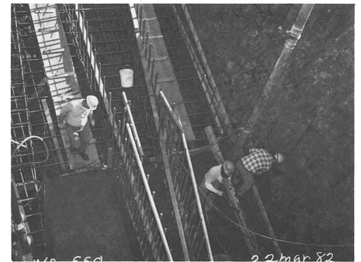
PLACING CONVENTIONAL CONCRETE IN THE OUTLET WORKS BY PUMP.
