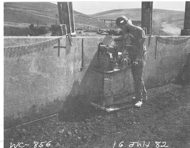
HAND COMPACTION OF RCC ADJACENT TO THE PANELS.
