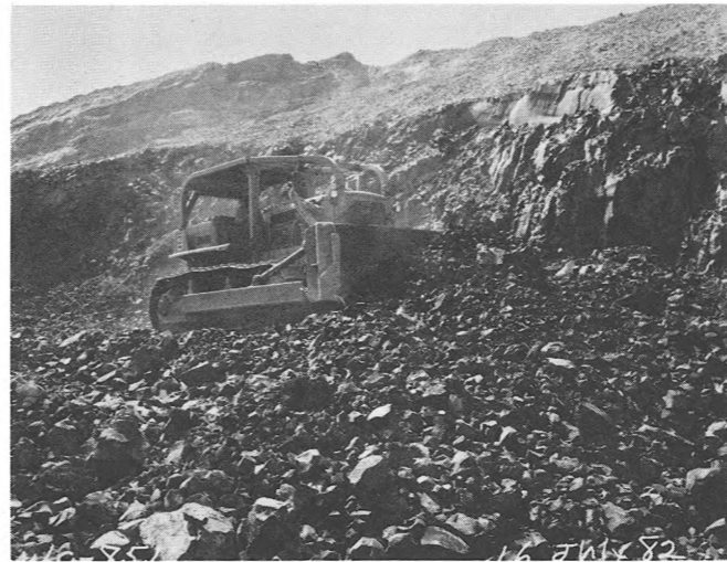
DOZING SHOT ROCK TO THE CRUSHER.
