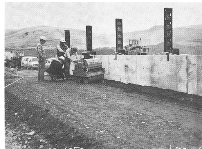
COMPACTION WITH FULL PRODUCTION EQUIPMENT.
