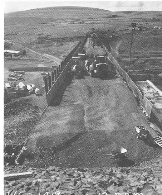
NARROW WORK AREA NEAR THE TOP OF THE DAM.
