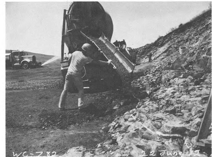
PLACING BEDDING ON THE FOUNDATION PRIOR TO ROLLING RCC INTO IT.
