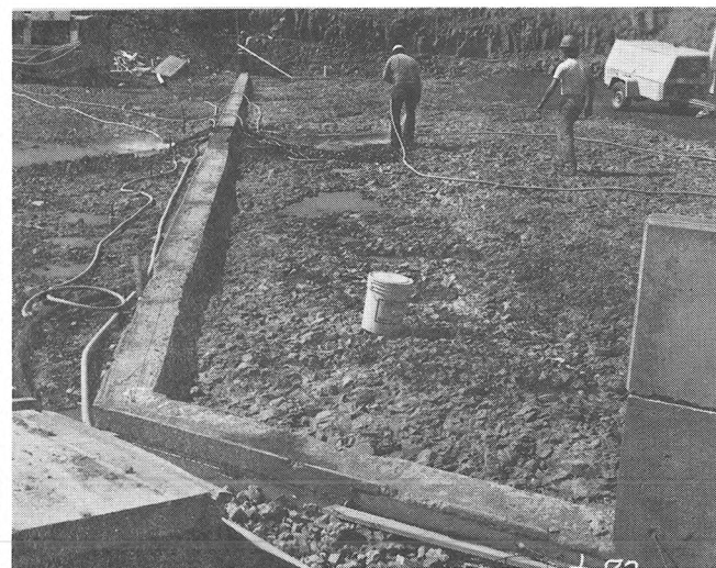
STARTER CURB/WALL FOR THE UPSTREAM PANELS.
