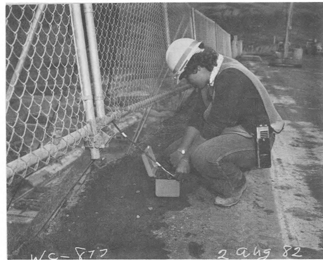
READING EMBEDDED RESISTANCE THERMOMETERS.
