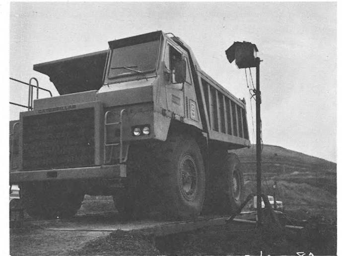
EACH LOAD TO STOCKPILE WAS WEIGHED.
