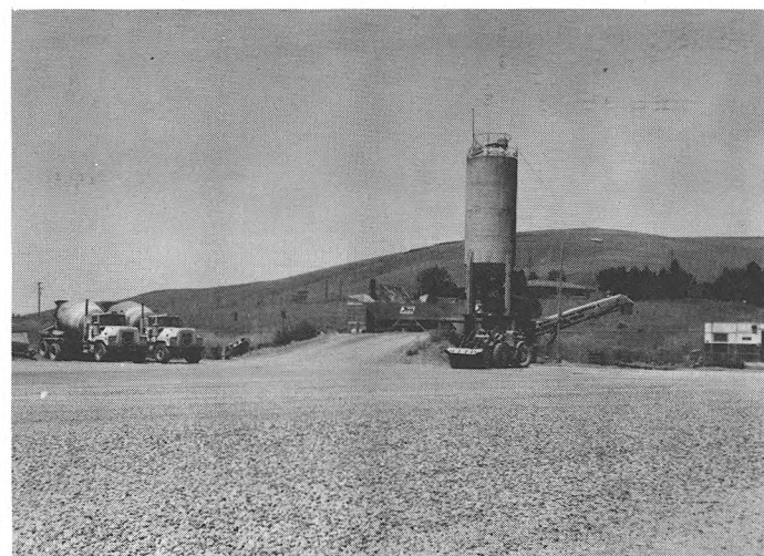
CONCRETE PLANT AND TRUCK
