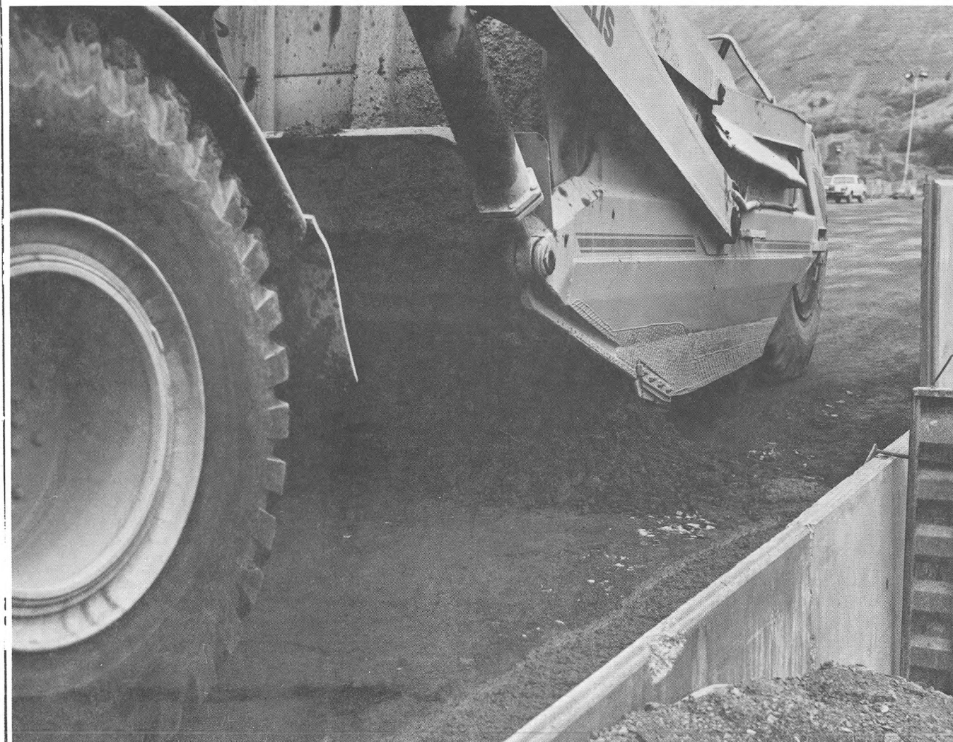
DUMPING FROM A SCRAPER HOLDING 16 CUBIC YARDS.
