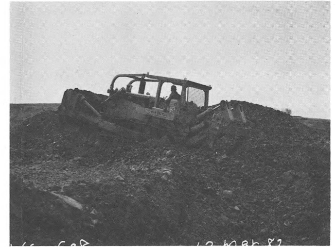
DOZING OVERBURDEN TO THE CRUSHER.
