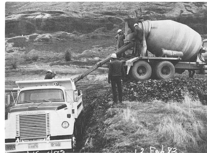
DISCHARGE FROM MIXER TRUCK INTO DUMP TRUCK.
