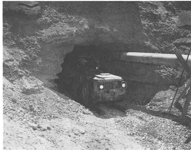
MUCKING OUT AGGREGATE FILL FROM THE GALLERY.
