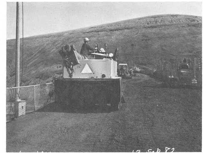
PNEUMATIC ROLLER USED IN A TRIAL AREA.
