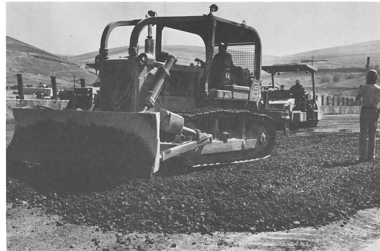
SPREAD WITH A D-6 DOZER.
