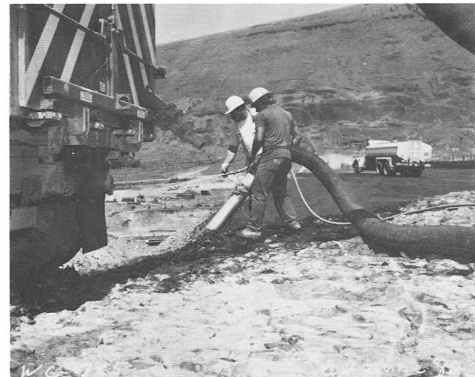
VACUUM CLEANUP OF THE FOUNDATION.
