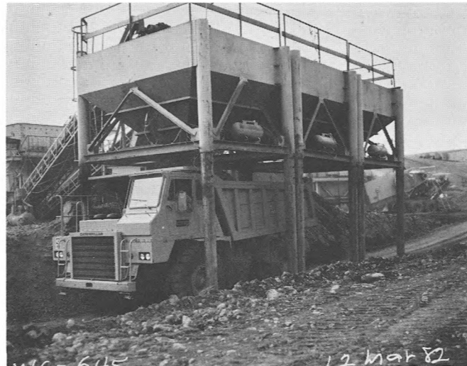
LOADING 1 1/2 AND 3 INCH AGGREGATE.
