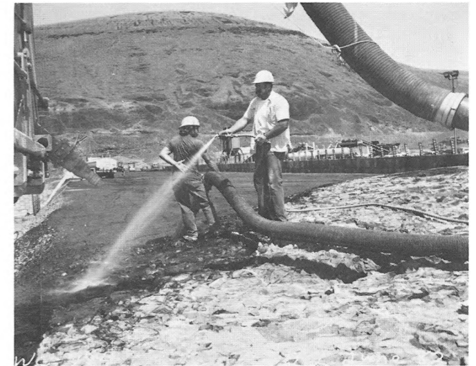
FOUNDATION CLEANUP WITH A STANDARD GARDEN HOSE AND THE VACUUM.
