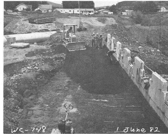
PLACING RCC BEHIND THE RIGHT TRAINING WALL.
