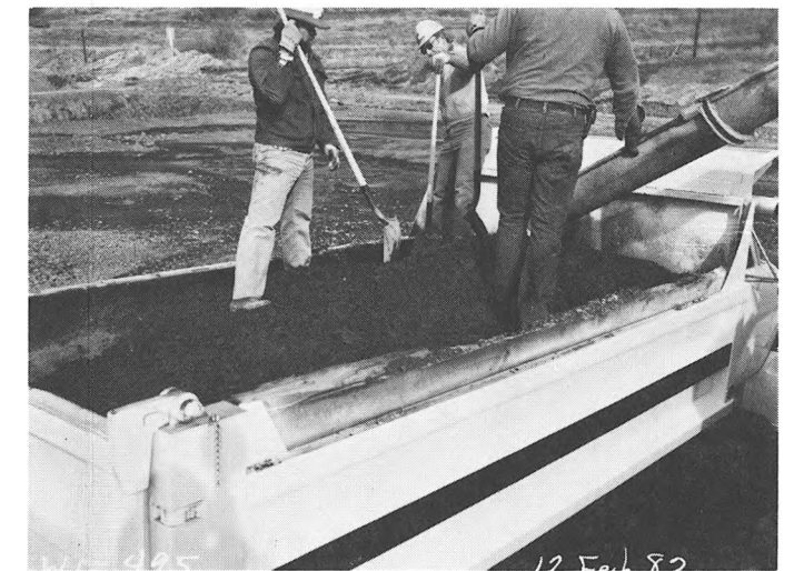
HAND WORKING RCC TO MINIMIZE SEGREGATION FROM THE READY MIX TRUCK.
