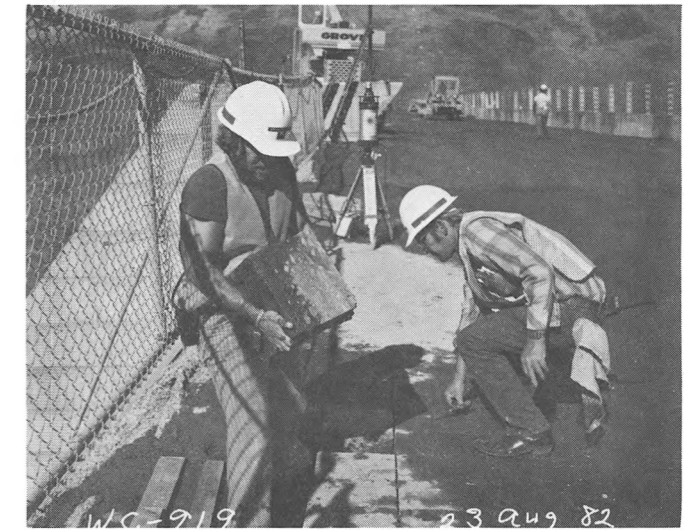
TEST BLOCK AT AN AGE OF 36 HOURS.
