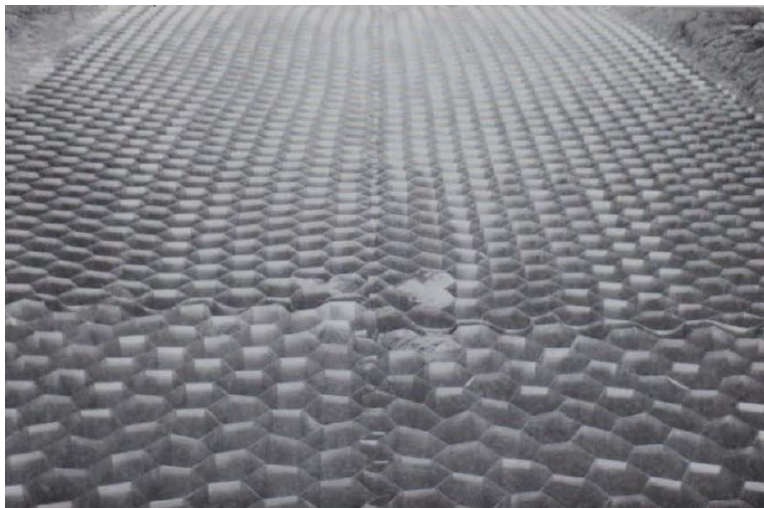
Figure 1-1. Hexagonal geocells (Webster 1981).
