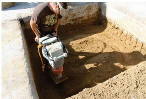
(c) Compaction of the CL layer with the rammer.
