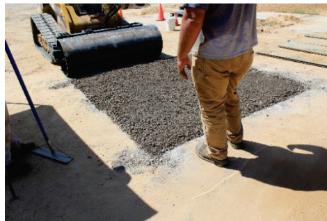
Compacting GP-GM with CV18B.
