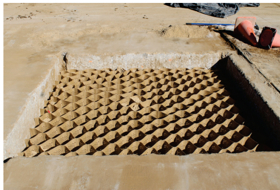
Figure 3-3. Neoweb geocell.
