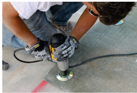
(e) Applying torque to concrete anchor bolt.
