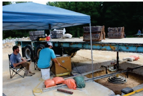
(a) Overall view of plate bearing test.
