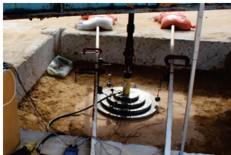
(b) Closeup view of plate bearing test.
