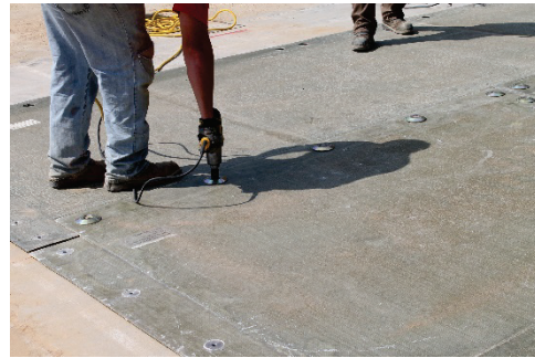
(b) Applying torque to connector bushing bolt.
