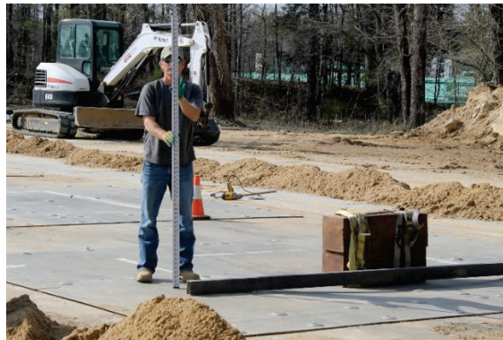
(b) Loaded cross-section measurements on the FRP FOD cover.
