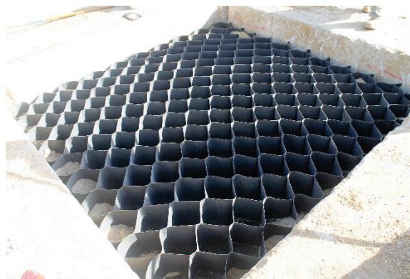
Figure 3-4. Typar geocell.
