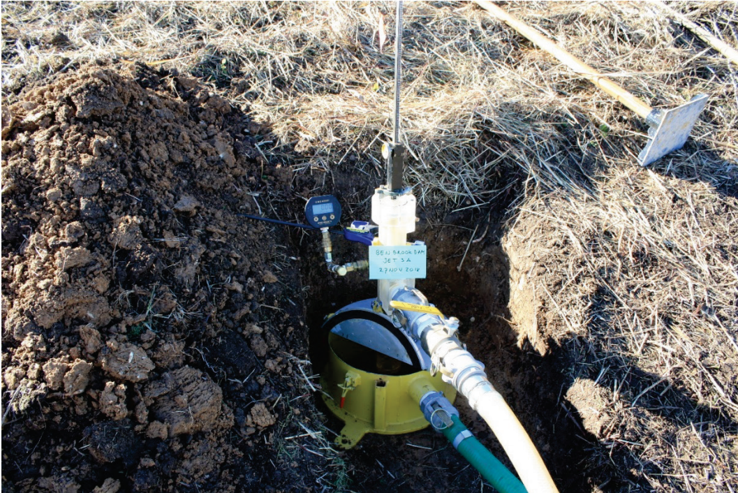
Figure 7. Benbrook JET 3A in progress.
