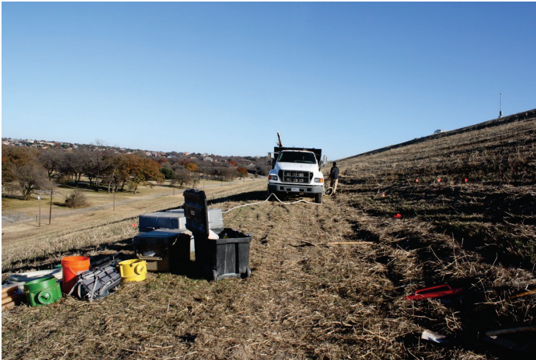
Figure 5. Site preparation for JET.
