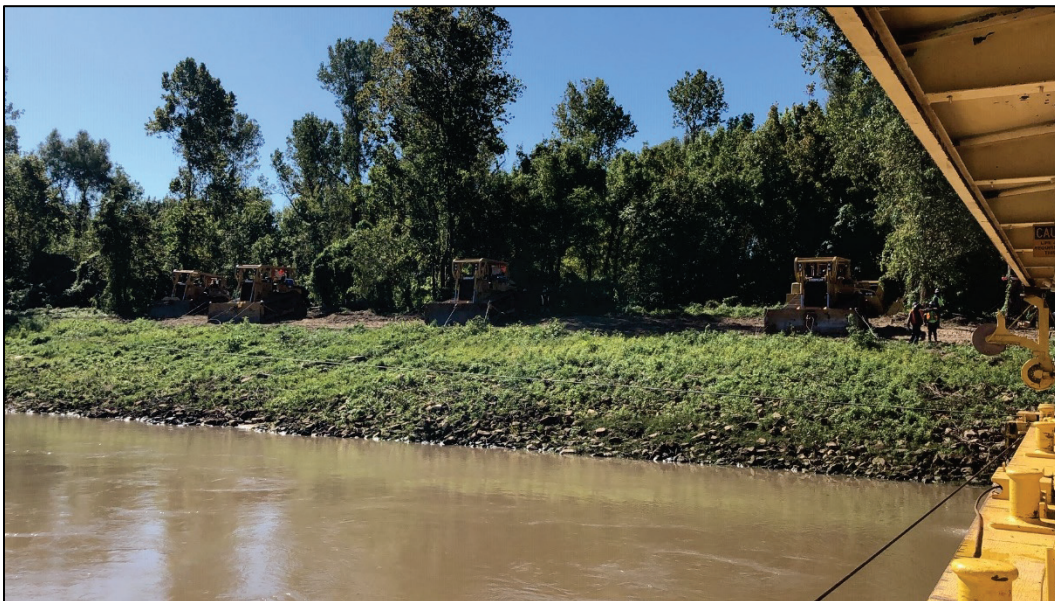
Figure 12. Dozer landside anchoring ACMs.
