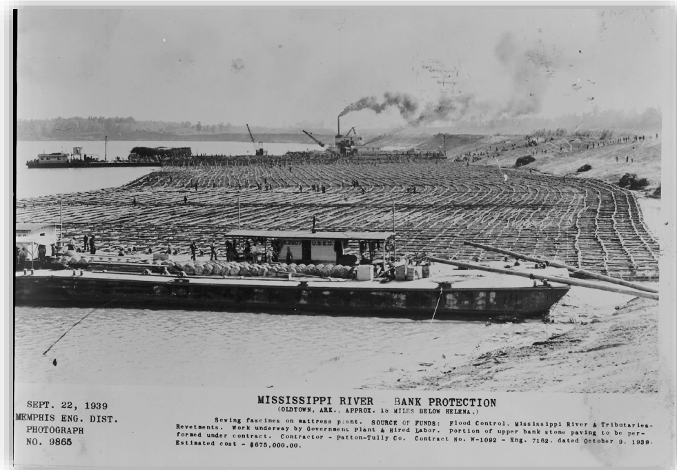
Figure 3. Wood and stone material used for bank protection in 1939 (courtesy of Memphis District [MVM]).
