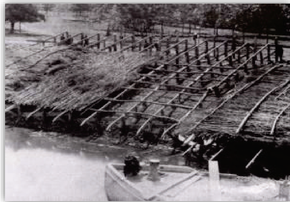
Figure 2. Willow mats being constructed by weaving the material (courtesy of MVK).
