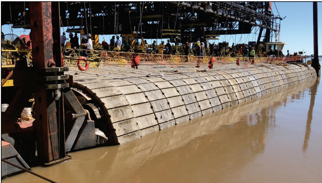
Figure 14. Operations on MSU for ACM placement.
