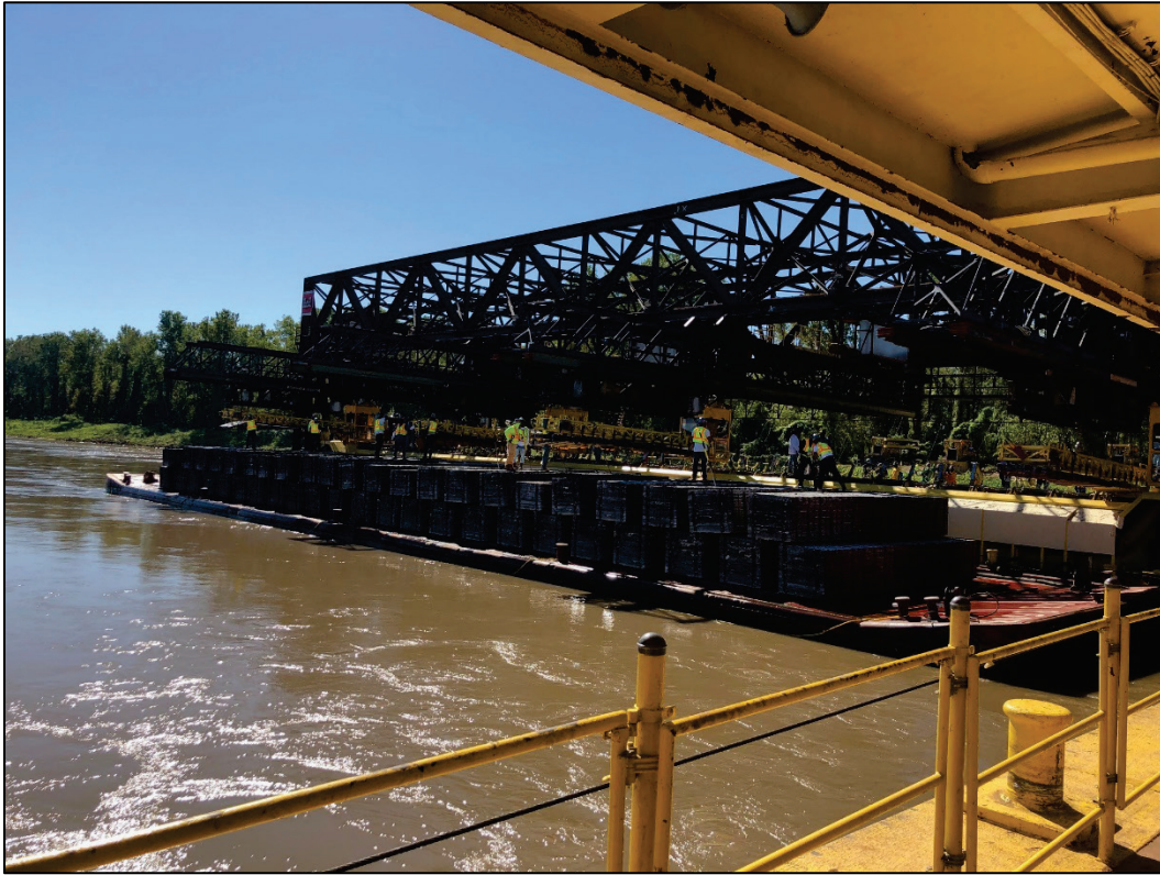
Figure 13. Supply stack barge for MSU operations.
