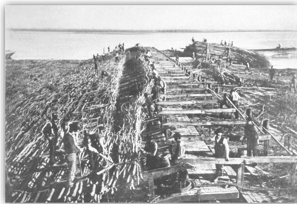
Figure 1. Willow mats being constructed by weaving the material (courtesy of Vicksburg District [MVK]).
