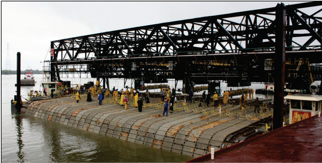
Figure 9. Workers tying mats during placement.
