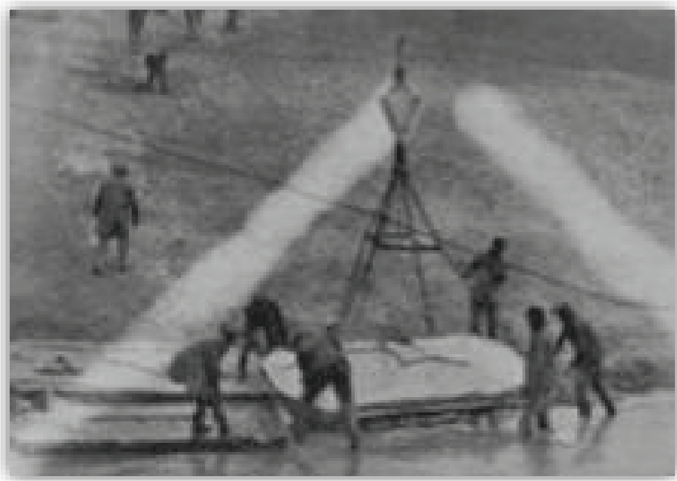
Figure 5. Personnel assist with placement of concrete slabs (courtesy of MVK).
