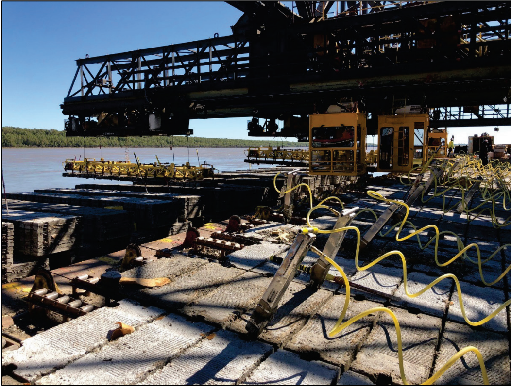
Figure 15. ACM being offloaded from supply barge.
