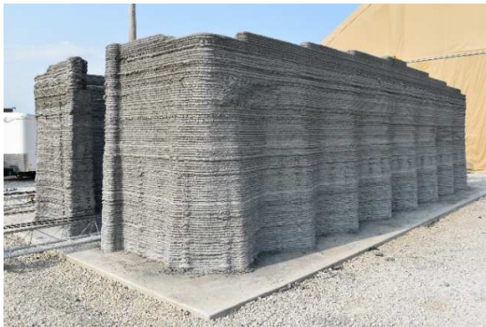
Figure 6. Completed North Wall.
