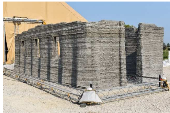
Figure 7. Completed South Wall.
