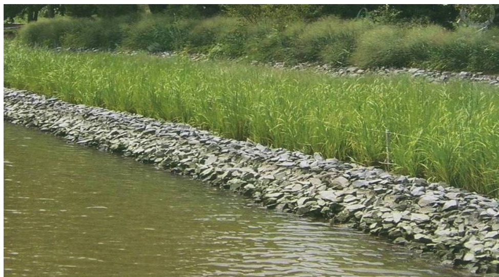
Figure 6-1. Tidal Wetland Flanked by a Stone Sill
