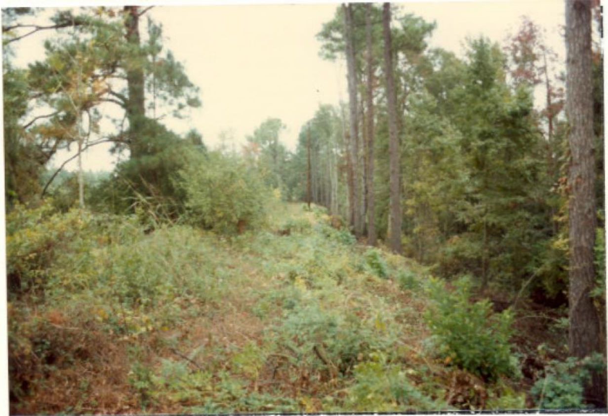
Photo 3 : Dam Crest view from right end of dam
