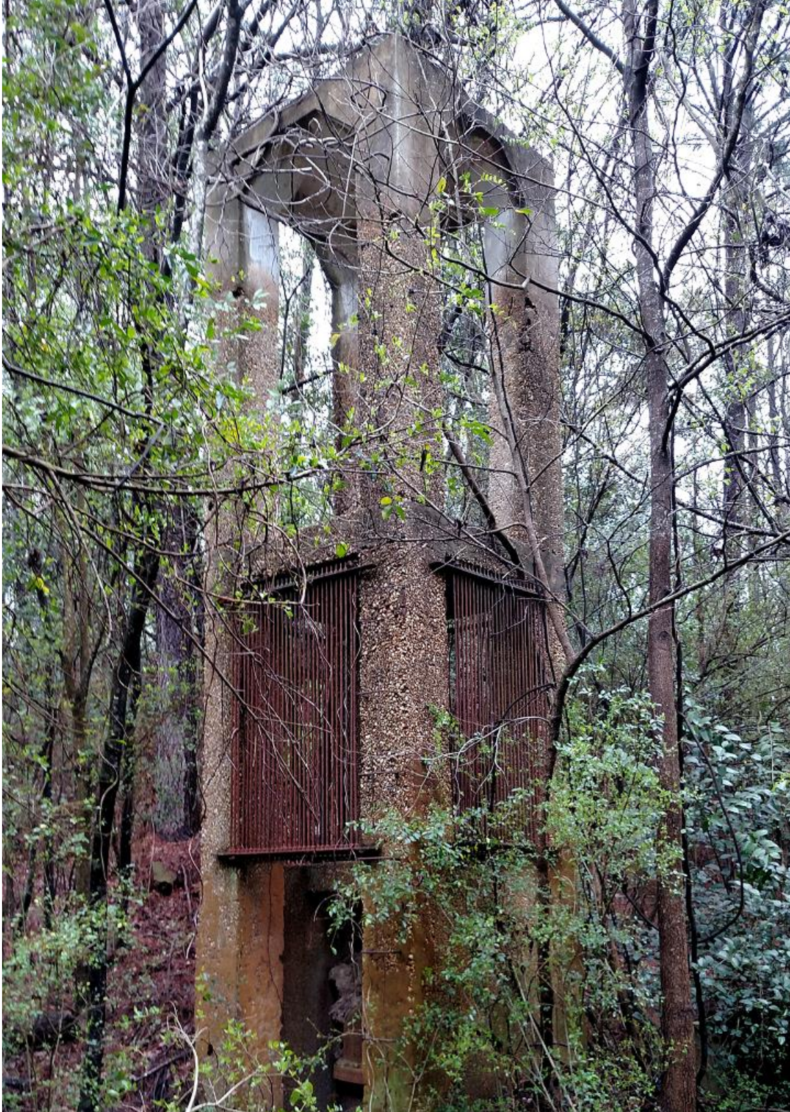
Photo 9 : Old Outlet Structure
