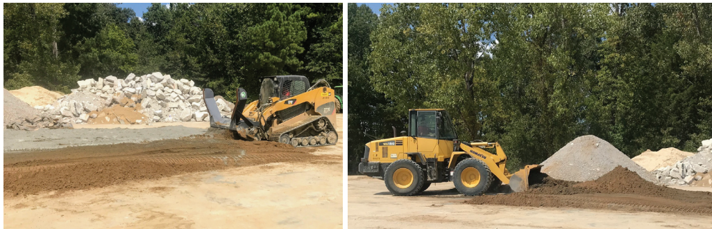
Figure 17. Tiller attachment mixing cement with silty sand and flipping soil with front-end loader.
