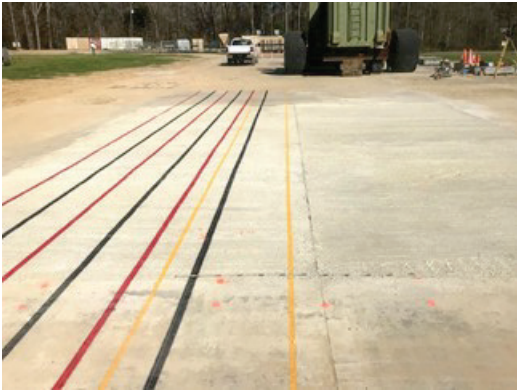
(a) Overview of repair at 0 passes
