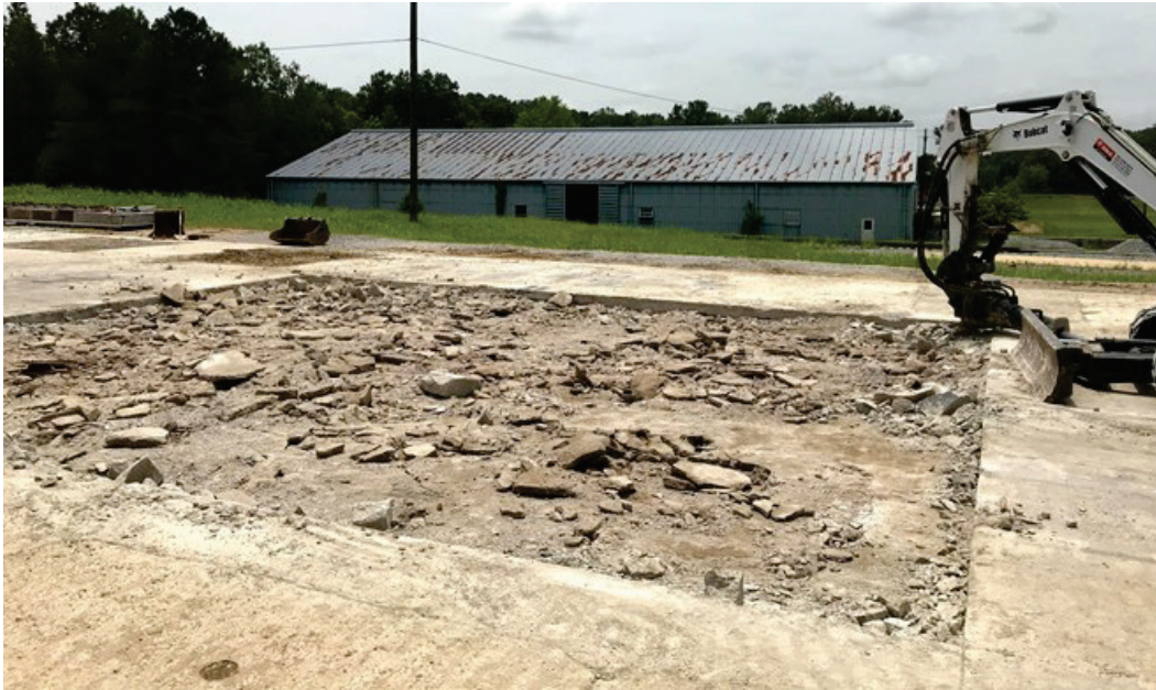
Figure 45. Close-up of flowable fill layers during removal.
