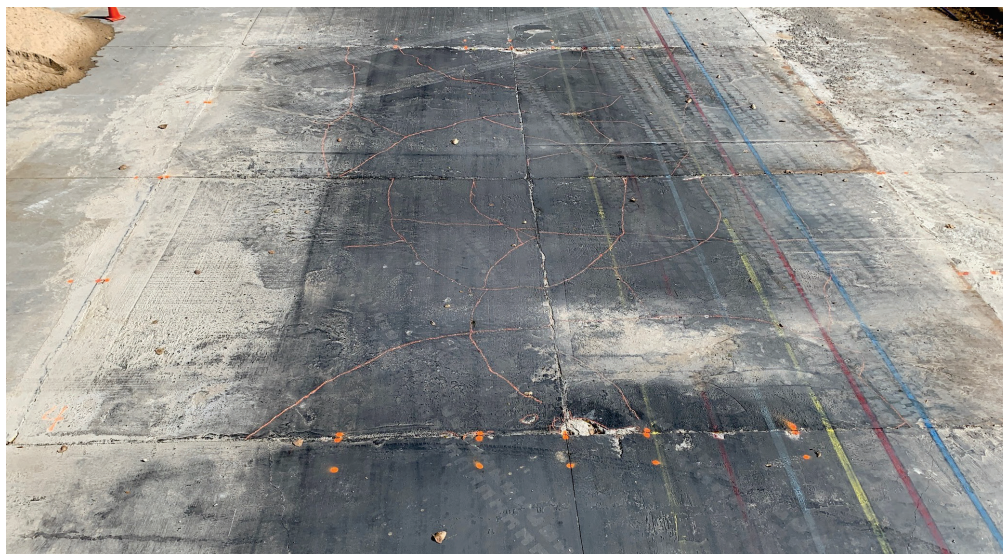
Figure 55. Overview of repair 7 after 896 passes.
