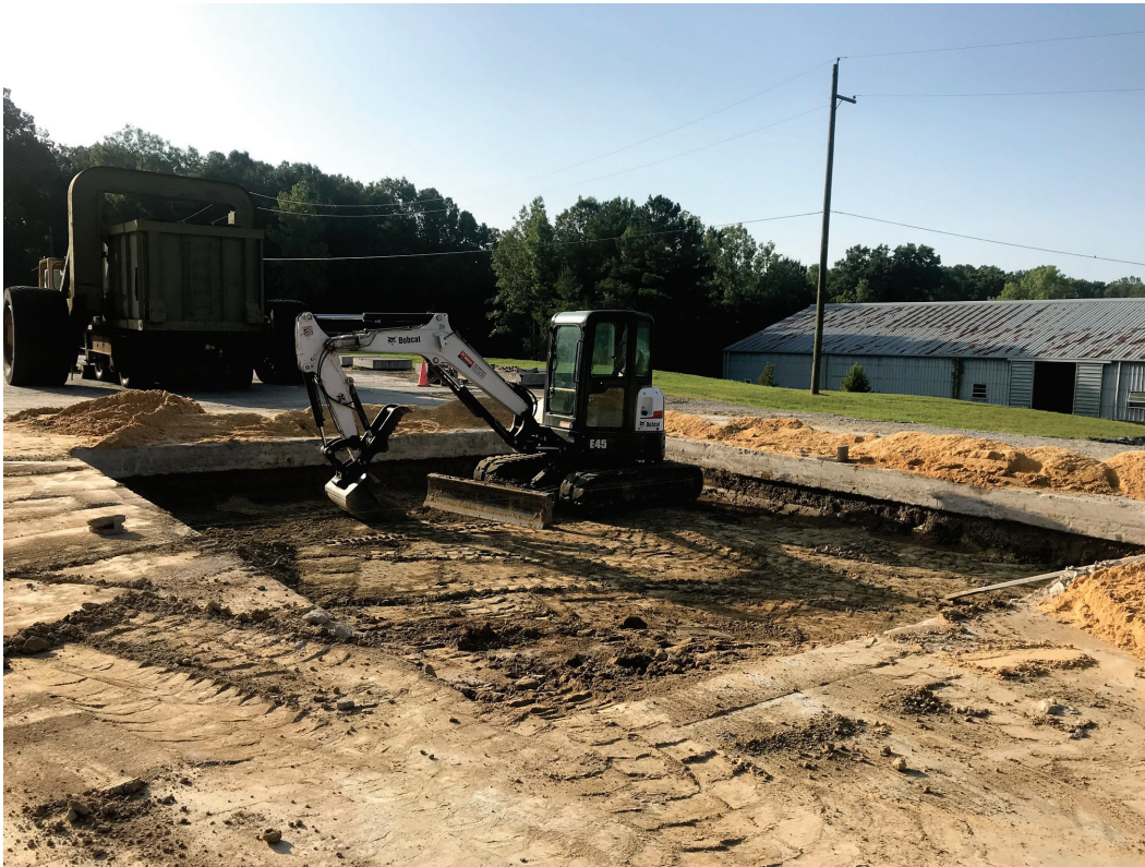
Figure 10. Excavating a repair with a mini excavator.
