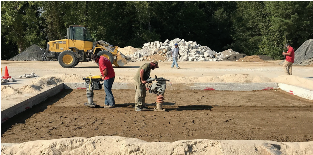
Figure 18. Jumping jack compaction.
