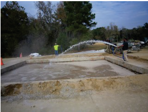
(c) Adding water to dry flowable fill
