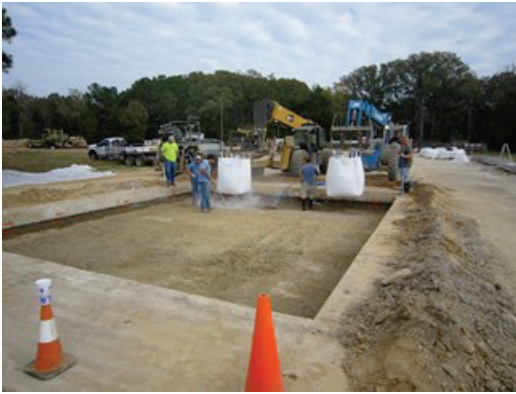
(a) Mobilizing super sacks of flowable fill
