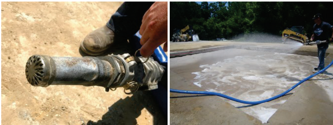
Figure 15. Shower-type nozzle used for dispensing water over dry flowable fill.
