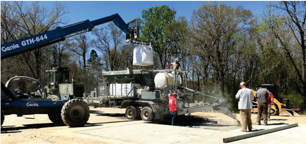
Figure 26. Close-up of placing rapid-setting concrete.
