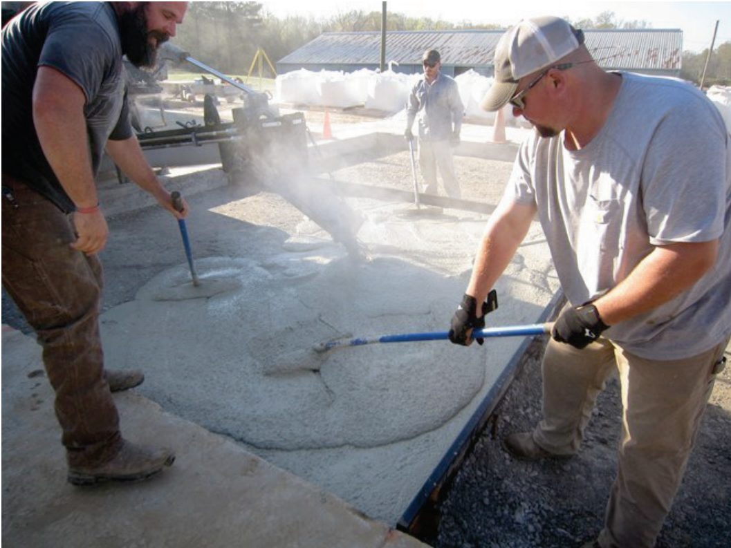
Figure 26. Close-up of placing rapid-setting concrete.
