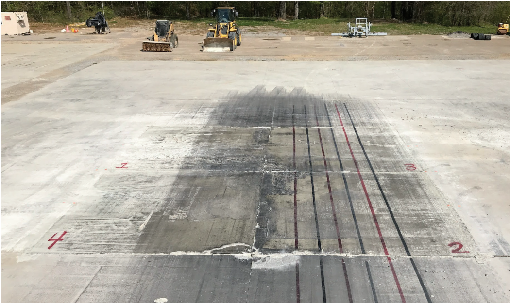
Figure 49. Overview of Repair 5 at 274 passes.
