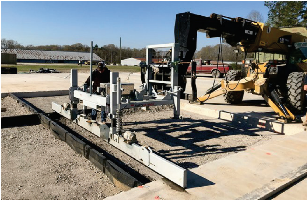
Figure 30. Modified prototype screed, RADR Screed.
