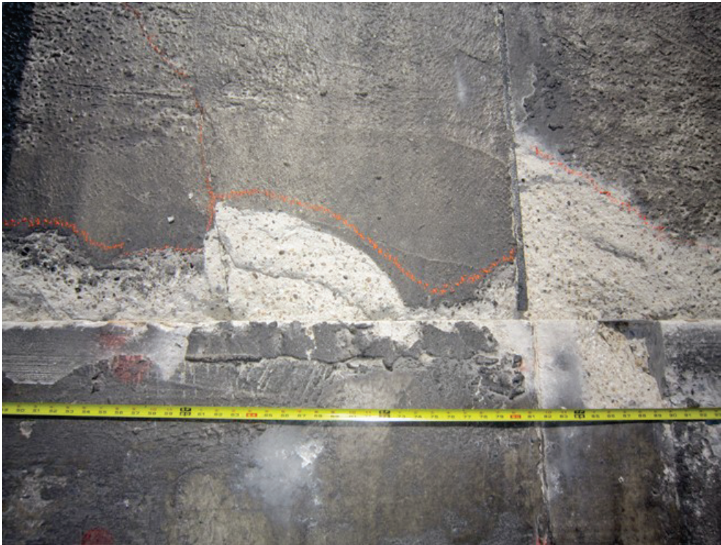
Figure 47. Western edge of Repair 4 after 336 passes.
