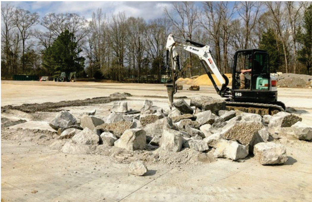
Figure 9. Breaking the PCC surface of the parent slabs.
