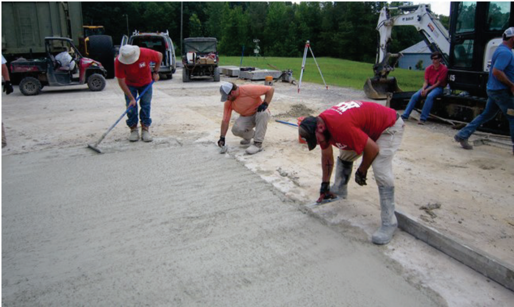
Figure 31. Cleaning excess material from outside of the repair.
