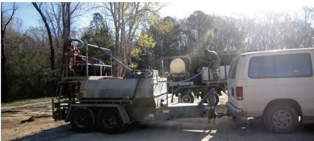
Figure 32. Refilling volumetric mixer water tanks (background).
