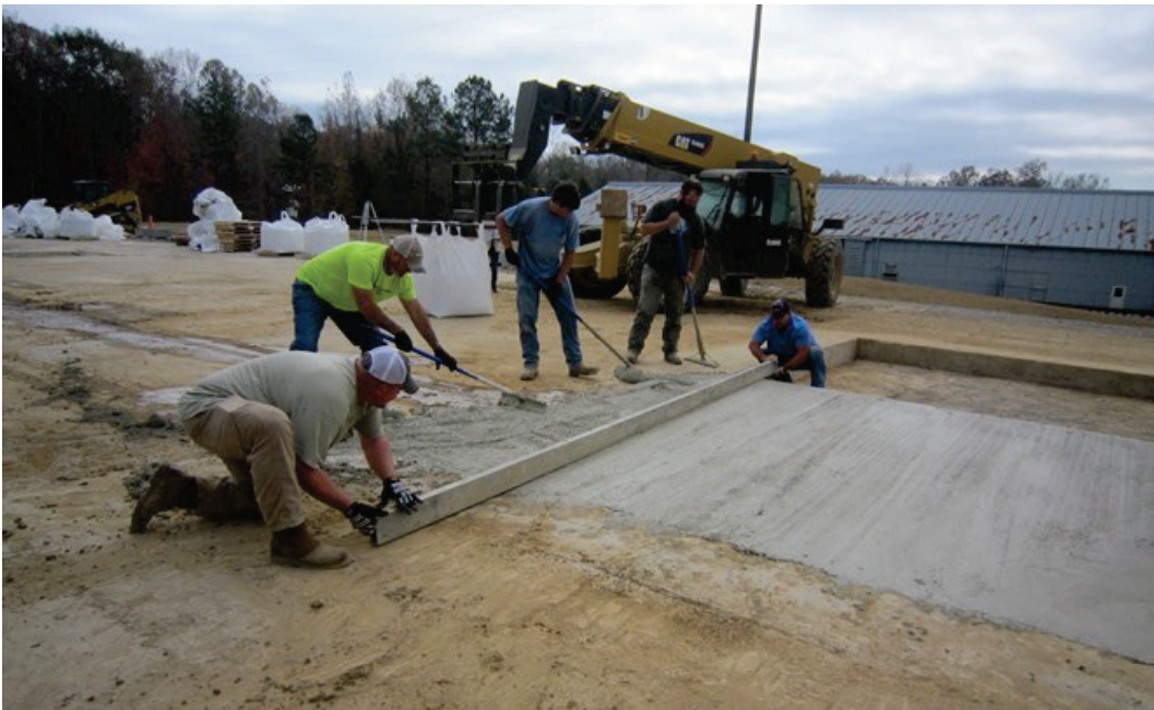
Figure 28. Screeding with 20-ft-long magnesium bar.
