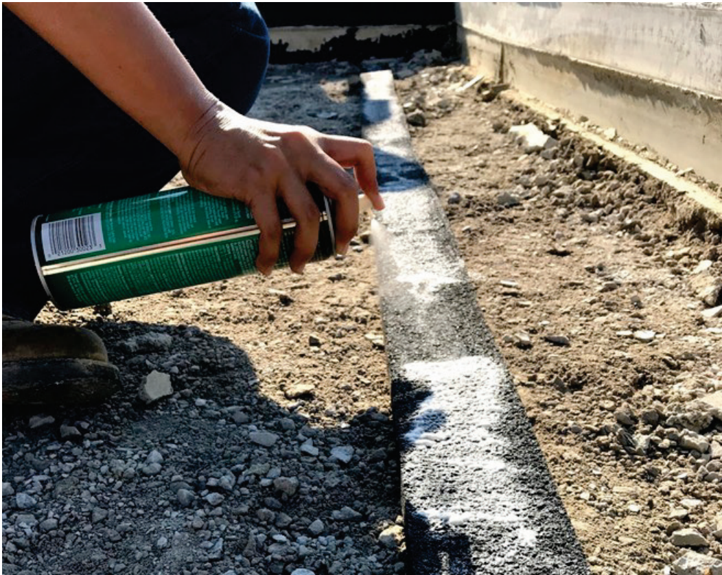
Figure 24. Spray adhesive on expansion board.
