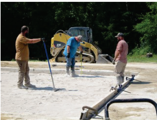
(e) Spot checking flowable fill depth
