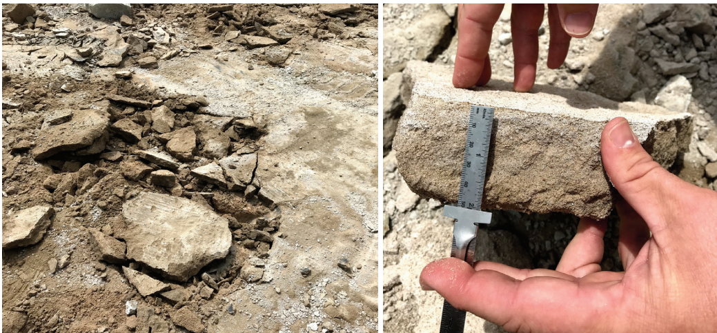
Figure 45. Close-up of flowable fill layers during removal.
