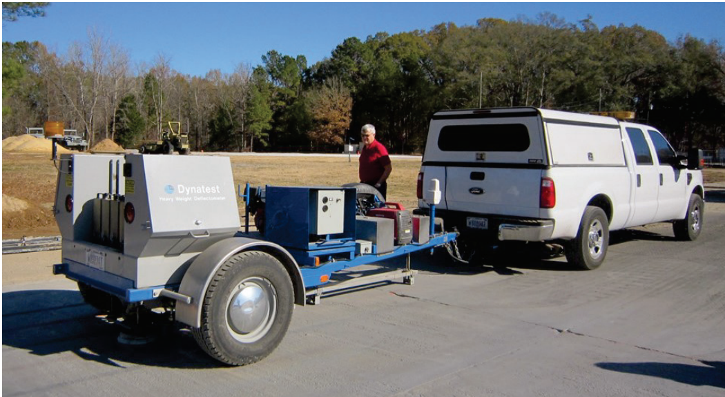
Figure 6. HWD testing on a large crater repair.
